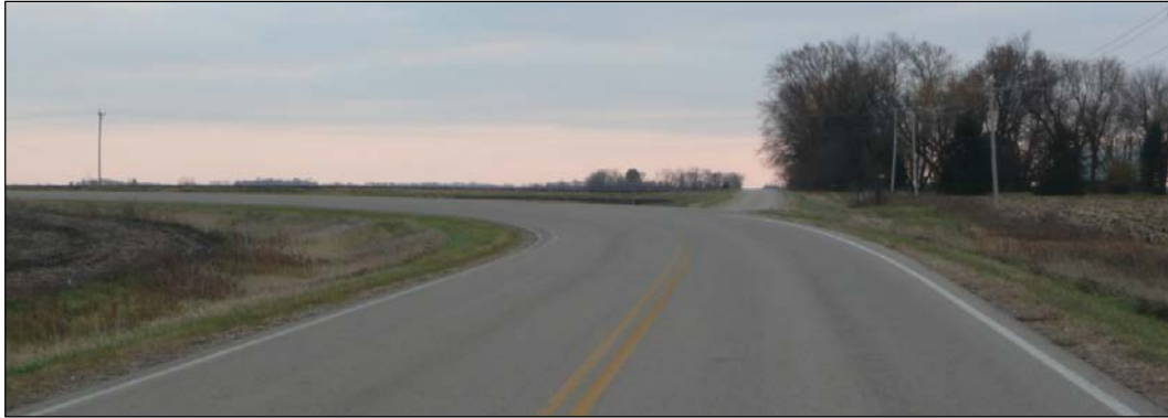
FIGURE 2-9 Example of a Visual Trap – Minor Road Intersects Roadway on a Curve
