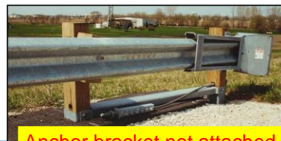
Anchor bracket not attached
