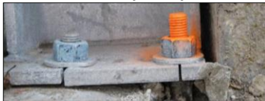
Full bolt depth required
