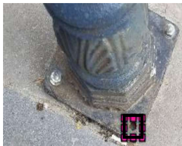
Figure 13: Structure with a missing bolt, shown by bonding box annotation
