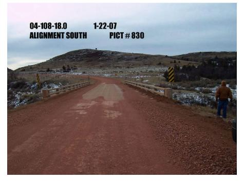
Well graded and maintained, good gravel or paved surface, tracks indicatethat 2 vehicle operation is normal Appendix G: Reinforced Concrete Box Culvert 48 Month Inspection Frequency Criteria
