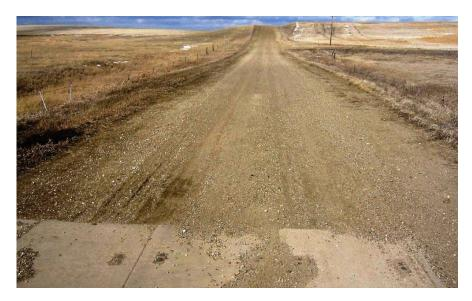
ADT = 20 Two tracks, grade raise apparent, gravelsurface, continual single vehicle use
