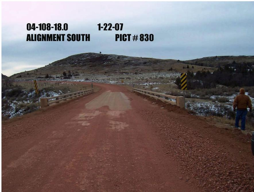
ADT = 50-100 Well graded and maintained, good gravel or paved surface, tracks indicate that 2 vehicle operation is normal
