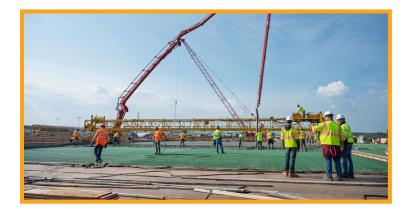
The deck was placed in four separate pours, each requiring a seven-day cure. The final pour is curing and will be complete by mid-July. In total, the bridge will use roughly 500 truckloads of concrete, with the deck itself accounting for 125.
