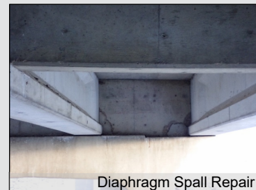
Diaphragm Spall Repair
