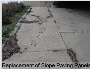
Replacement of Slope Paving Panels
