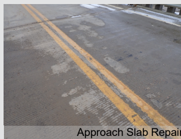
Approach Slab Repair
