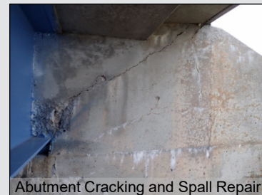
Abutment Cracking and Spall Repair
