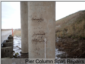
Pier Column Spall Repairs
