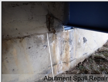
Abutment Spall Repair
