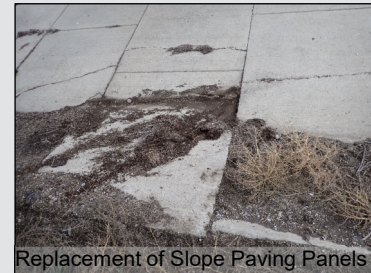
Replacement of Slope Paving Panels
