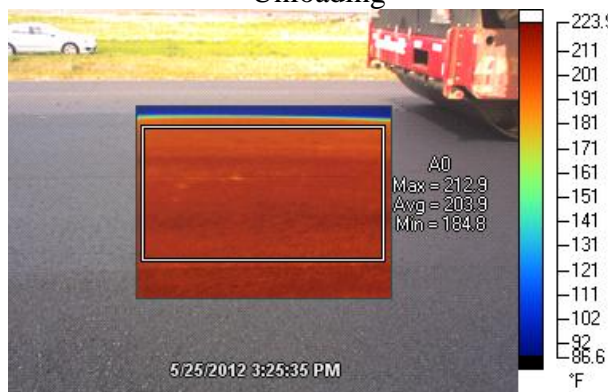
Before Breakdown Roller
