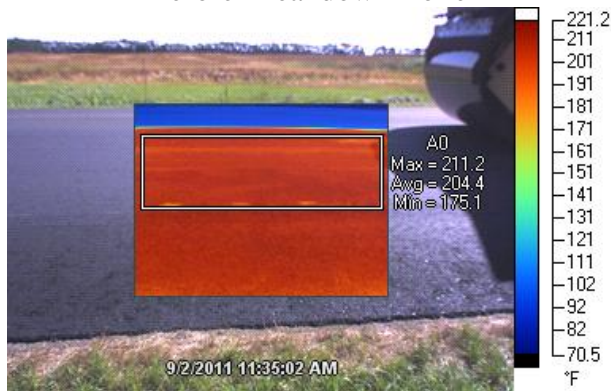
Before Intermediate Roller
