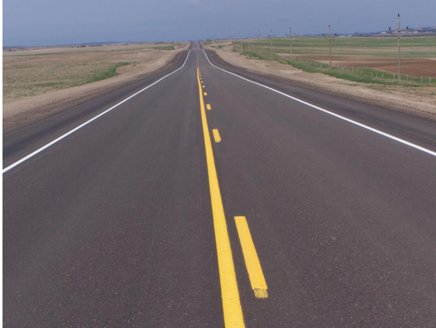
Photo 2 – US 12 after placement of pavement markings and shoulder rumble strips.
