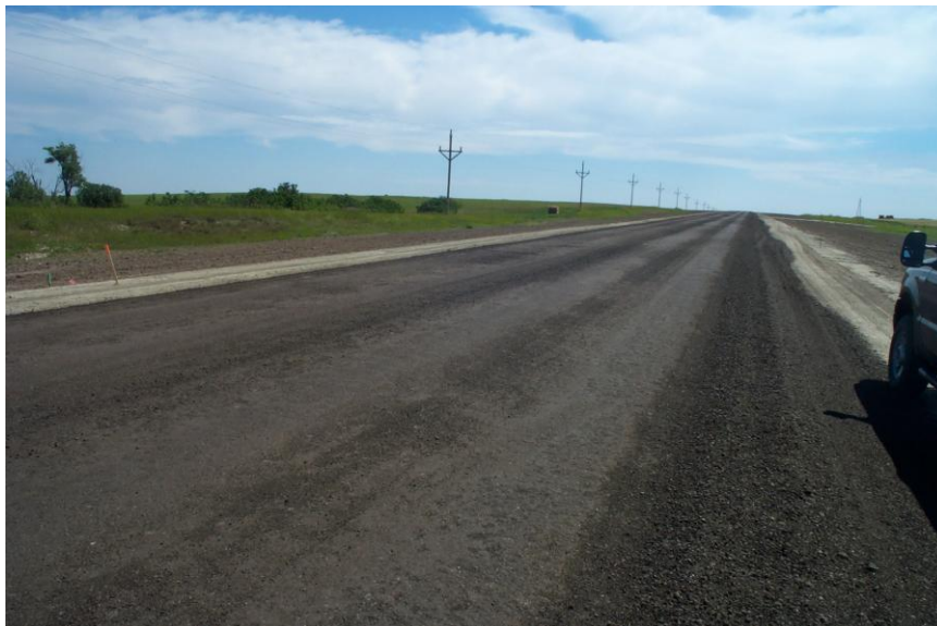
Photo 1 – Test segment with salvaged HBP on top of the pavement.
