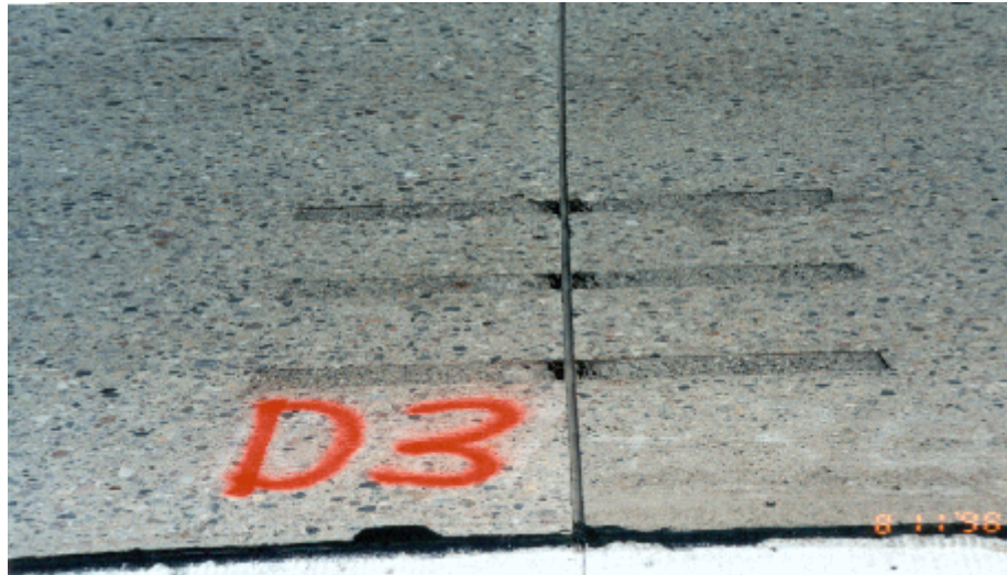
Photo 16. An area that is experiencing mix problems in the dowel bar slots.
