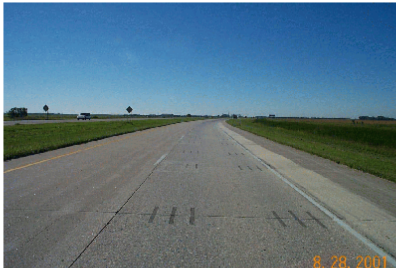
Photo 2. An overall view of the dowel bar retrofit section.
