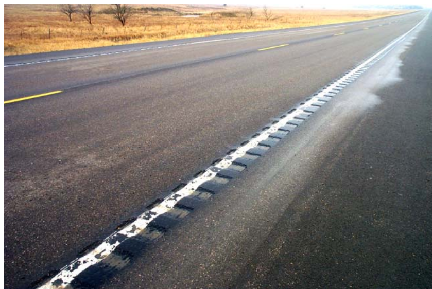
Photo 5 - -An overview of the “rumble stripes”.
