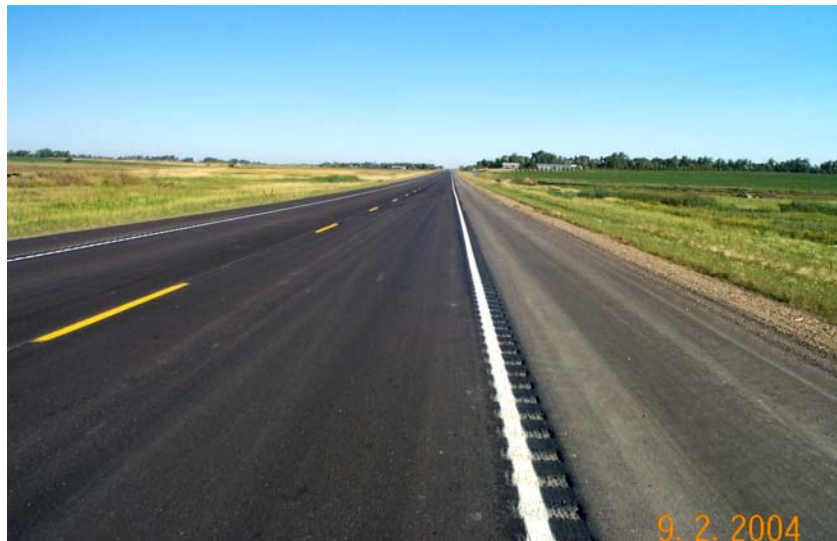
Photo 1 – Completed test section.
