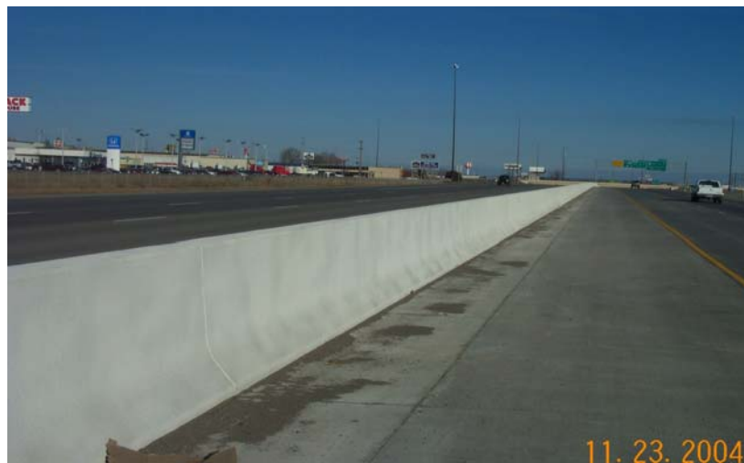
Photo 3 – Cured XL-70C on Jersey barrier.
