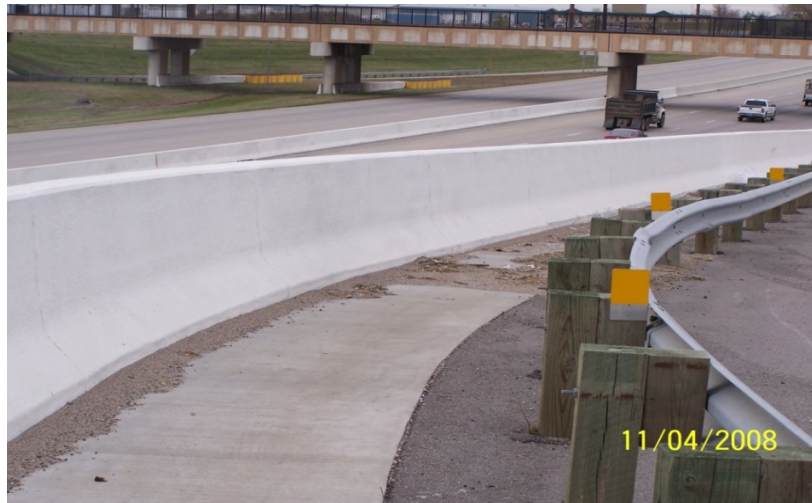
Photo 7 – Control section performing well behind guardrail.
