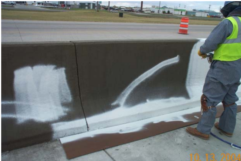
Photo 2 – Contractor’s personnel applying the product.
