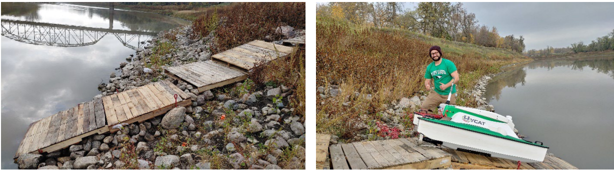
Figure 36. Temporary walkway built for launching HYCAT on a rocky steep slope.
