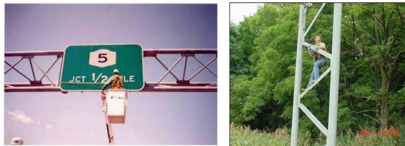
Figure 1: Inspection with (a) Bucket truck and (b) Climbing [2]
