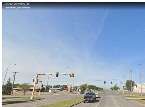
Figure 23: Inspection Location, 3526 Gateway Drive, Grand Forks, ND
