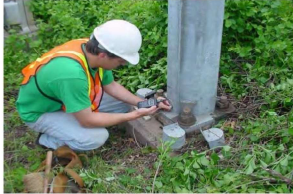
Figure 2: Thickness Measurement at Critical Location of Structure Post [2]
