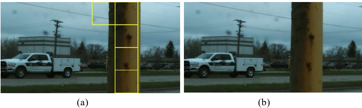
Figure 27: Saved image in repository after completing the inspection (a) Corrosion (b) Crack & defective bolt
