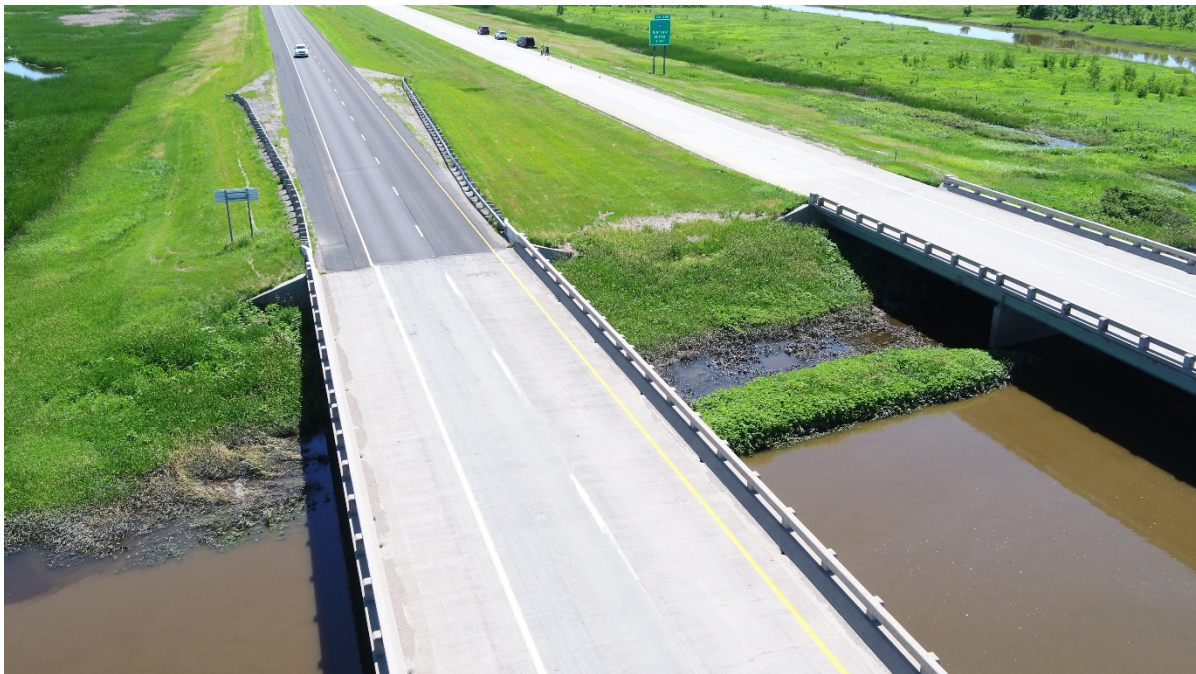
Figure 1. Picture showing a section of the Forest River North & South-Bounds approach and concrete bridge deck captured using a UAS during one of the flight operations in 2020 summer.
