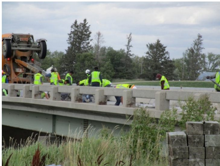
Figure 14. Shows Forest River bridge steel girders and concrete barrier rails.
