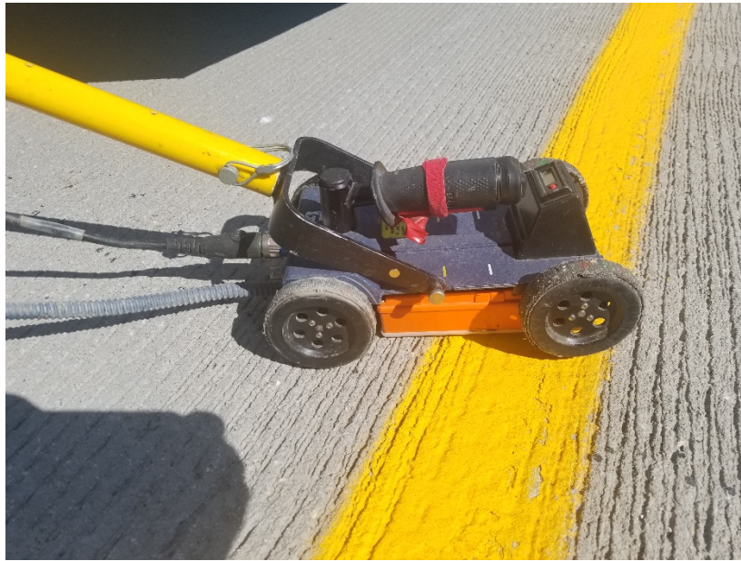
Figure 3. Data Collection on a Bridge Deck Using Ground-Coupled GPR
