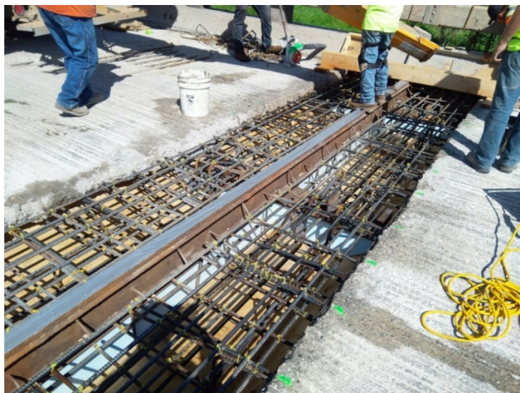
Figure 15. Crew preparing Park river bridge expansion joint for repair.
