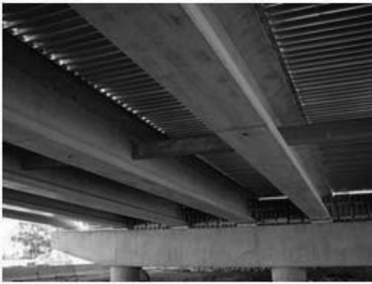
Figure 4: SCC girders support the PRB [13]
