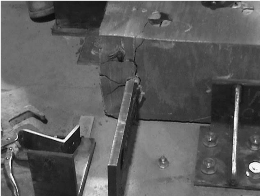
Figure 48: Typical pullout failure.
