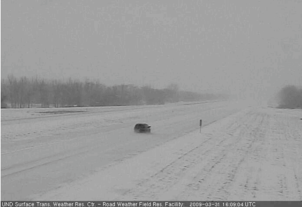
Figure 17 Interstate 29 pavement conditions at 16:09 UTC on March 31, 2009. Snow covered conditions on the road would warrant slower driving conditions as indicated in Table 11 above.
