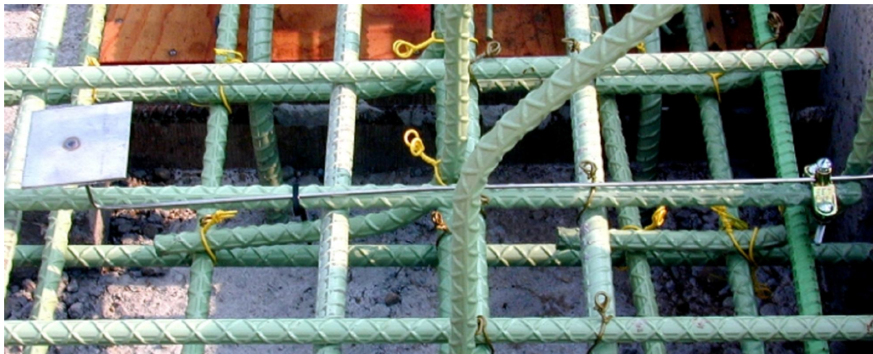
Figure 1: Stainless Steel Contact Attached to Bridge Deck Rebar
