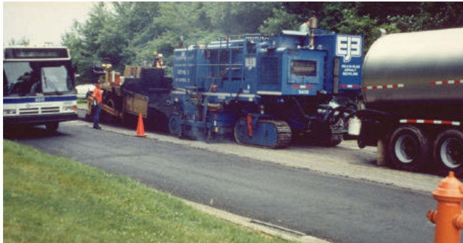
Figure 4.6. The recycling train used on the job (Baltimore County).
