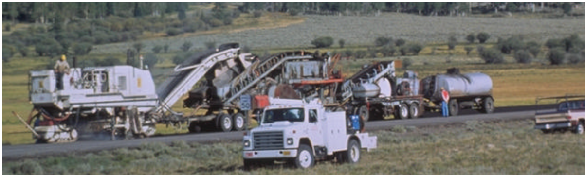
Figure 3.10. An overview of the recycling units of a multi-unit train.
