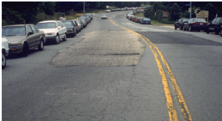
Figure 4.5. Existing road (Baltimore County).
