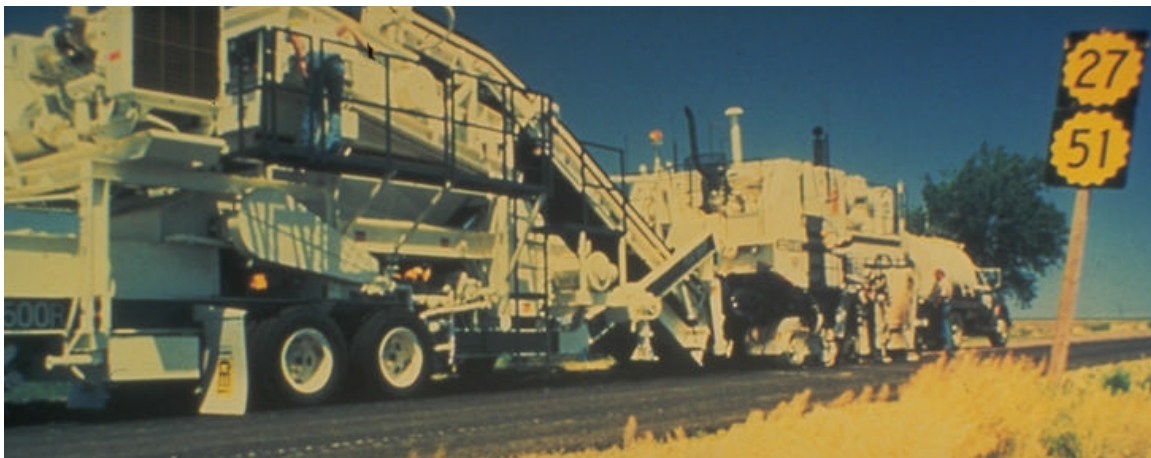
Figure 3.6. Portable crusher attached to cold-milling machine.
