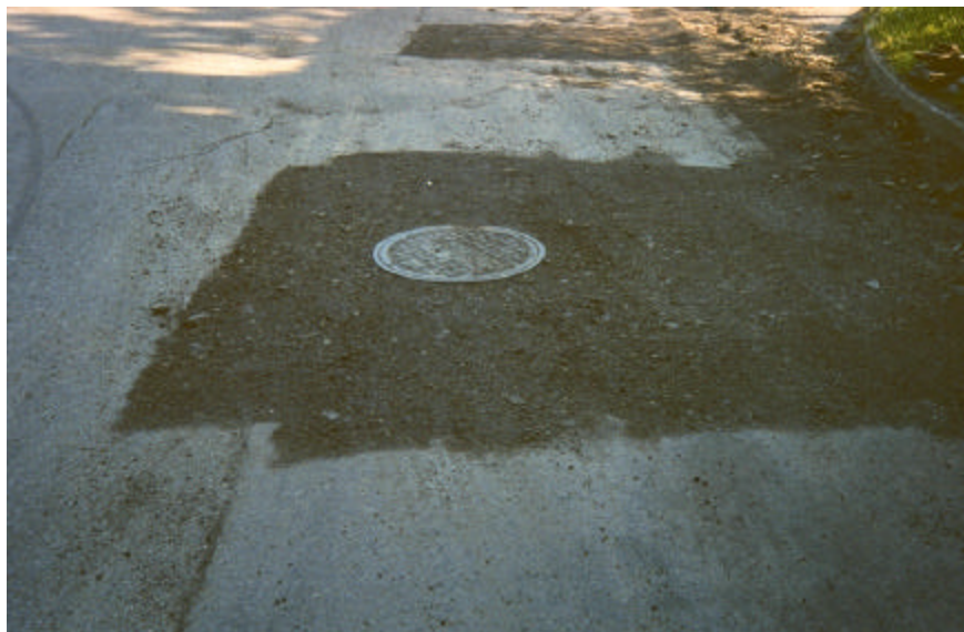
Figure 4.10. Recycled material around utility.
