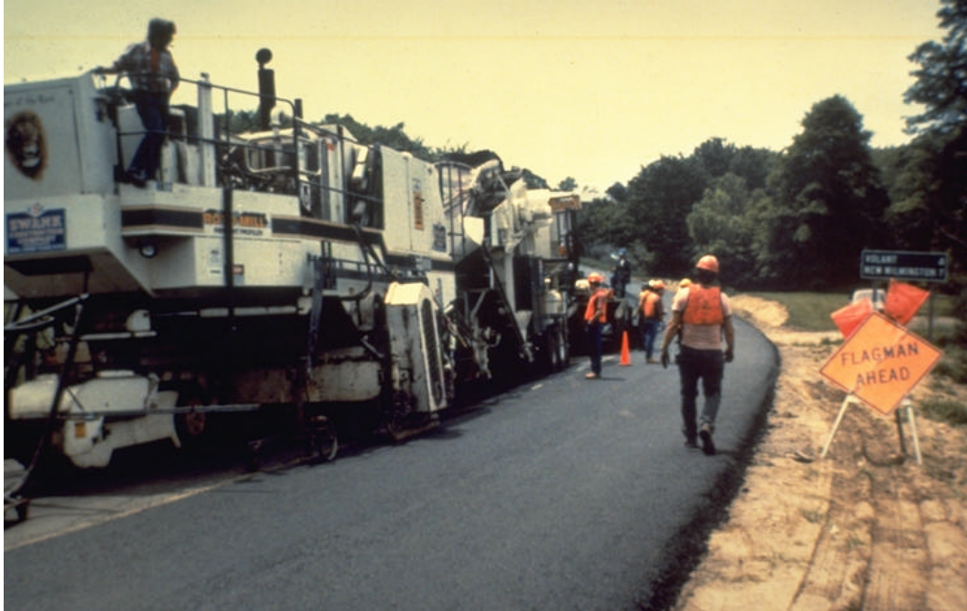
Figure 4.1. Recycling train used on the Mercer County project.
