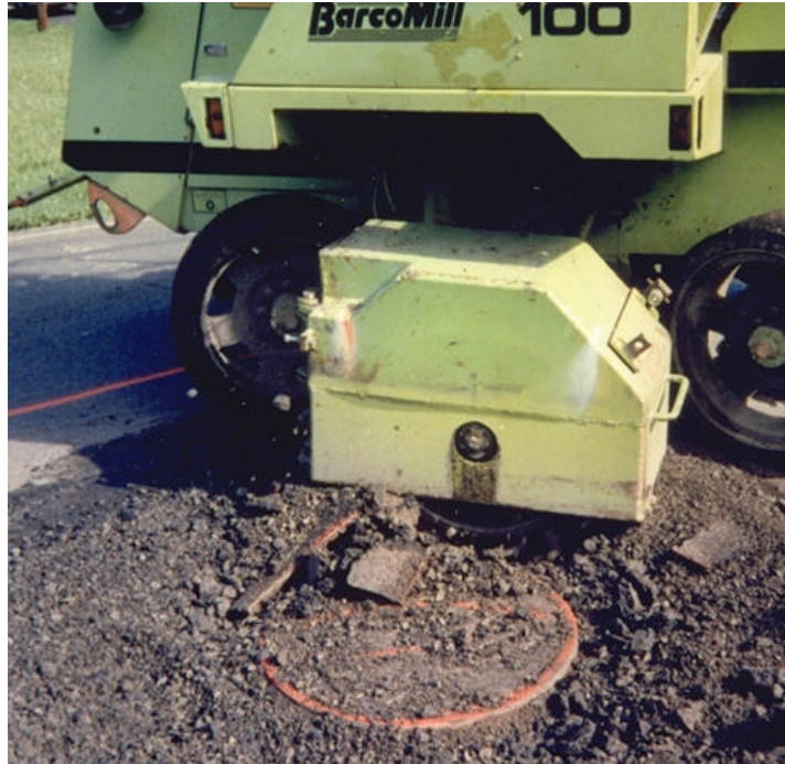
Figure 4.9. Milling around utility.
