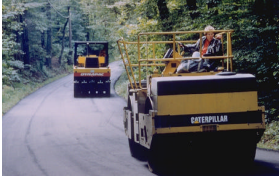
Figure 4.7. Rollers used for compaction.
