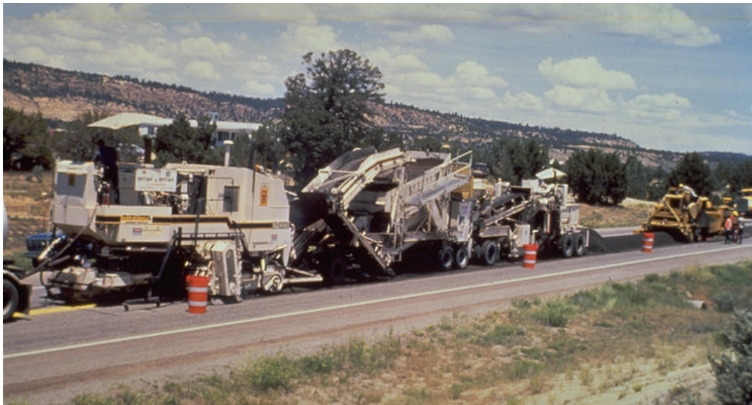
Figure 4.3. Recycling train used on the US 64 project.
