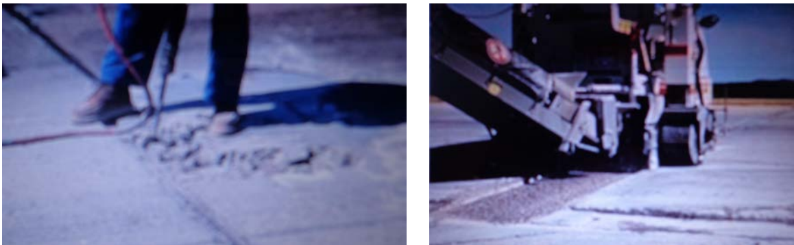
Fig. 3. Concrete removal for patching using jackhammer (left) and milling machine (right).
