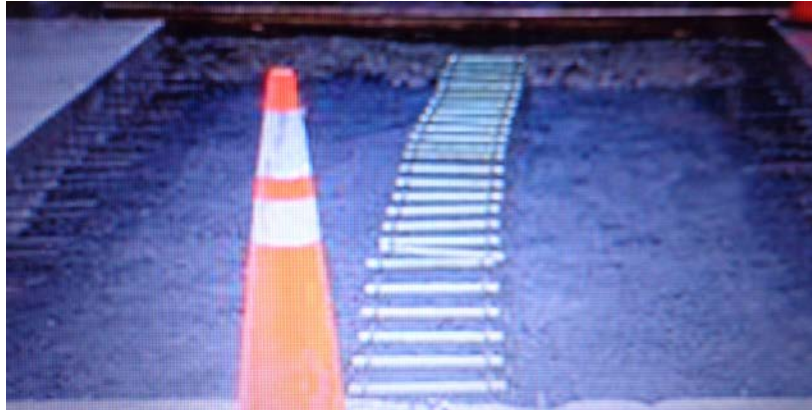
Fig. 2. Installation of tie bars and dowels for load transfer
