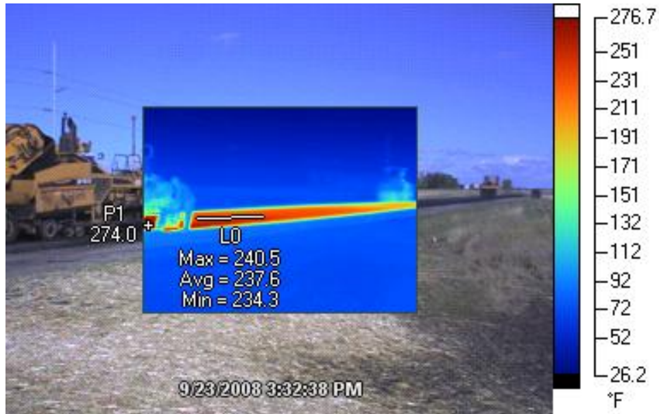
Figure 2. Mainline paving on Highway 5 (ambient temperature 64°F)
