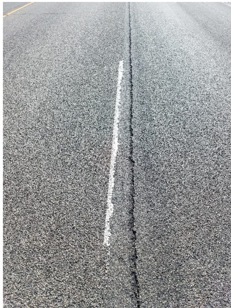
Photo 7 & 8 – Damaged markings at RP 168.0 (Potters Visibead)
