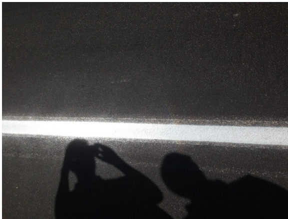
Photo 1 – Epoxy Centerline with 3M All-Weather Elements
