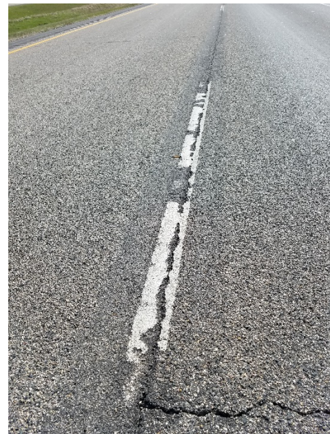
Photo 11 & 12 – Damaged markings at RP 180.0 (3M AW Elements)
