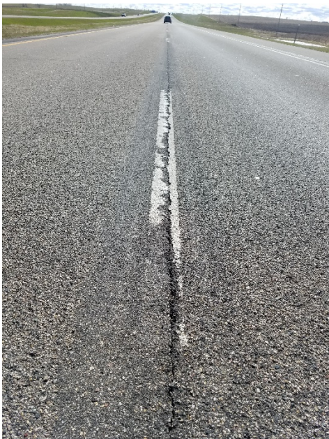
Photo 11 & 12 – Damaged markings at RP 180.0 (3M AW Elements)
