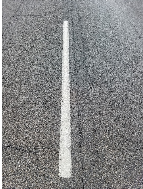
Photo 5 & 6 – Good condition markings at RP 169.0; Typical condition of pavement marking along project corridor (Potters Visibead)
