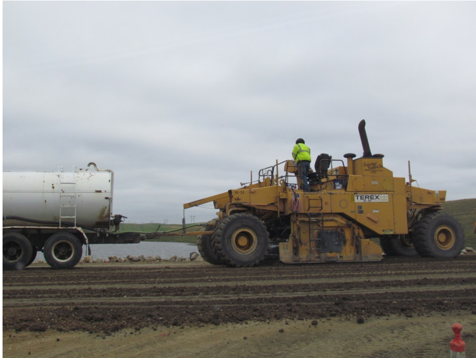
Photo 1: Application of diluted Permazyme 11x on EB ND 53, RP 30
