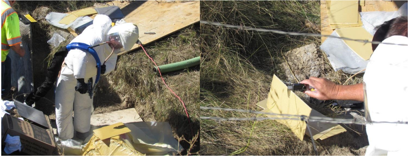
Photo 9 – Spraywall test panel and thickness measurement.
