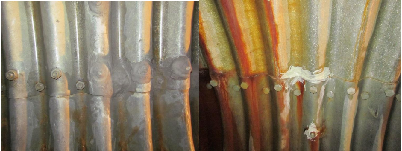
Photo 13 – Quick set mortar and SR 6100 smoothing out sharp angles.
