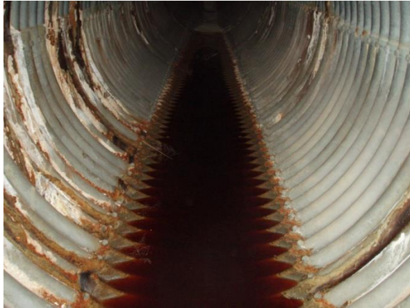
Photo - Deterioration of 90" Structural Steel pipe
