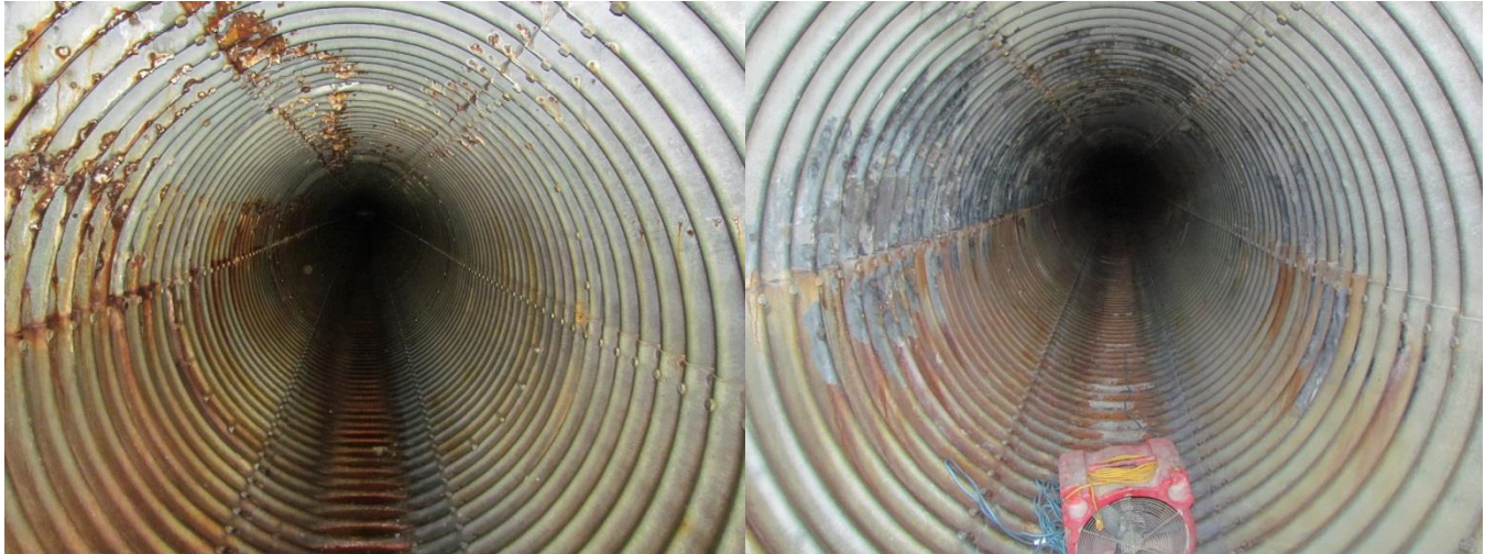
Photo 5 – Before and after pipe preparation
