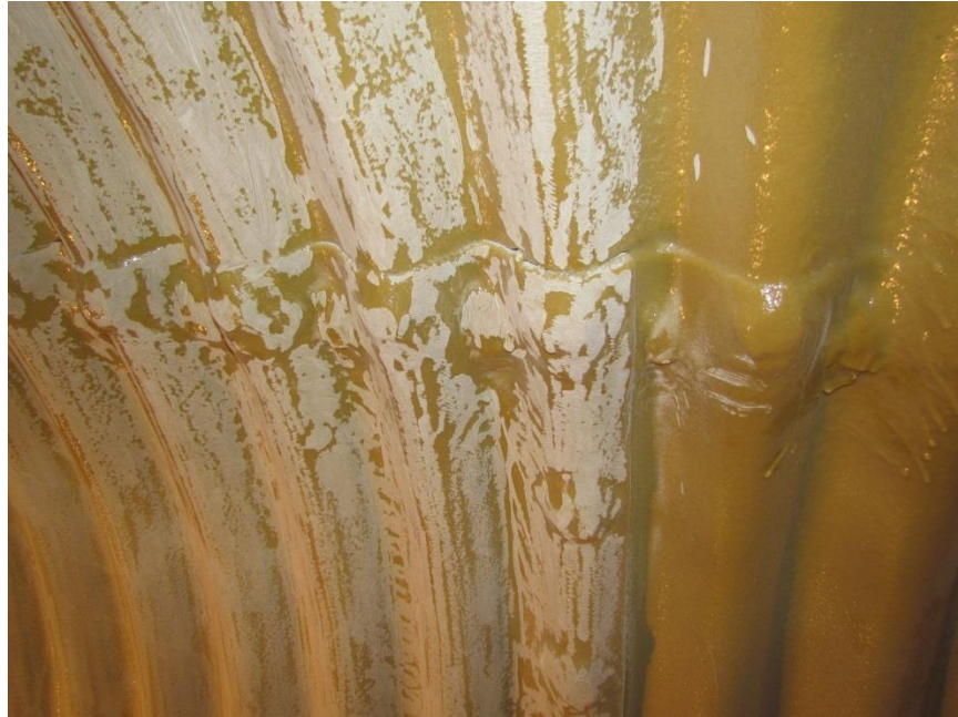
Photo 11 – Spraywall Liner scuffed for overlap preparation.
