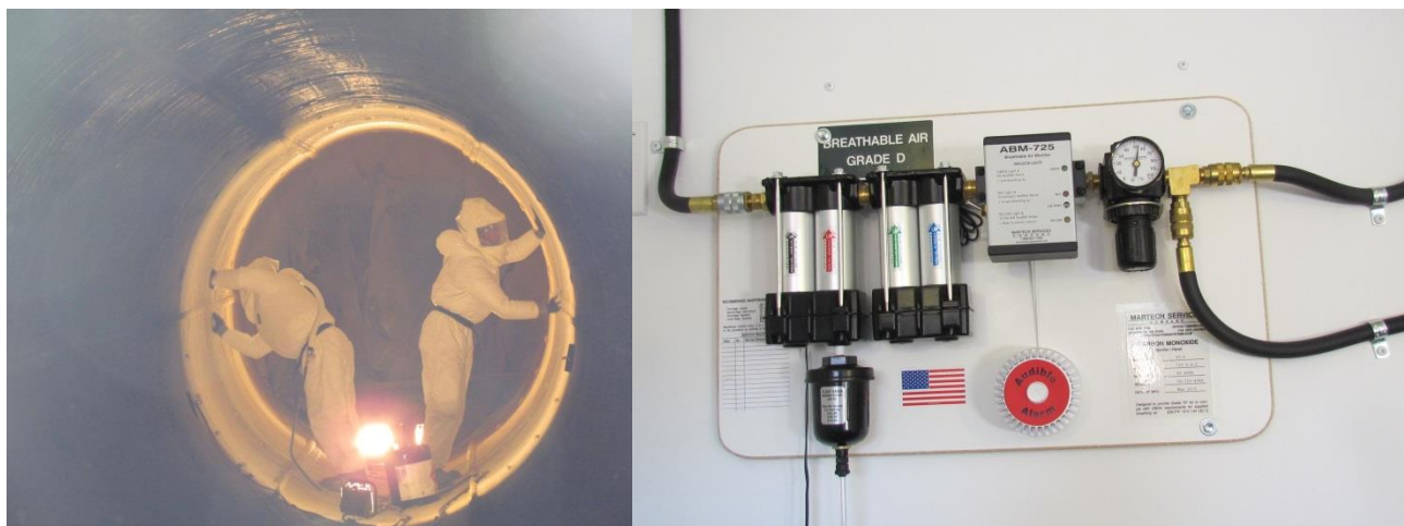
Photo 8 – Full body suit and breathable air regulator.
