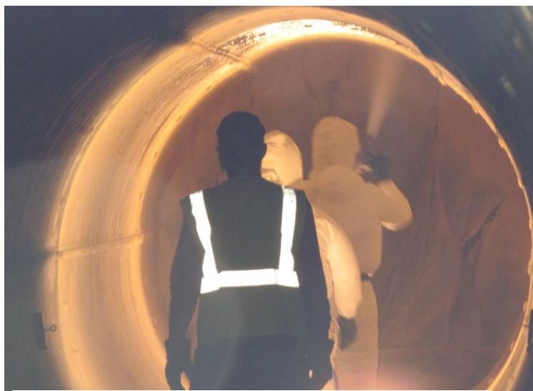
Photo 10 – Application of Spraywall.
