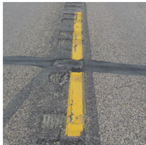
Photo 2 – General Condition of Segment 1
