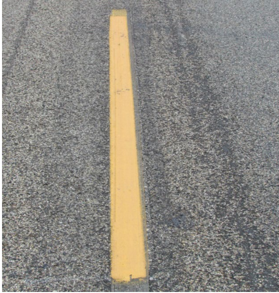
Photo 5 – Segment 3 – Epoxy Marking Intact
