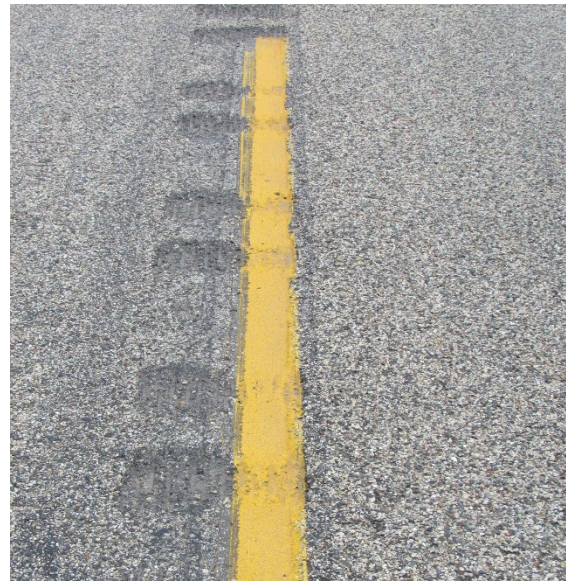
Photo 4 – General Condition of Segment 2
