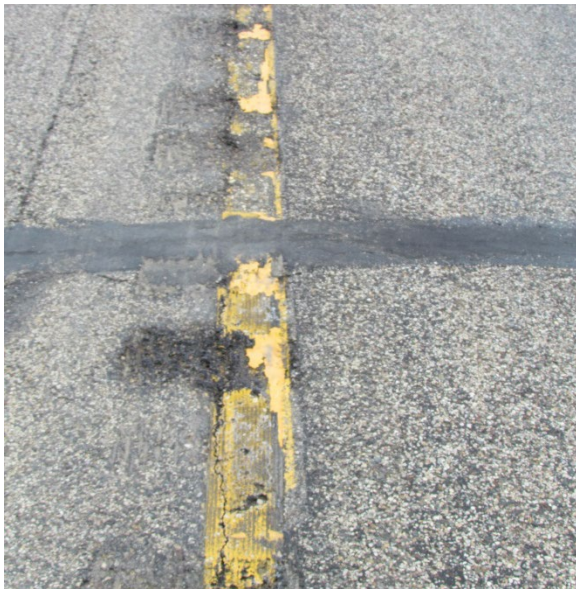
Photo 7 – Segment 3 Delamination
