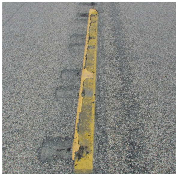
Photo 6 – Segment 4 Delamination
