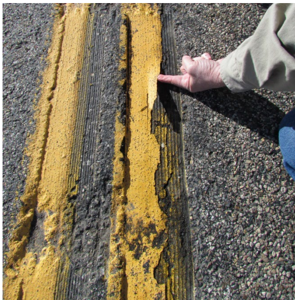
Photo 8 – Segment 4 – Delamination
