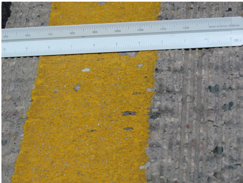
Segment 1B - NB Yellow Grooved Paint with 3M AW Elements – RP 139
