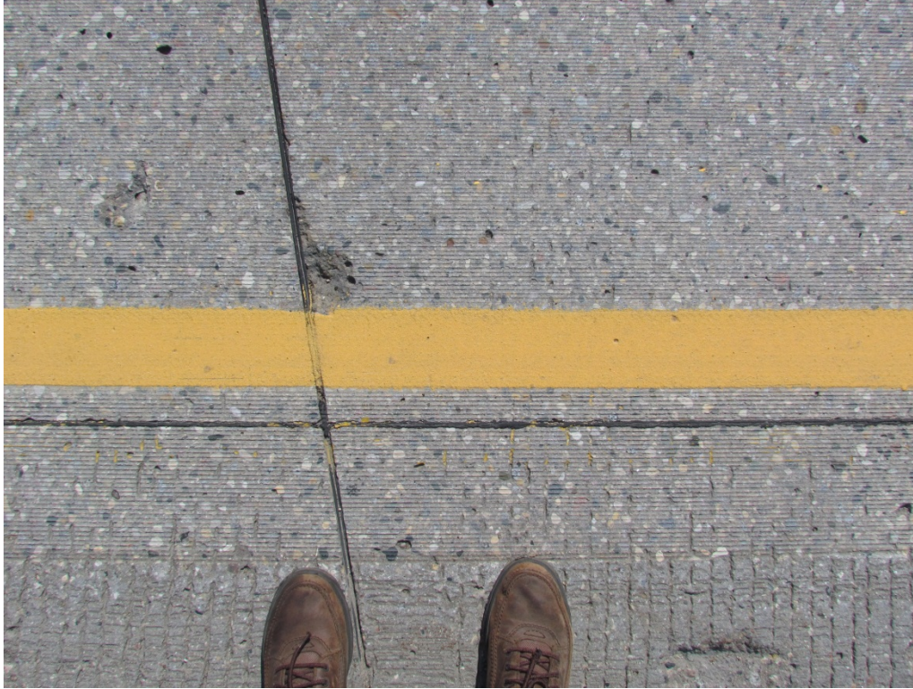
Segment 2A - NB Yellow Grooved Epoxy with Standard Glass Beads – RP 141
