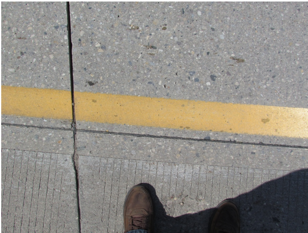
Segment 3B - SB Yellow Surface applied Epoxy with 3M AW Elements – RP 147
