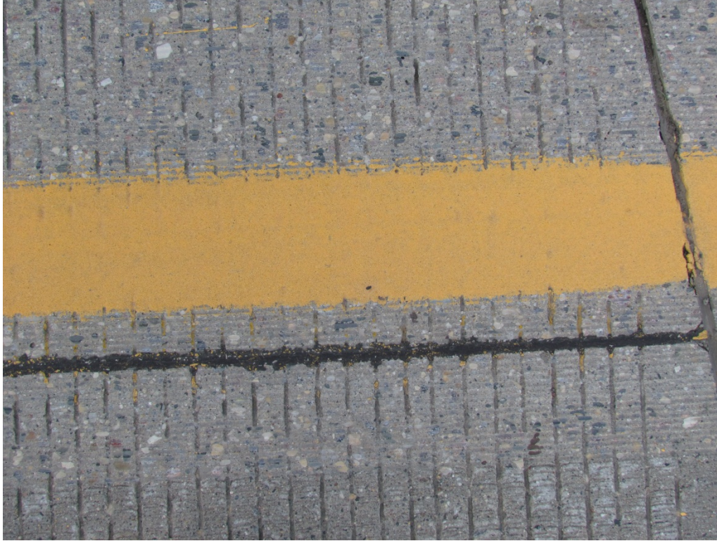
Segment 2A - SB Yellow Grooved Epoxy with Standard Glass Beads – RP 141
