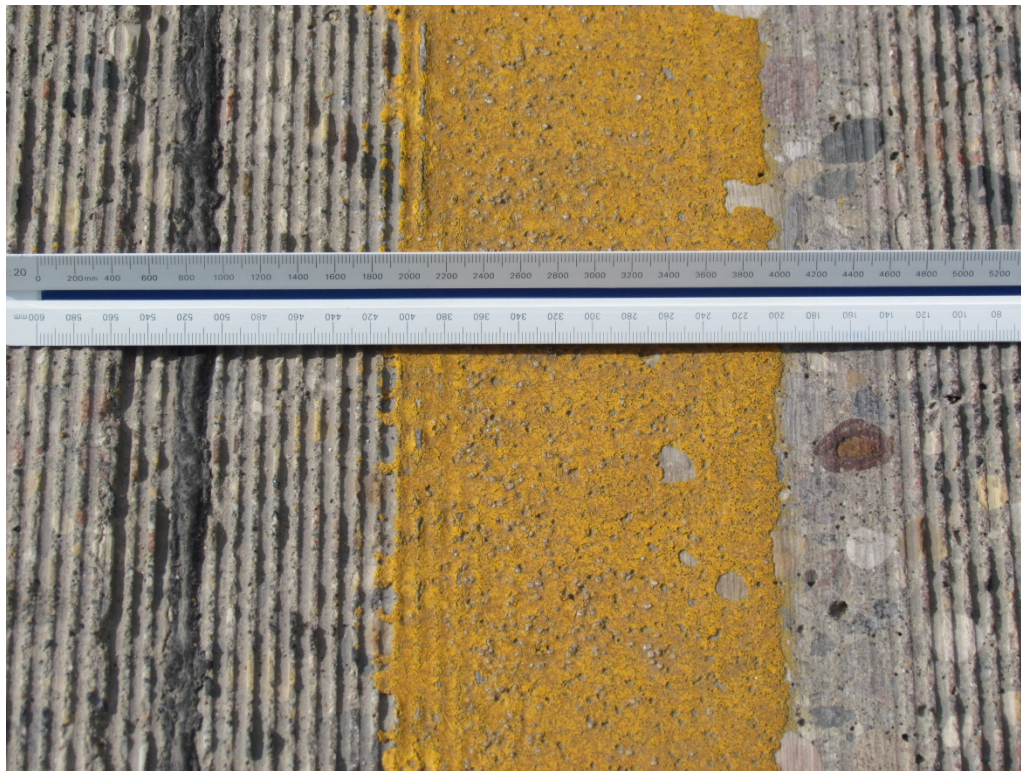
Segment 1B - SB Yellow Grooved Paint with 3M AW Elements – RP 139
