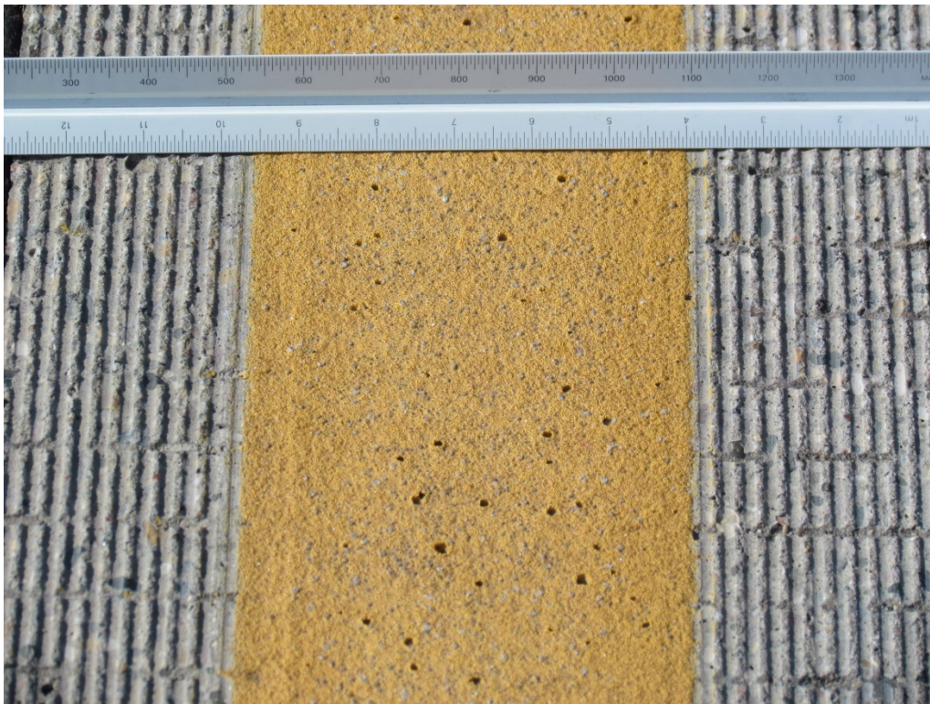
Segment 2B - SB Yellow Grooved Epoxy with 3M AW Elements – RP 143
