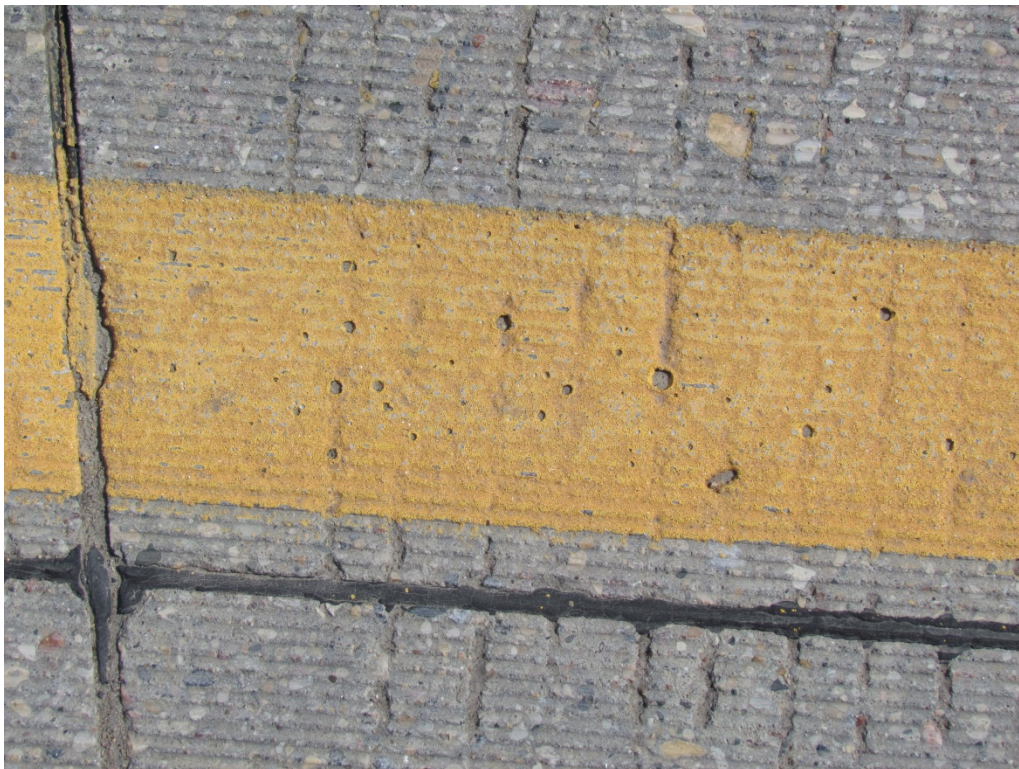
Segment 3B - NB Yellow Surface applied Epoxy with 3M AW Elements – RP 147
