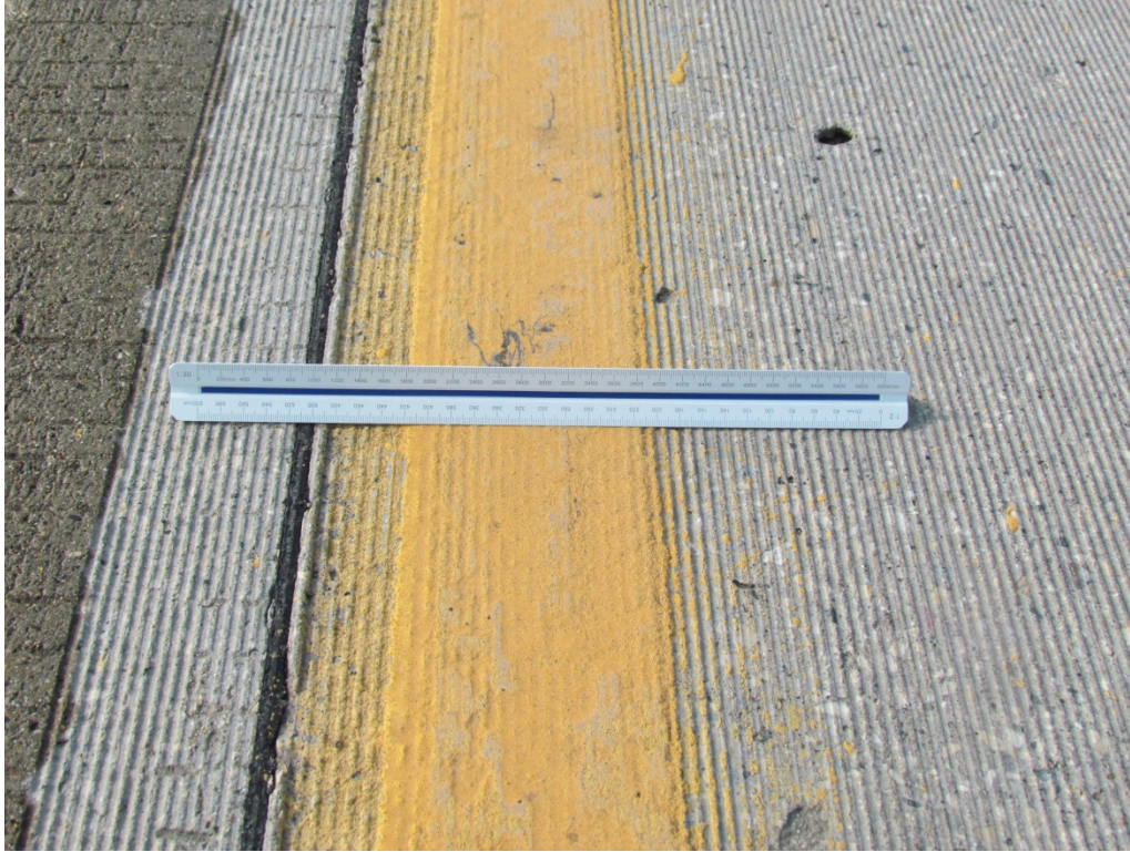
Segment 3A - SB Yellow Surface applied Epoxy with Standard Glass Beads – RP 145
