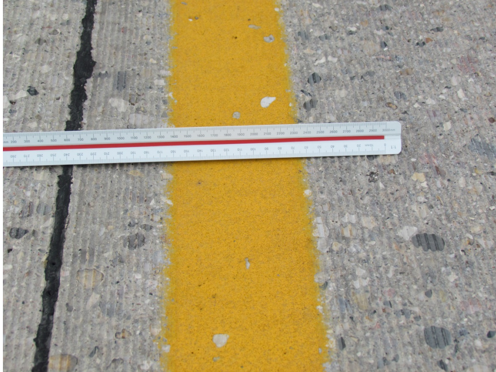
Segment 1A - SB Yellow Grooved Paint with Standard Glass Beads – RP 137
