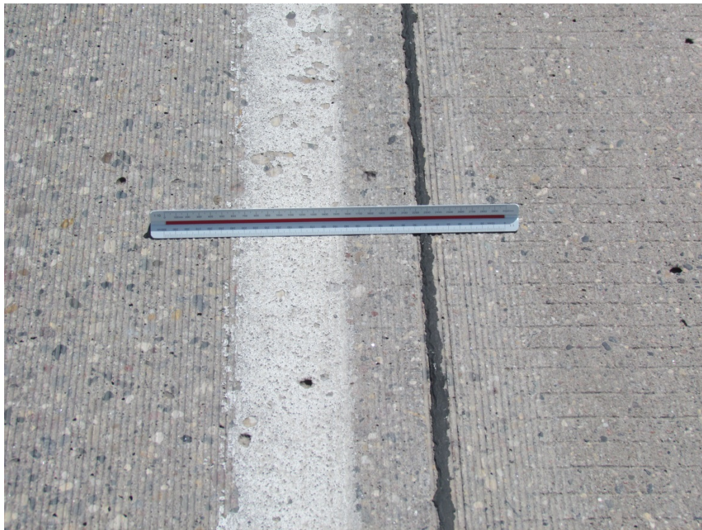
Segment 1B - SB White Grooved Paint with 3M AW Elements – RP 139
