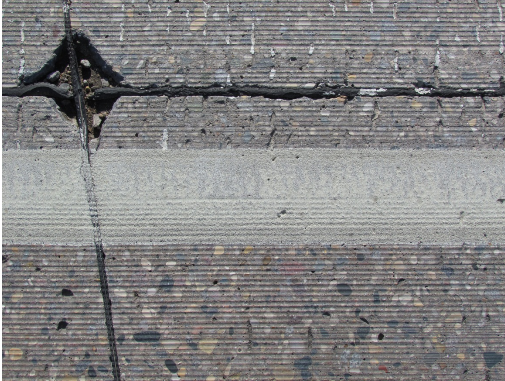
Segment 2A - NB White Grooved Epoxy with Standard Glass Beads – RP 141
