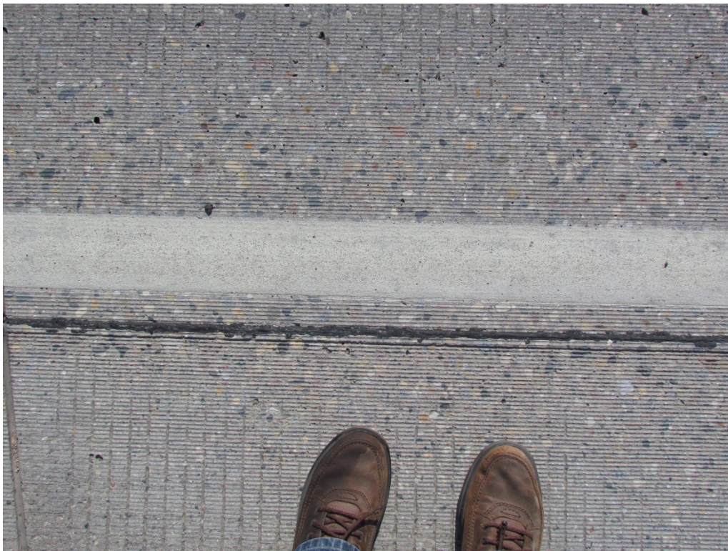
Segment 2B - SB White Grooved Epoxy with 3M AW Elements – RP 143
