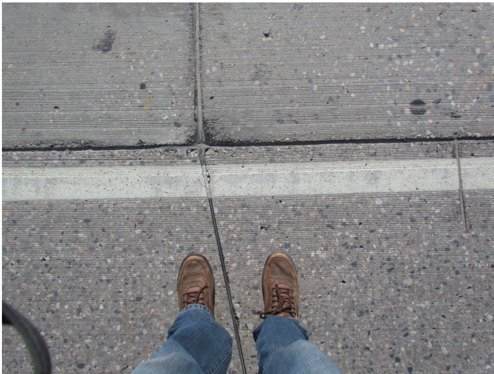
Segment 2B - NB White Grooved Epoxy with 3M AW Elements – RP 143
