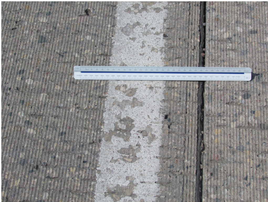
Segment 1B - NB White Grooved Paint with 3M AW Elements – RP 139
