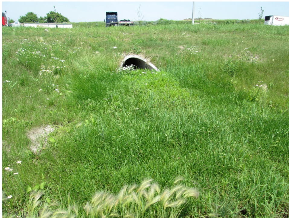
Photo 20: 2nd Evaluation Installation at - Sta. 50+36 Rt. (07/9/2015).
