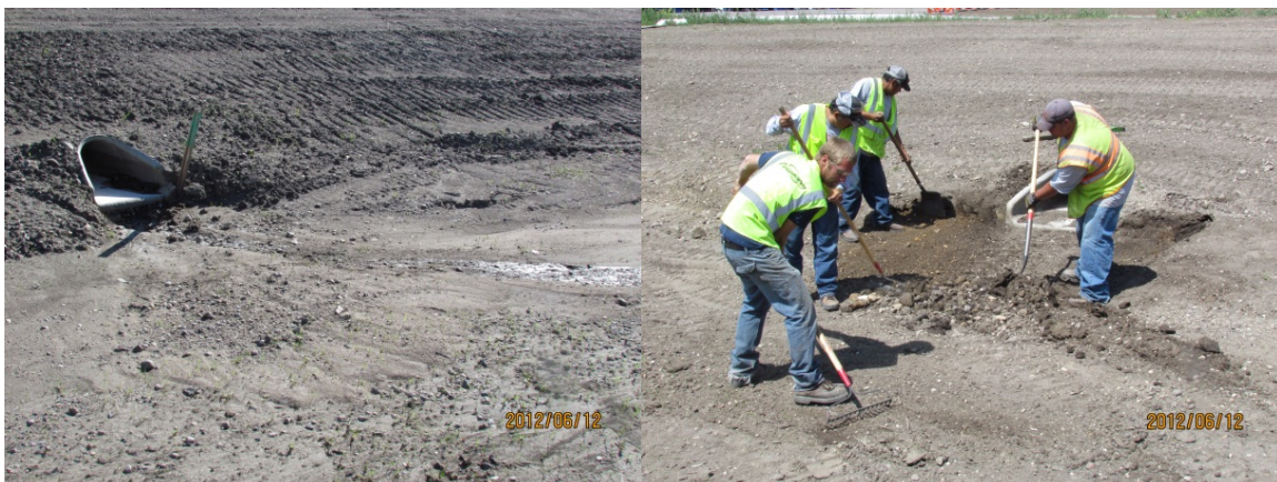
Photo 1: Crew performing grade prep prior to install.
