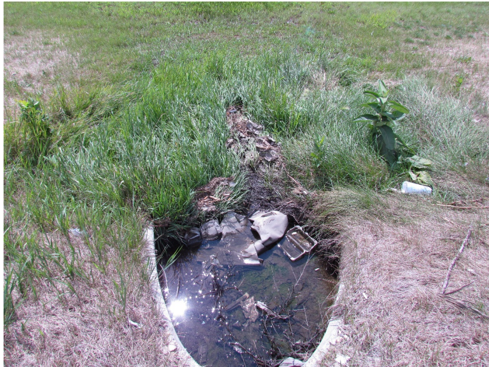
Photo 31: ScourStop® STA 47+90 Rt. Installation (August 9, 2017).
