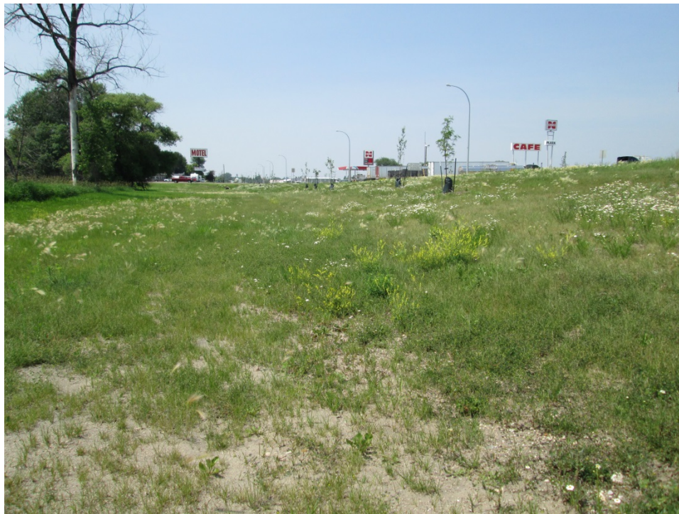
Photo 28: ScourStop® installations (July 9, 2015.)
