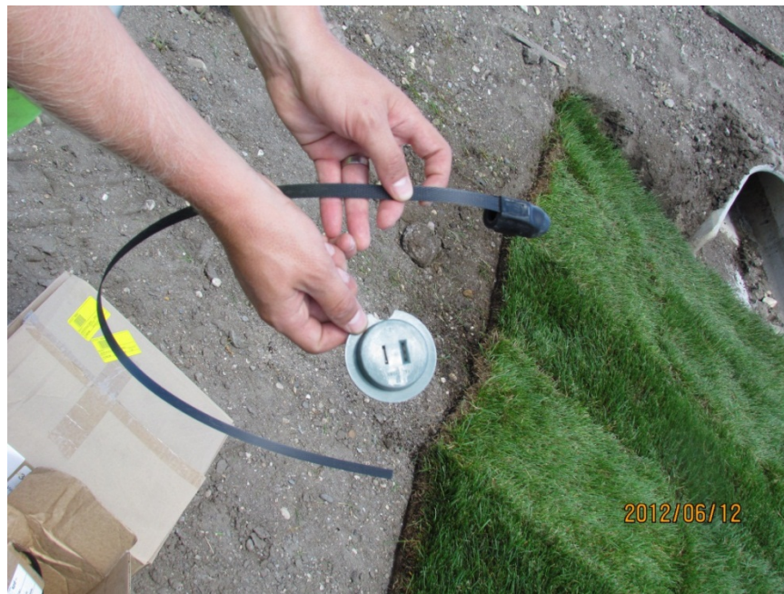
Photo 4: ScourStop® bullet anchor.
