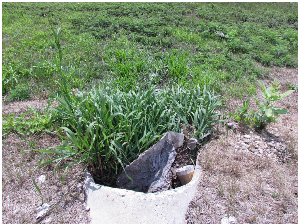
Photo 32: ScourStop® Sta. 50+36 Rt. Installation (August 9, 2017).
