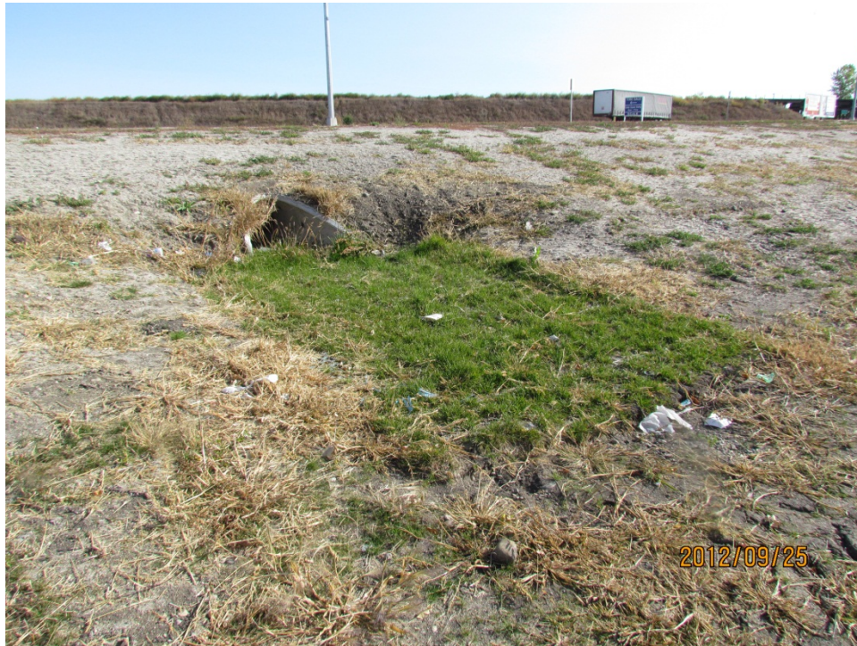
Photo 10: Installation at – Sta. 50+36 Rt. (9/25/2012)
