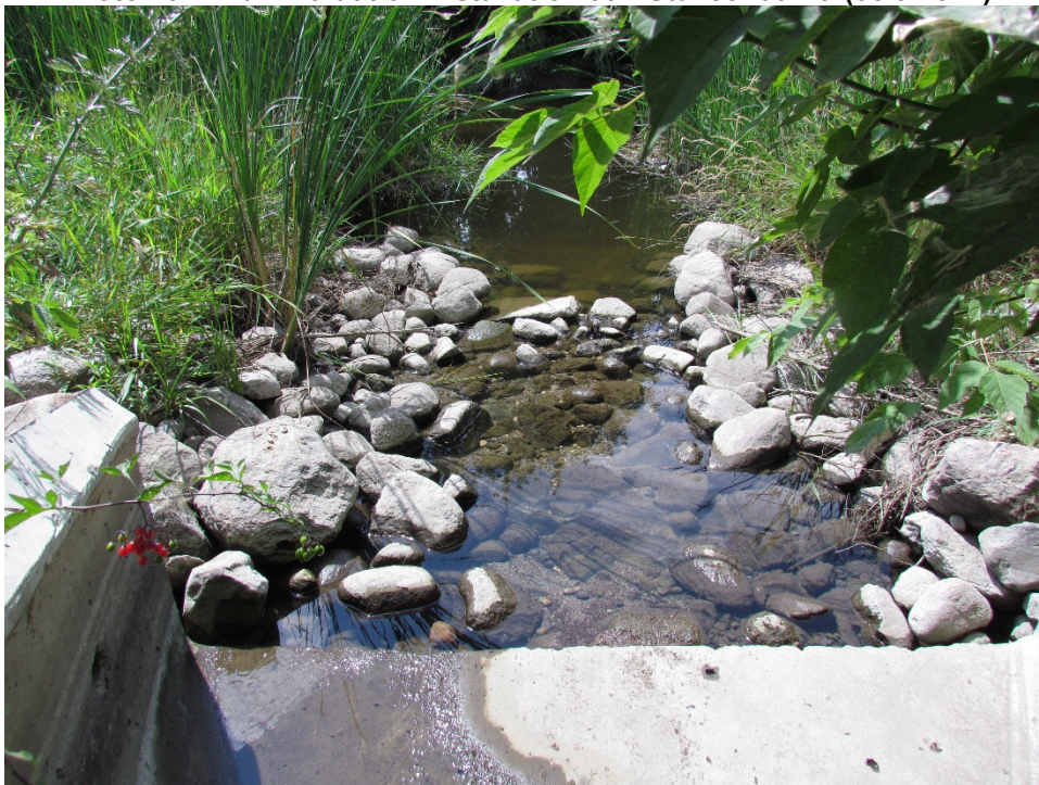
Photo 27: Final Evaluation Control Installation Sta. 24+36 Rt. to Sta. 24+57 Rt. (8/9/17)
