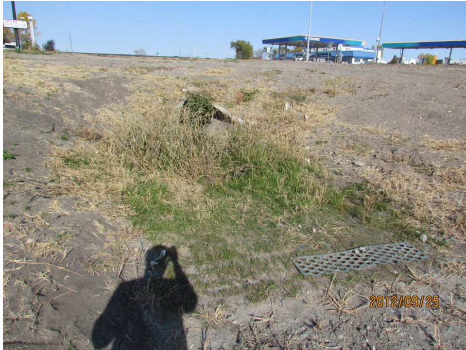
Photo 6: Installation at - Sta. 47+90 Rt. (09/25/2012)
