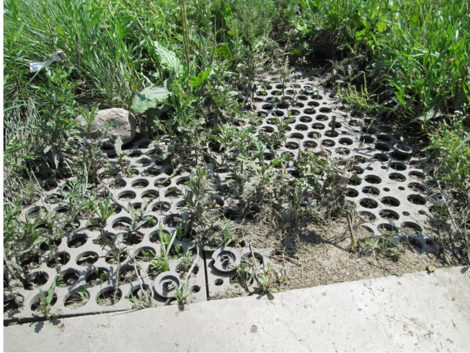
Photo 29: ScourStop® STA 47+90 Rt. Installation (July 9, 2015.)
