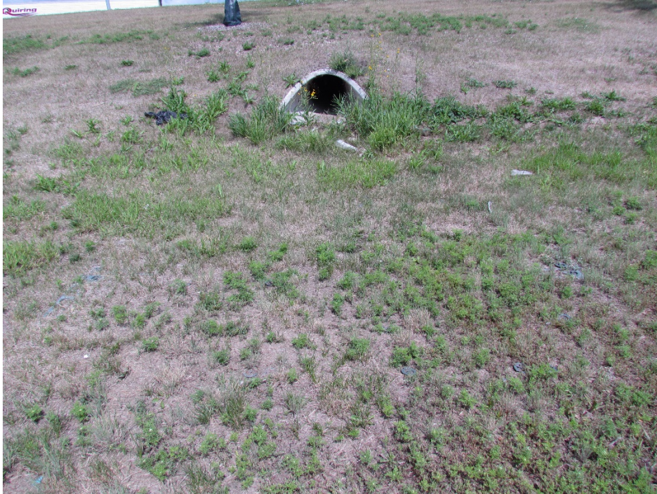
Photo 26: Final Evaluation Installation at – Sta. 53+00 Rt. (08/9/2017)
