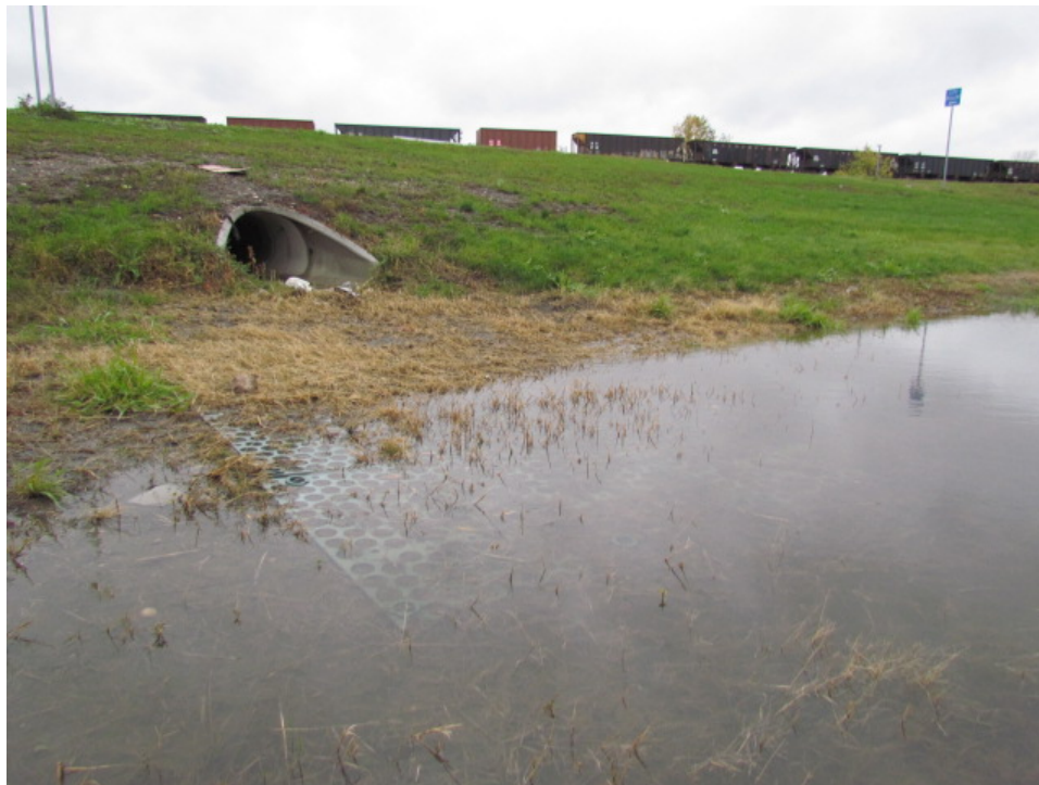
Photo 13: Installation at – Sta. 53+00 Rt. 1 st Evaluation (10/15/2013)
