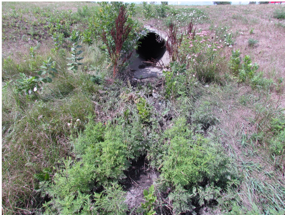
Photo 23: Final Evaluation Installation at - Sta. 47+90 Rt. (08/9/2017).
