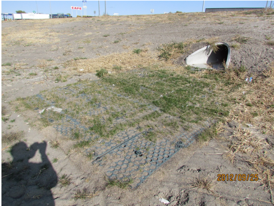
Photo 12: Installation at - Sta. 53+00 Rt. (9/25/2012)
