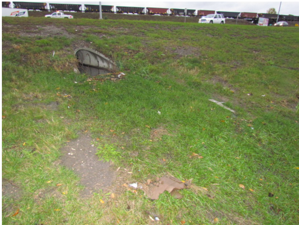
Photo 11: Installation at – Sta. 50+36 Rt. 1 st Evaluation (10/15/2013)
