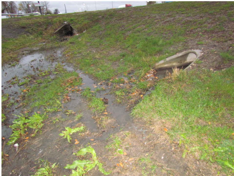
Photo 9: Installation at - Sta. 48+25 Rt. 1 st Evaluation (10/15/2013)
