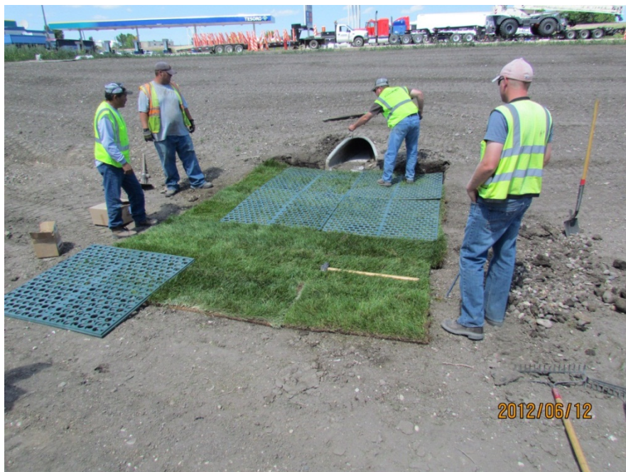
Photo 3: Crew placing the ScourStop® panels.
