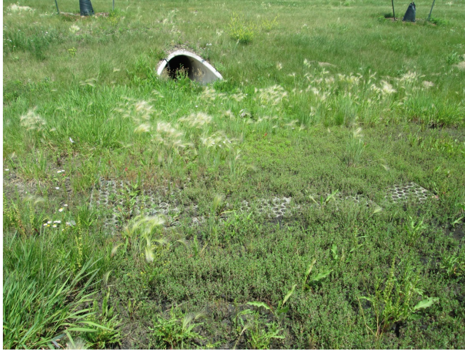
Photo 21: 2nd Evaluation Installation at – Sta. 53+00 Rt. (07/9/2015)
