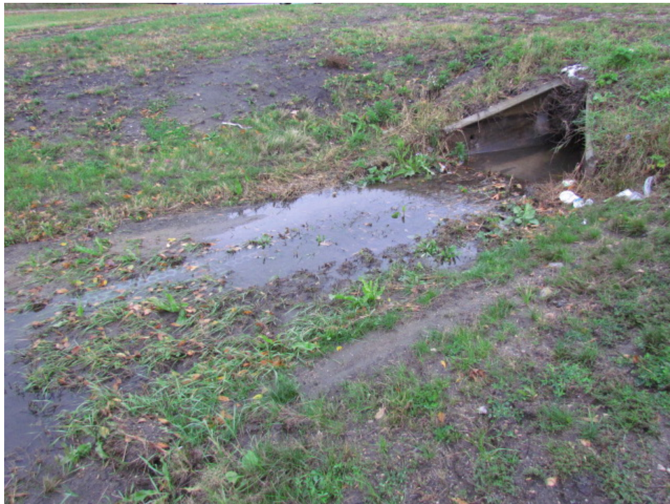
Photo 7: Installation at - Sta. 47+90 Rt. 1 st Evaluation (10/15/2013)
