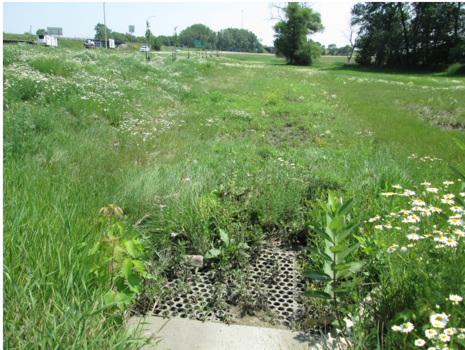
Photo 18: 2 nd Evaluation Installation at - Sta. 47+90 Rt. (07/9/2015).
