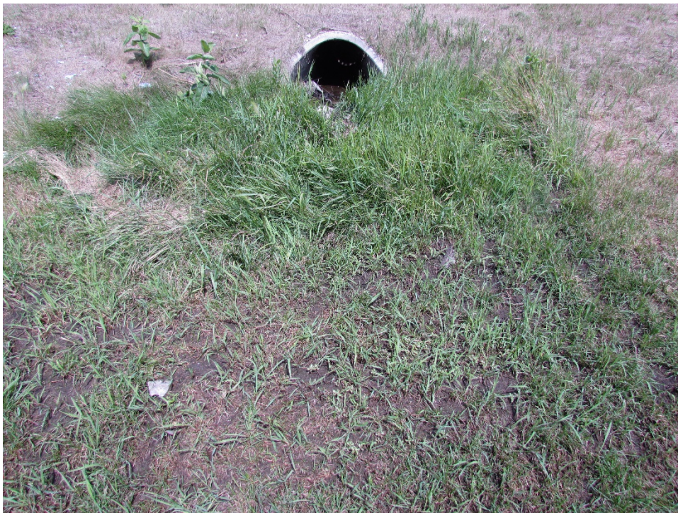
Photo 25: Final Evaluation Installation at - Sta. 50+36 Rt. (08/9/2017).
