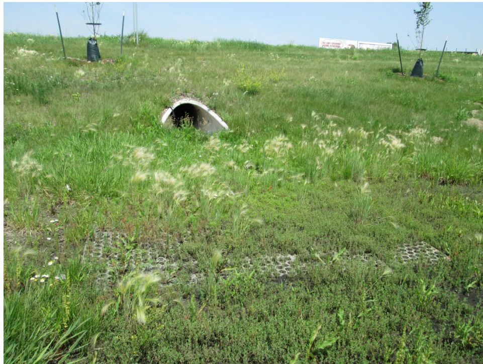
Photo 30: ScourStop® STA 53+00 Rt. Installation (July 9, 2015.)
