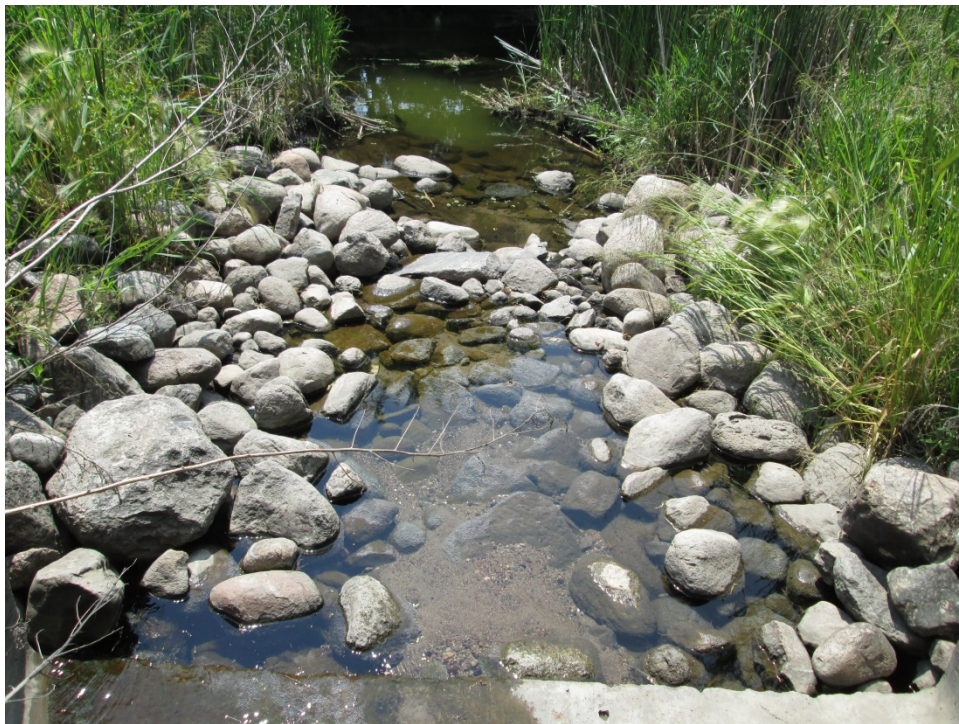
Photo 22: 2nd Evaluation Control Installation Sta. 24+36 Rt. to Sta. 24+57 Rt. (7/9/15)
