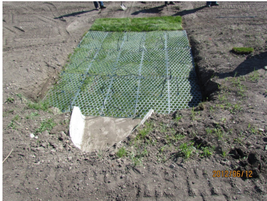
Photo 5: Completed ScourStop® installation.
