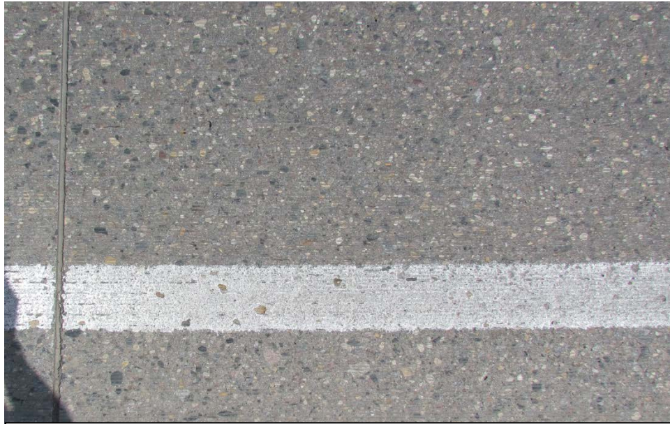
Photo 7 – White Water-based Paint Southbound - AWP – 6/3/14
