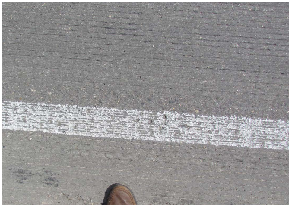
Photo 6 – White Water-based Paint Southbound – Standard Paint – 6/3/14
