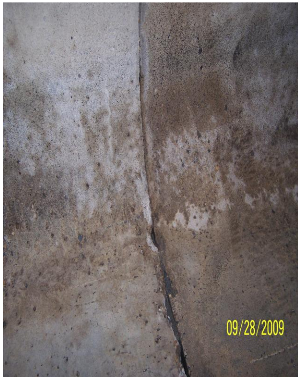
Photo 122: N13 South Haunch
