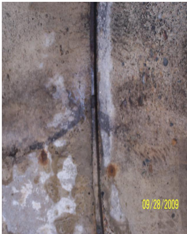
Photo 114: N11 South Haunch
