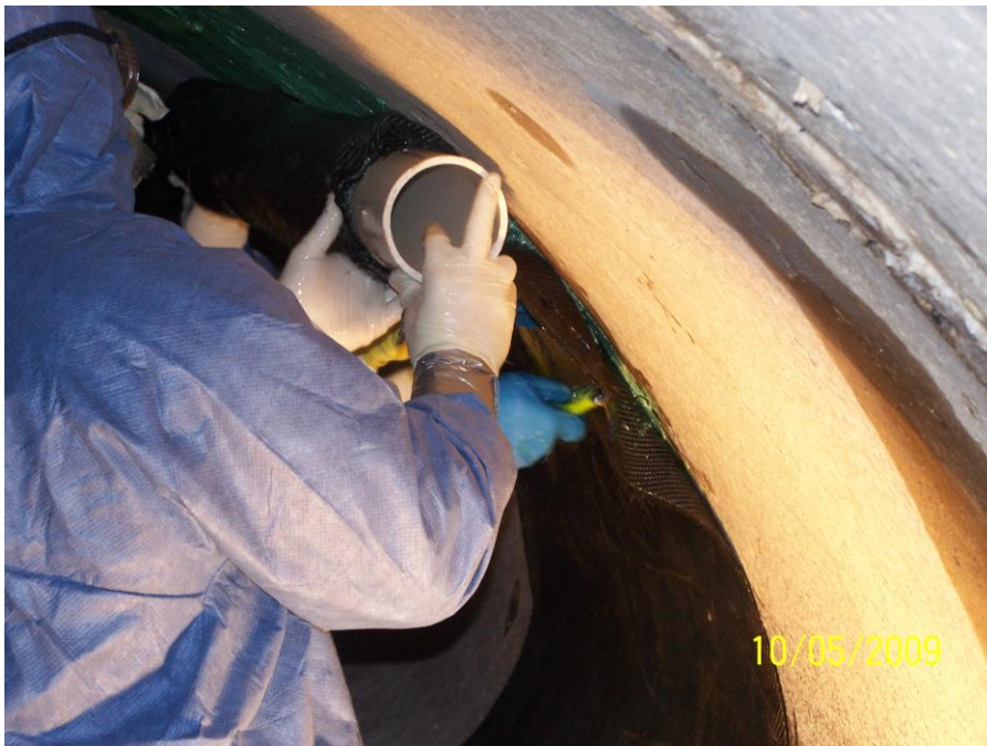
Photo 144: QuakeWrap™ TB20C Carbon Fabric being installed
