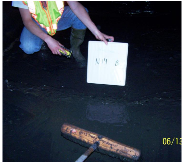
Photo 150: Joint repair before excavation in 2011
