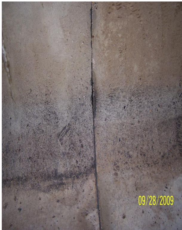
Photo 86: N4 South Haunch
