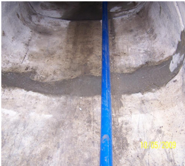
Photo 147: After repair in 2009
