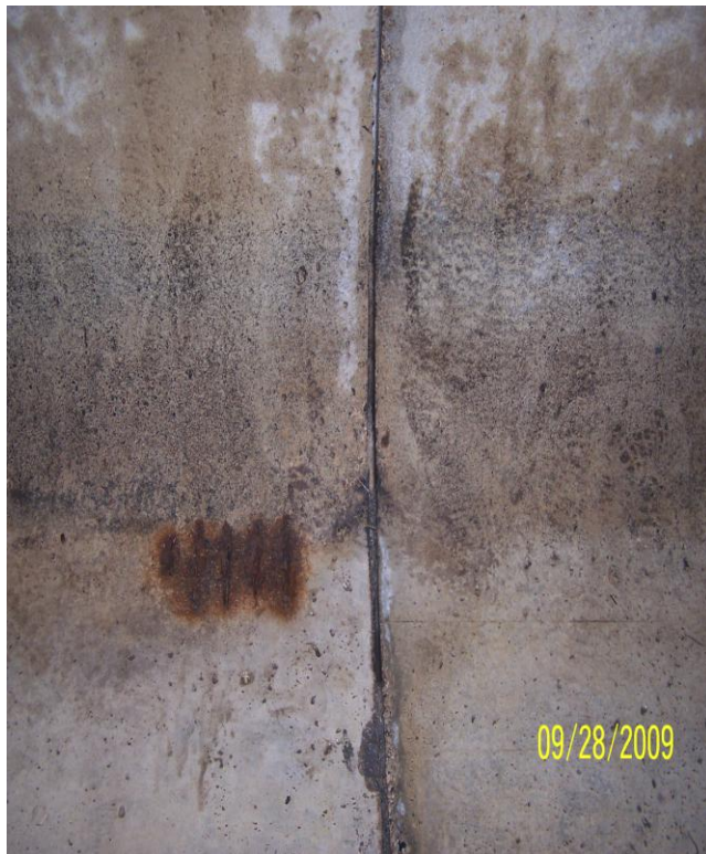
Photo 94: N6 South Haunch
