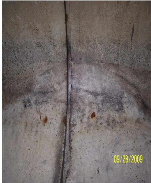
Photo 89: N5 North Haunch
