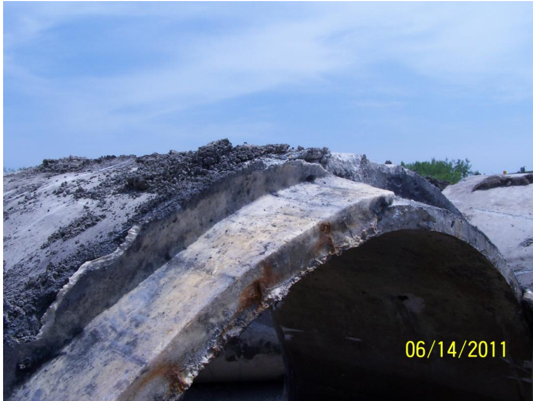
Photo 175: Flexible sealant on the bell side after excavation.
