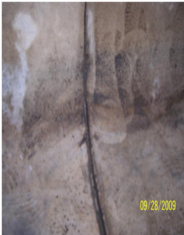
Photo 106: N9 South Haunch
