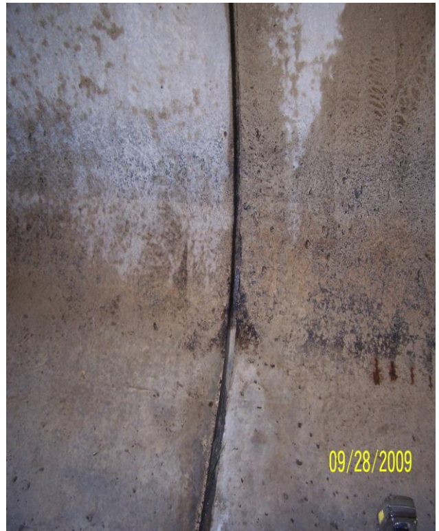
Photo 93: N6 North Haunch
