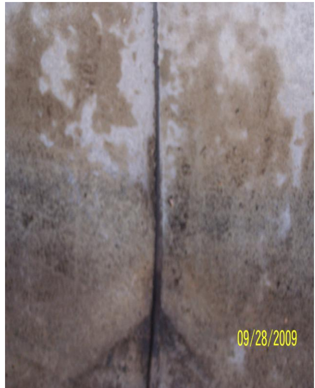
Photo 109: N10 North Haunch
