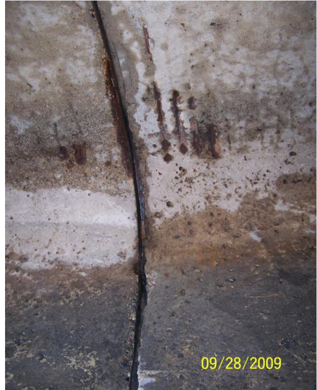
Photo 129: N15 North Haunch
