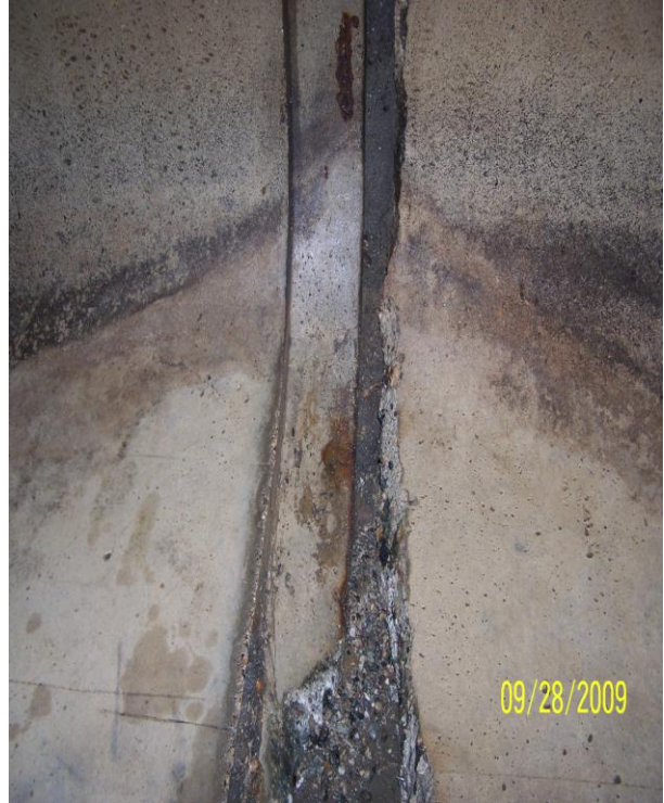
Photo 81: N3 North Haunch
