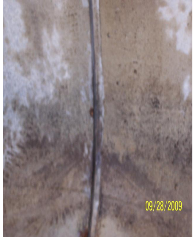
Photo 113: N11 North Haunch
