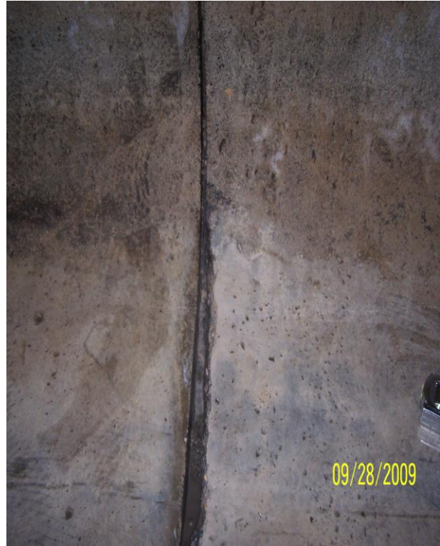
Photo 97: N7 North Haunch
