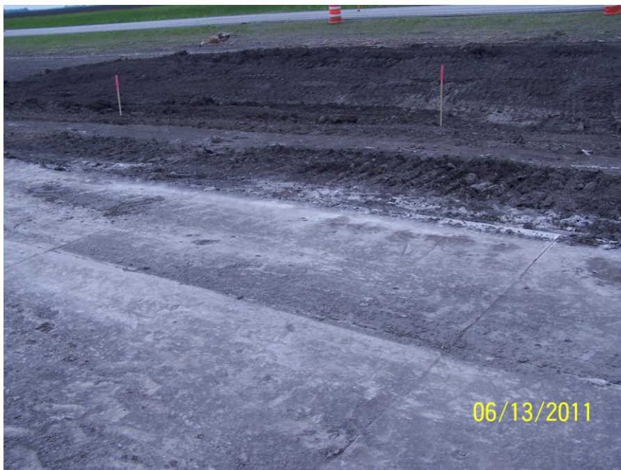
Photo 162: Slabs cut into 10' x 4' slabs to be removed.
