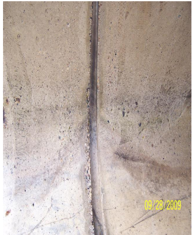
Photo 75: N1 South Haunch
