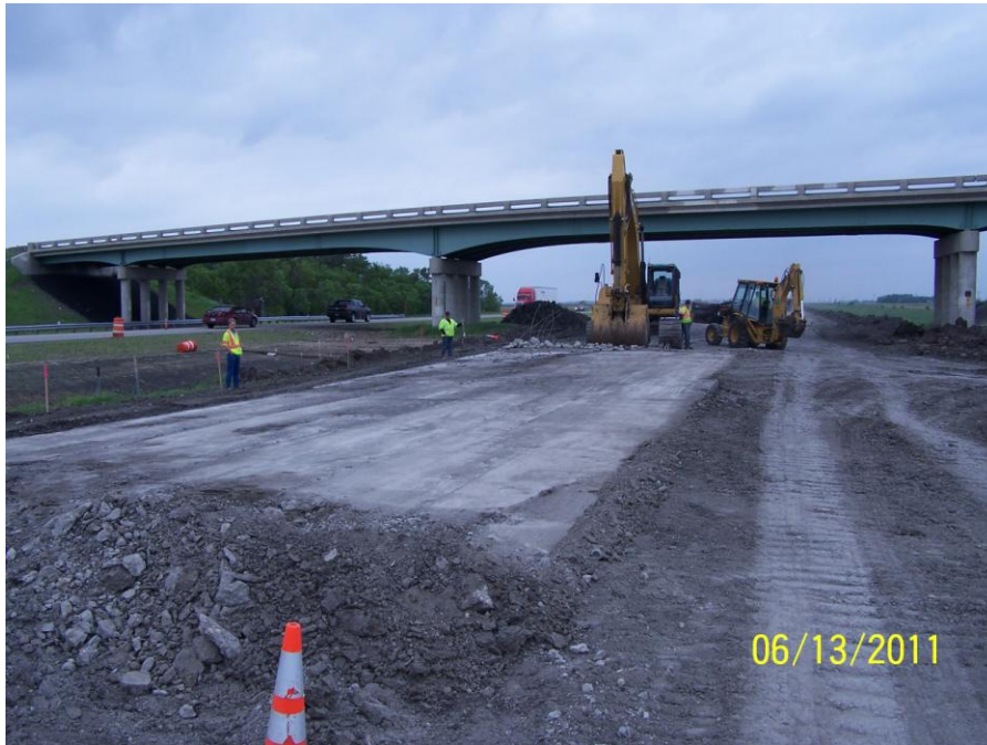
Photo 161: Work zone for forensic excavation.
