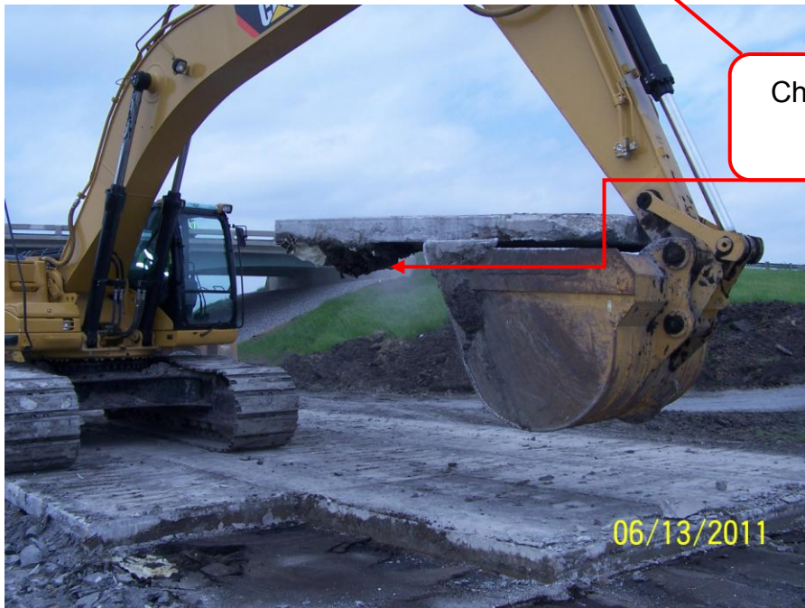
Photo 164: Backhoe removing concrete slab.
