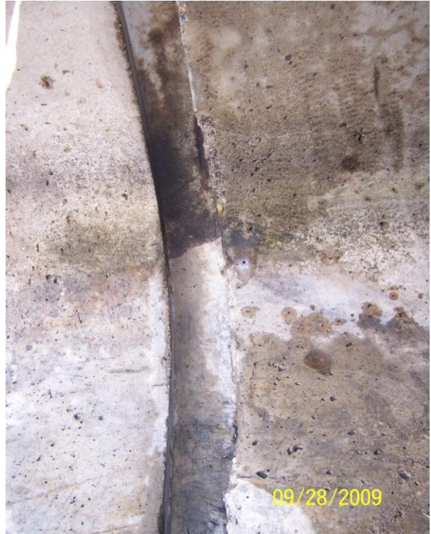
Photo 133: N16 North Haunch
