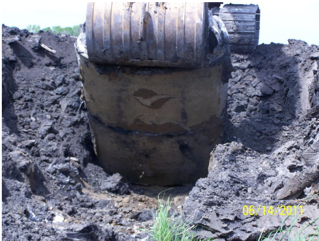
Photo176: Two sections of pipe being held together by QuakeWrap.
