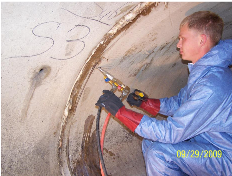
Photo 139: Subsurface injecting flexible foam
