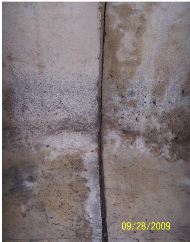
Photo 30: S5 South Haunch
