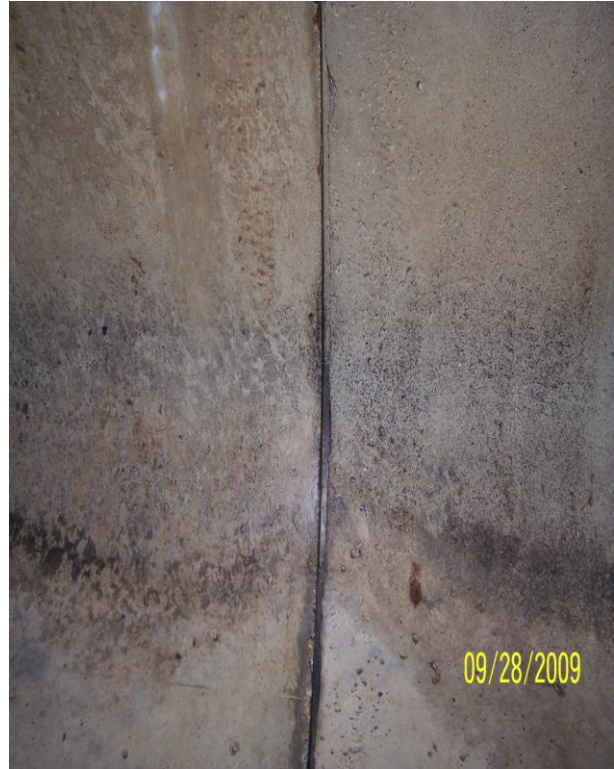
Photo 85: N4 North Haunch
