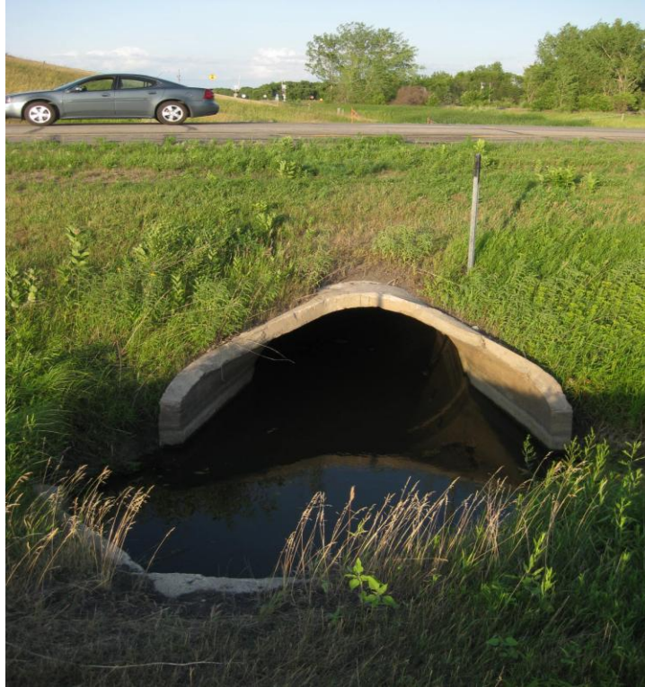
Photo 3: Inlet of pipe at roadway median
