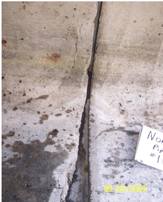
Photo 134: N16 South Haunch
