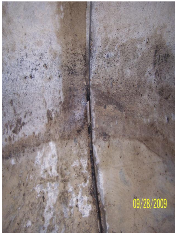
Photo 118: N12 South Haunch
