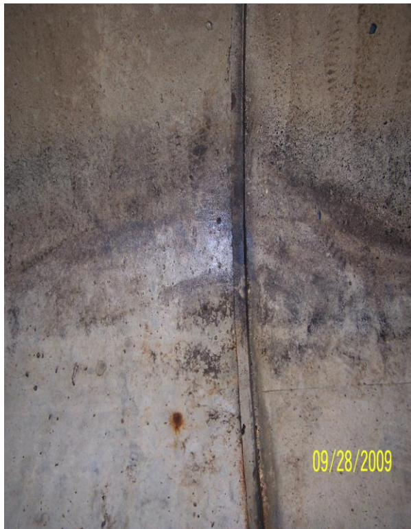
Photo 90: N5 South Haunch
