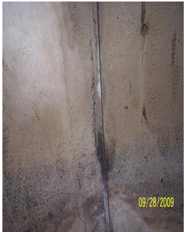
Photo 83: N3 South Haunch
