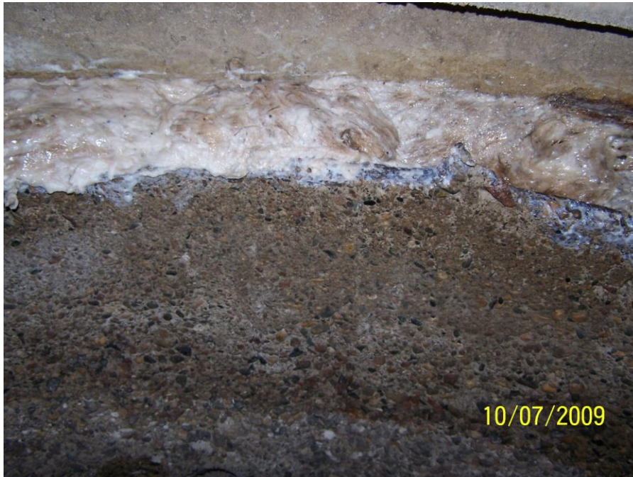
Photo 138: Oakum Rope and 900 XLV Foam expanded in pipe joint.
