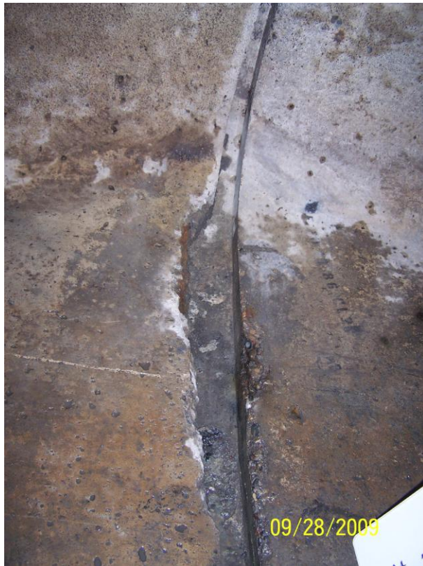
Photo 126: N14 South Haunch
