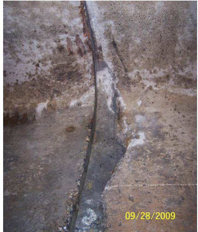
Photo 125: N14 North Haunch
