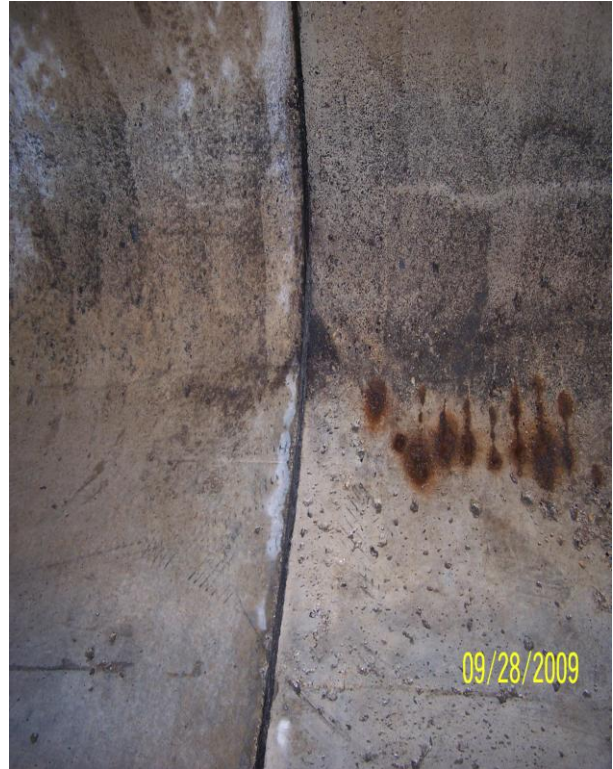
Photo 101: N8 North Haunch
