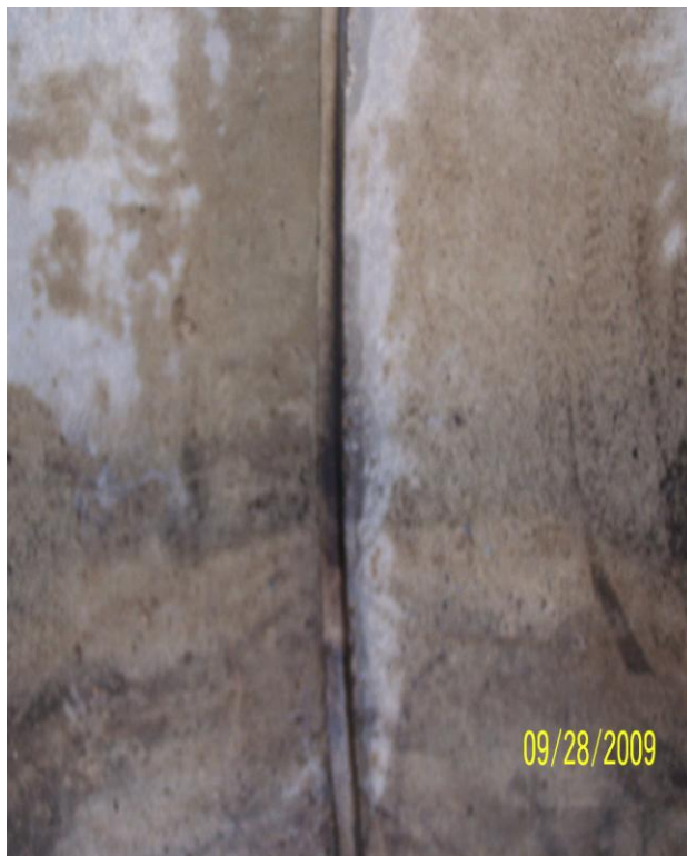
Photo 110: N10 South Haunch
