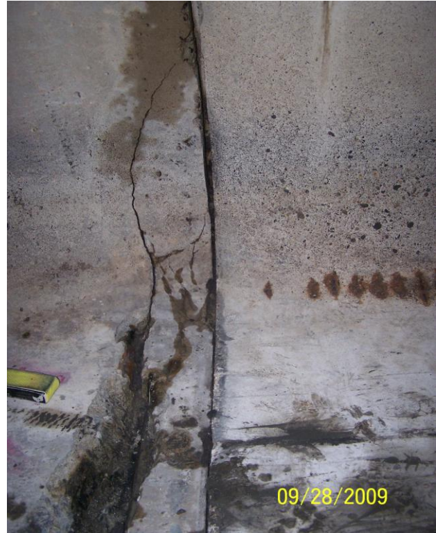
Photo 57: S13 North Haunch
