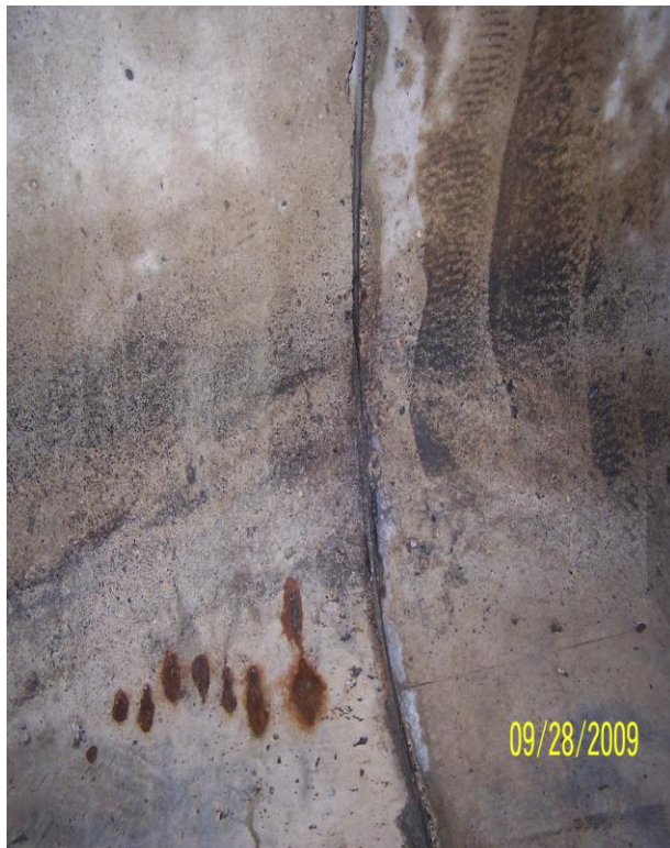
Photo 102: N8 South Haunch
