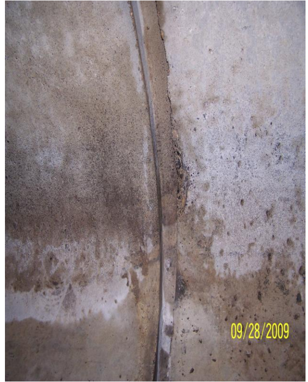
Photo 121: N13 North Haunch
