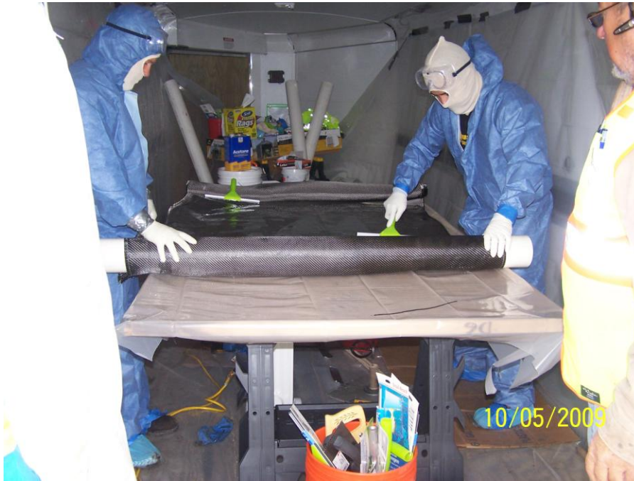
Photo 142: QuakeWrap being saturated before installation
