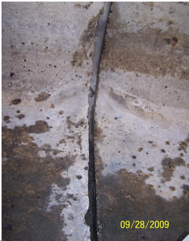
Photo 130: N15 South Haunch
