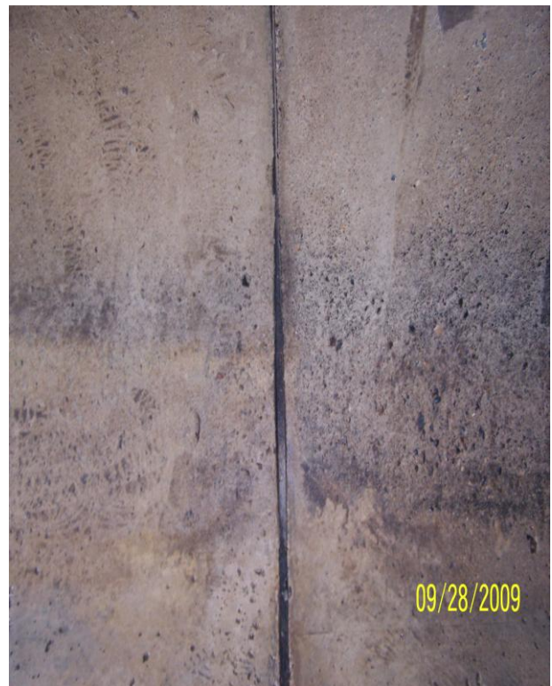
Photo 79: N2 South Haunch
