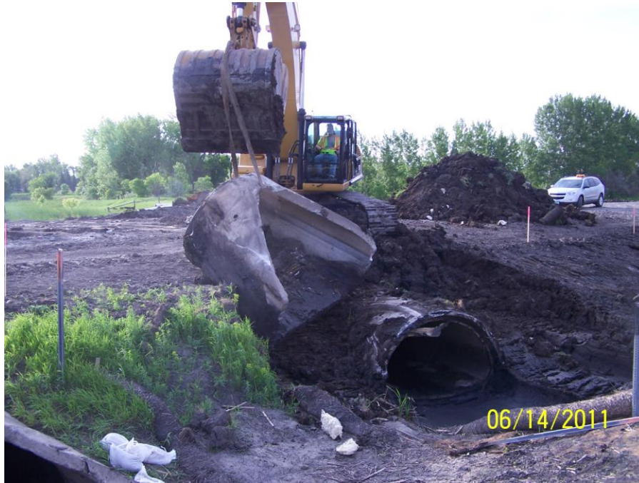
Photo 146: Northern Improvement removing I-29 arch pipe section.
