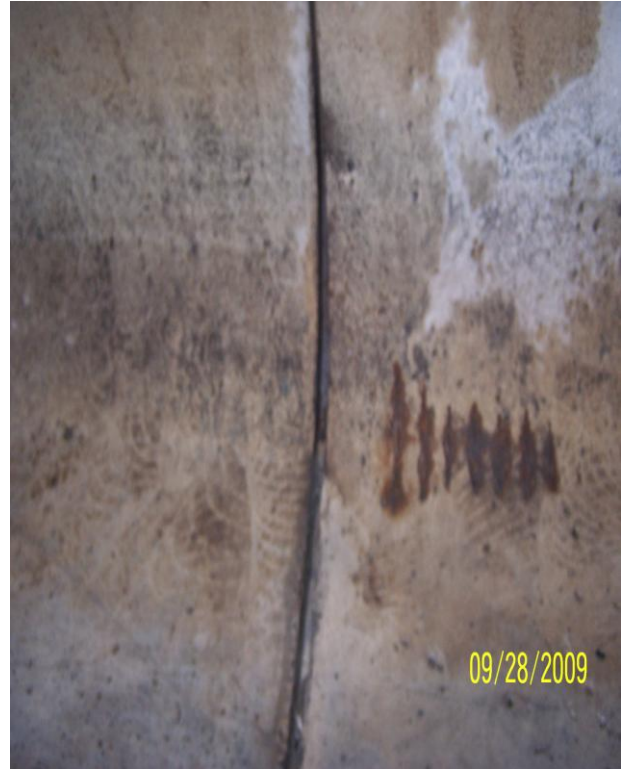
Photo 105: N9 North Haunch
