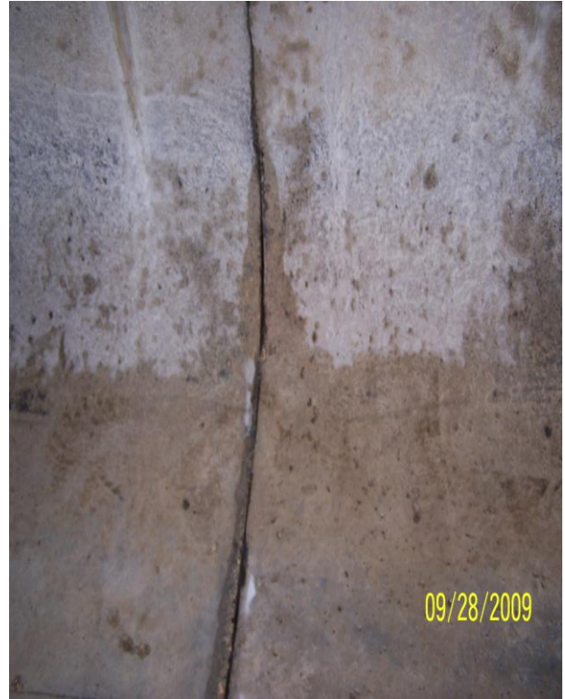
Photo 117: N12 North Haunch
