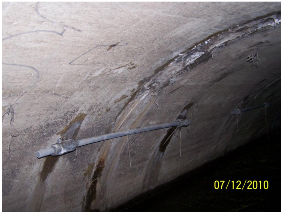
Photo 141: Internal pipe tie installed.
