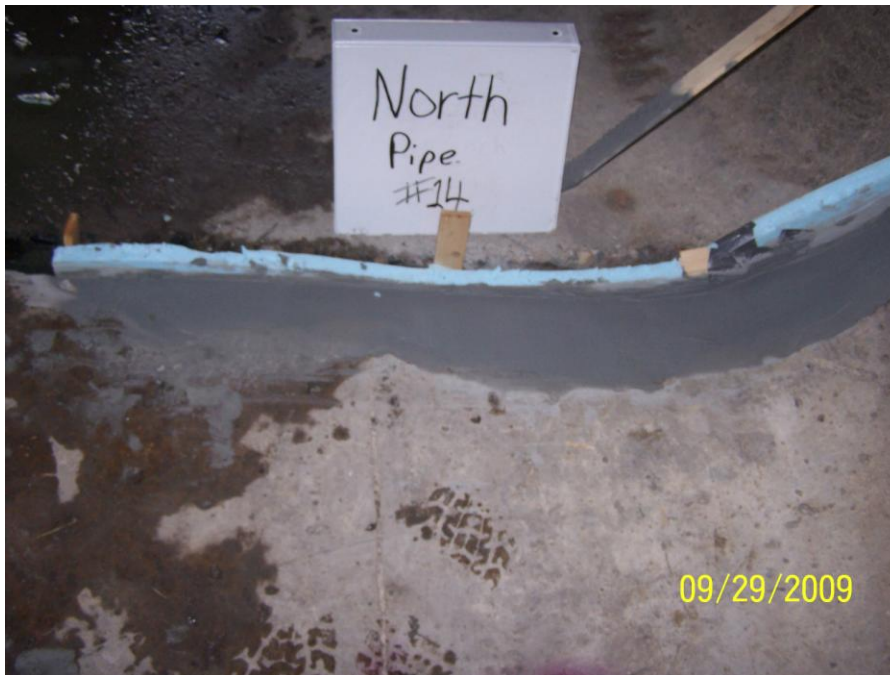
Photo 137: Subsurface did joint rehabilitation with a product called Verticote Supreme
