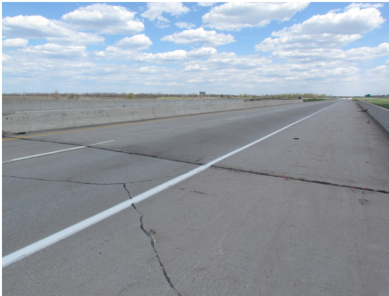
Photo 30: FLEXOGRID™ Installation Looking East
