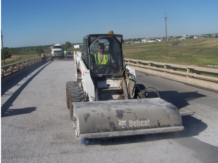
Photo 11: Contractor Using Power Broom
