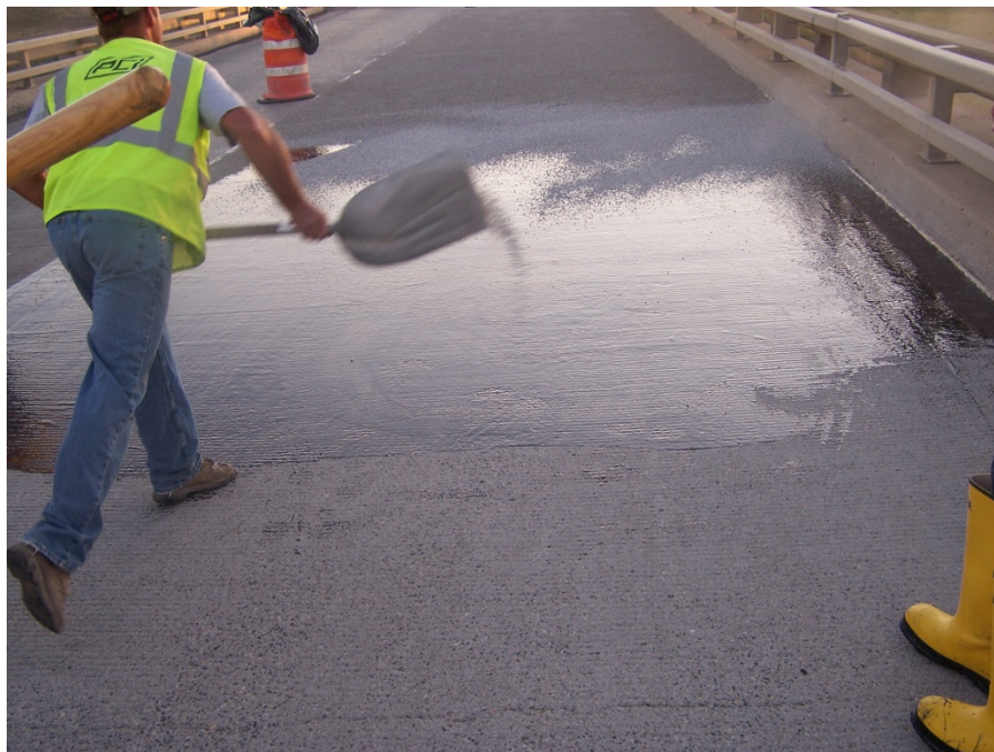
Photo 9: PCI Spreading SafeLane™ Aggregate
