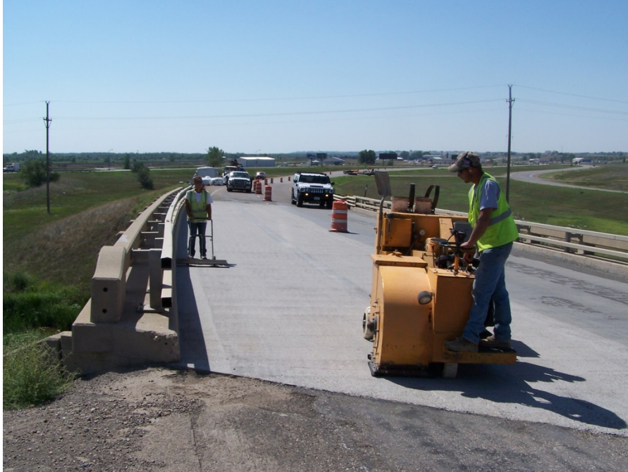
Photo 4: Progressive Contractors Incorporated (PCI) Shot Blasting a Concrete Bridge Deck
