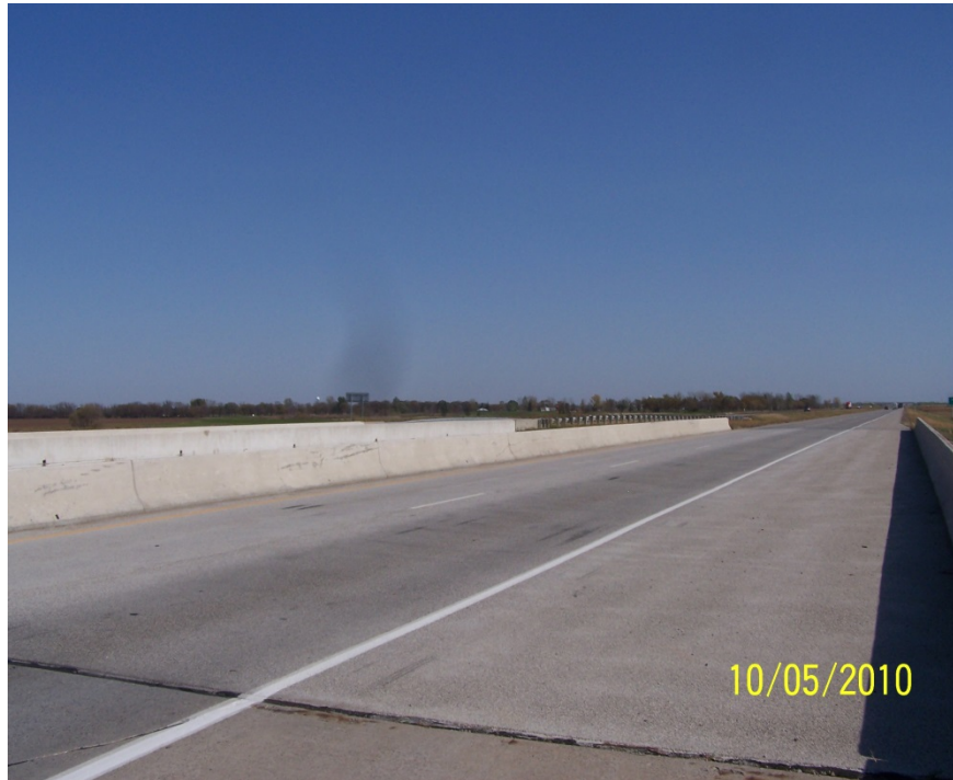
Photo 24: FLEXOGRID™ Installation Looking East
