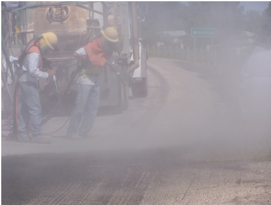
Photo 5: PCI Sand Blasting Operation in Williston, ND
