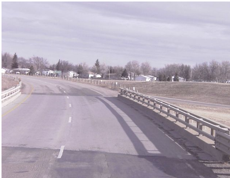
Photo 1: Sand Creek Bridge Eastbound
