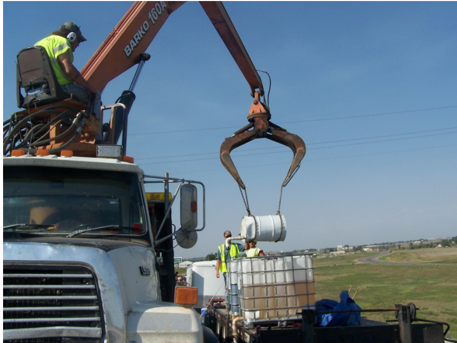
Photo 10: Contractor Refilling Plastic Totes With Epoxy
