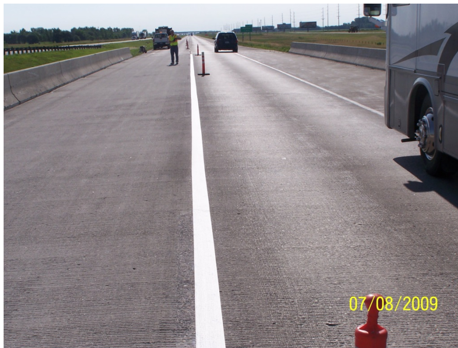
Photo 16: Maple River Bridge Deck Prior to Installation
