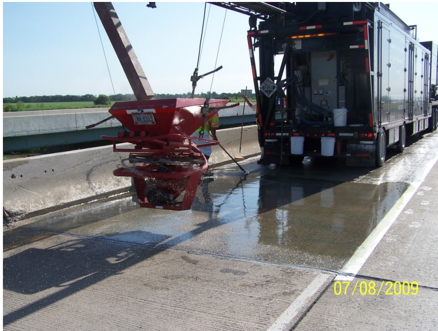
Photo 15: FLEXOGRID™ Installation Semi-Trailer
