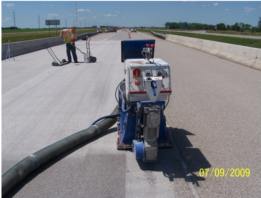
Photo 17: SURF-PREP INC. Shot Blasting
