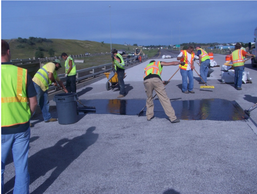
Photo 15: Traffic Safety Services Applying Second Course
