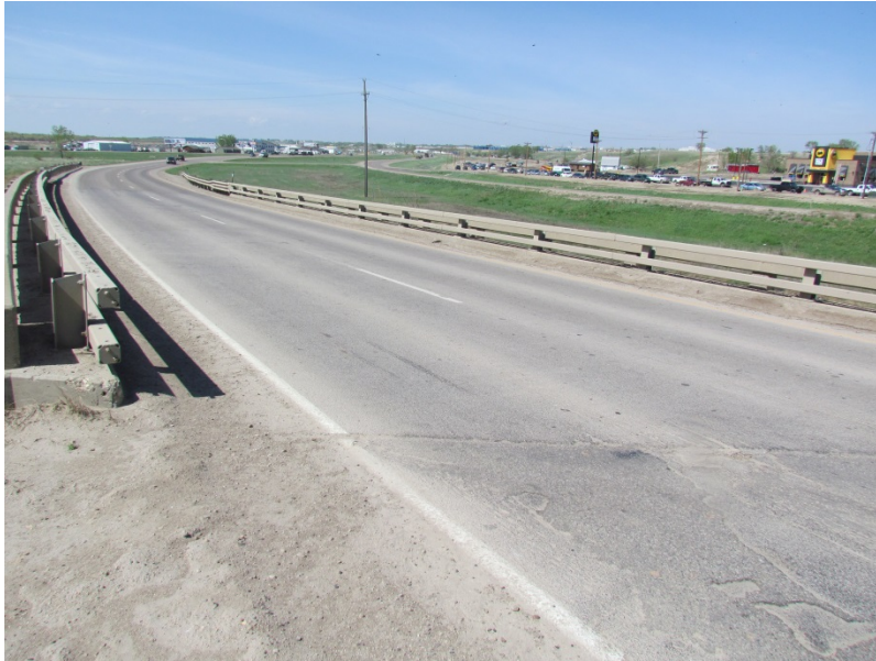
Photo 26: SafeLane™ Facing West
