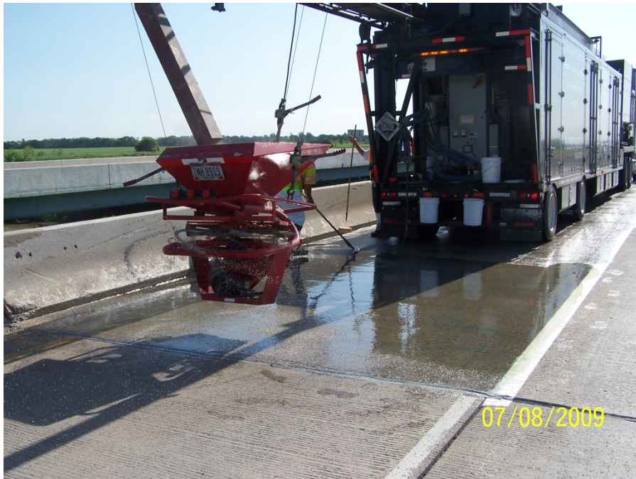
Photo 19: Contractor Applying First Pass Application
