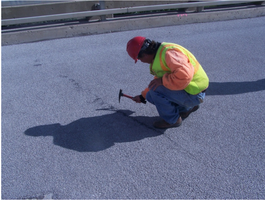
Photo 14: Project Engineer Inspecting Hand Mixed Portion
