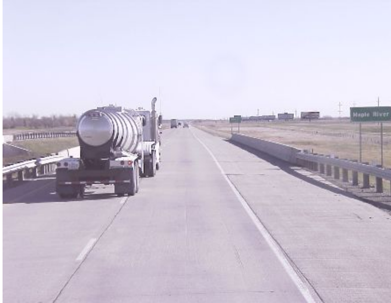
Photo 3: Maple River Bridge Westbound
