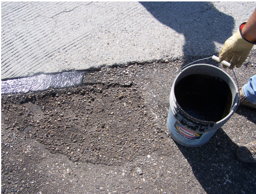
Photo 6: Slurry Seal
