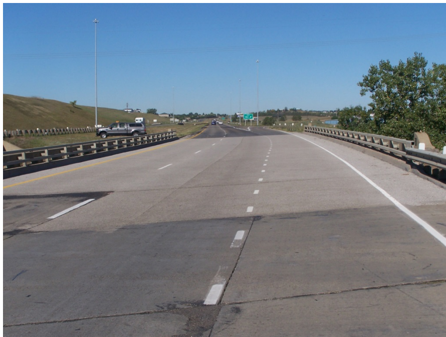
Photo 13: BNRR and Missouri Road Structure With the SafeLane™ Application
