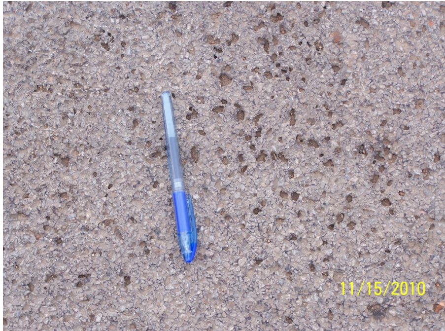
Photo 21: Small Pockets Were Evident in the Aggregate
