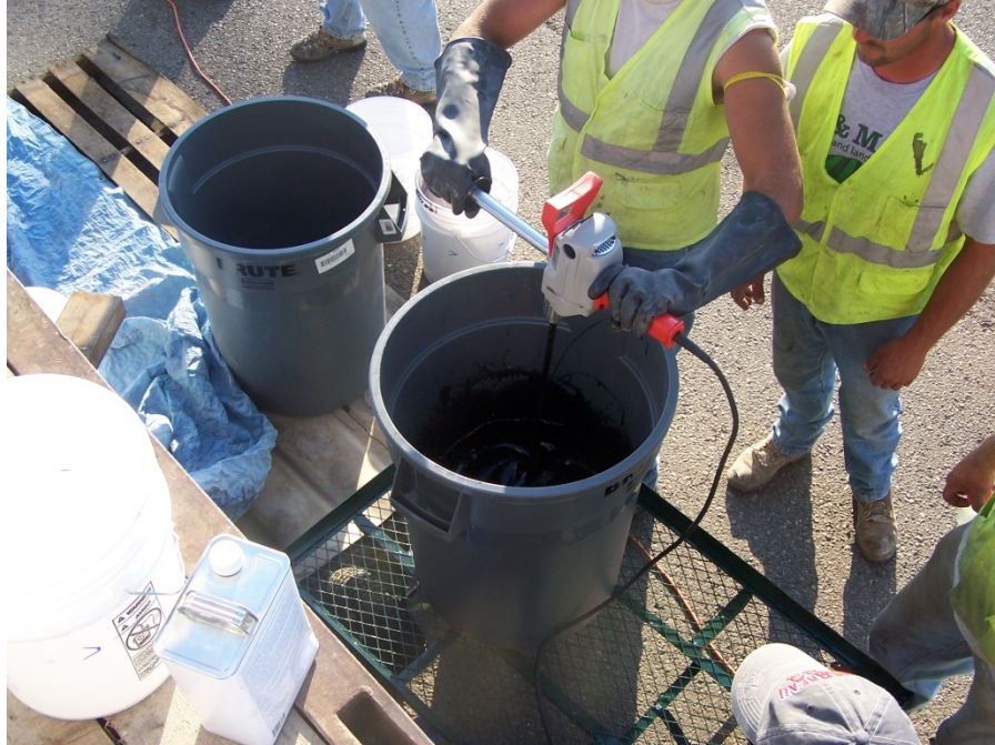
Photo 8: PCI Mixing Epoxy with a Drill and Paddle End
