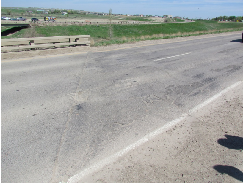
Photo 27: SafeLane™ Asphalt Portion
