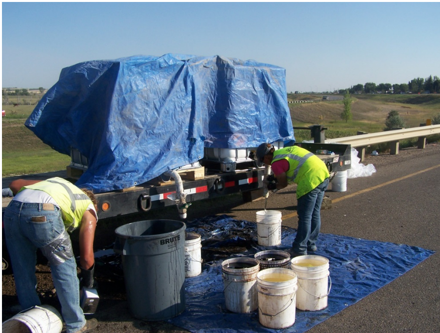
Photo 7: PCI Pouring Two Part Epoxy into Five Gallon Buckets
