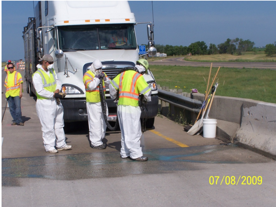
Photo 18: Contractor Applying Crack Sealer During First Pass of Passing Lane
