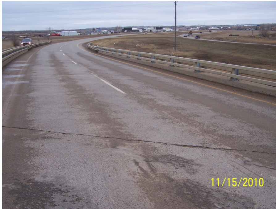
Photo 20: SafeLane™ Facing West
