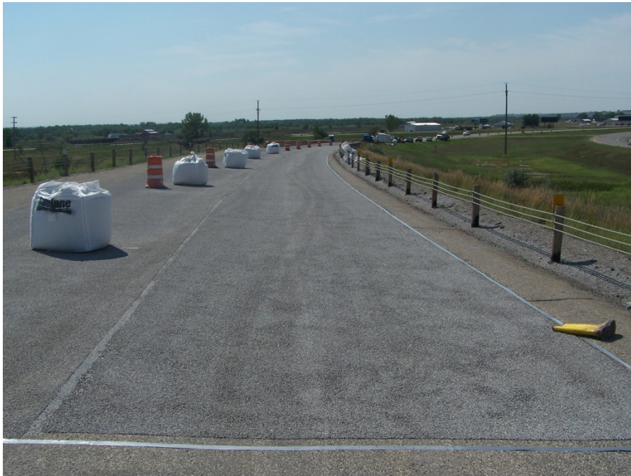
Photo 12: Aggregate Staged for Second Course
