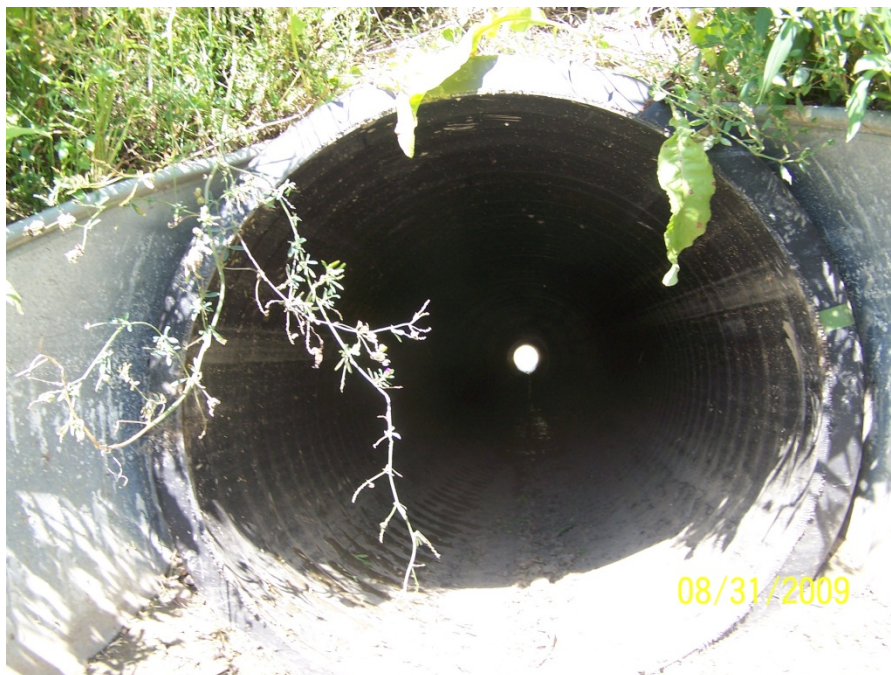
Photo 3:End Section of Pipe
