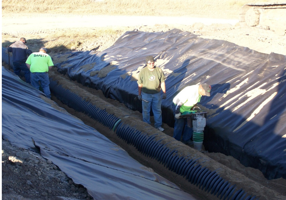
Photo 1: Centerline HDPE pipe being installed
