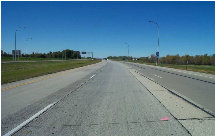
Photo 7 - Overall view of the experimental section.
