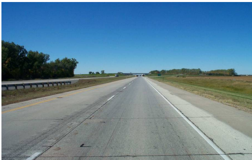
Photo 5 - Overall view of control section 2.
