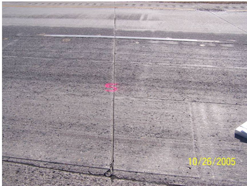
Photo 8 - Typical joint in experimental section.
