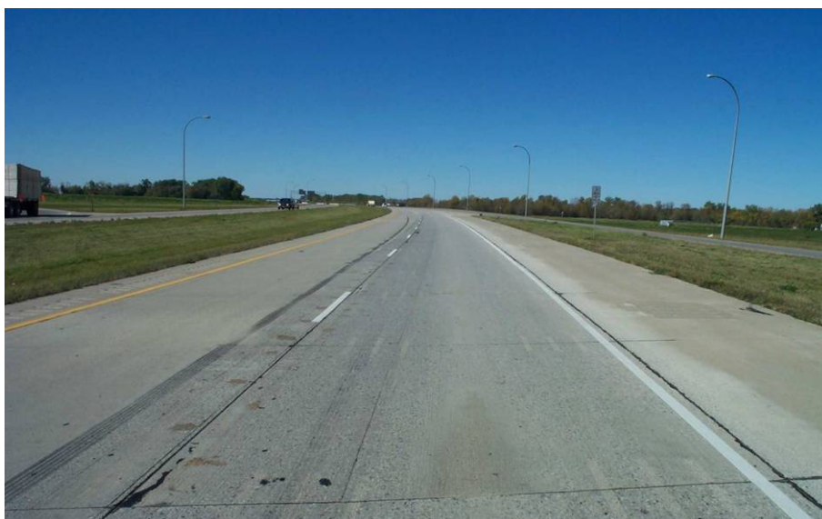
Photo 1 - Overall view of control section 1.
