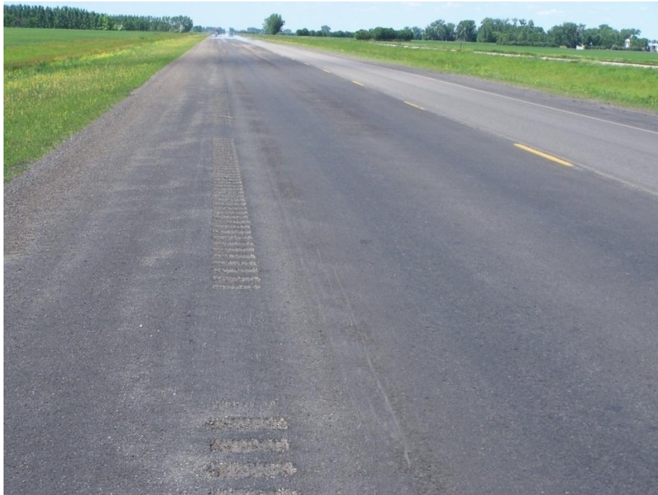
Photo 2 – Blade patching after final paver lift.
