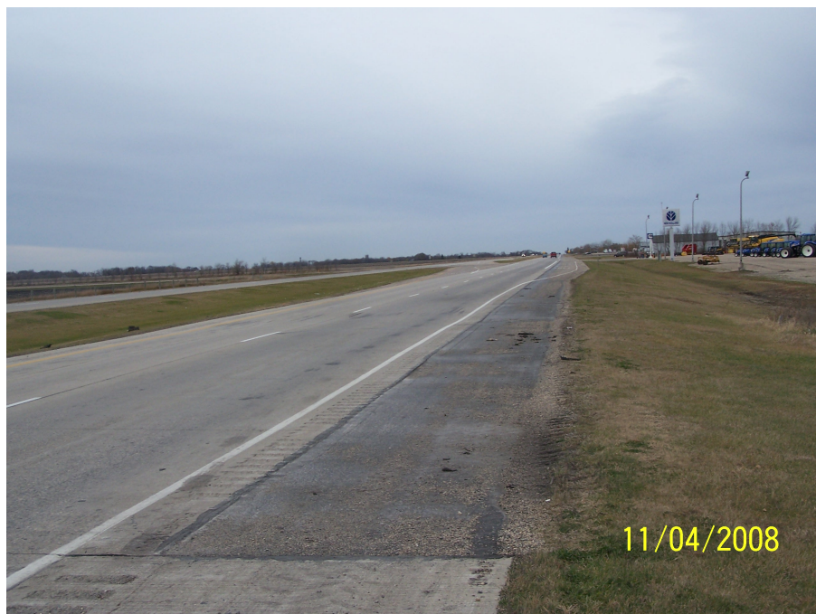
Photo 1 – Asphalt shoulder near implement dealership at transition between Segments 2 and 3.
