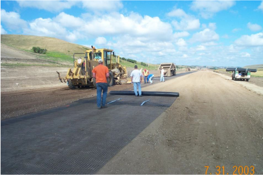
Photo 4 – Starting new roll of geogrid.
