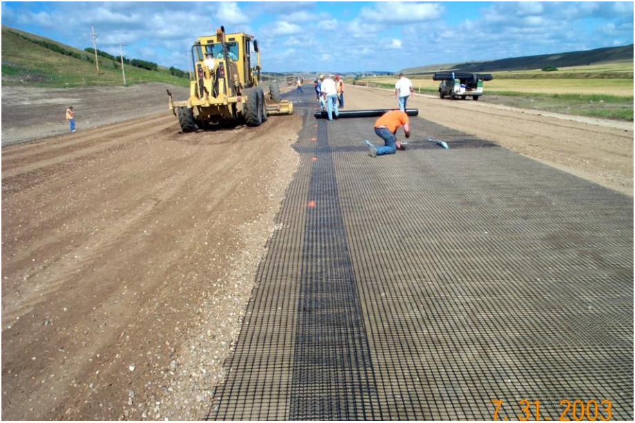
Photo 5 – Nailing down overlap of new roll, rolling out geogrid, and spreading base material.
