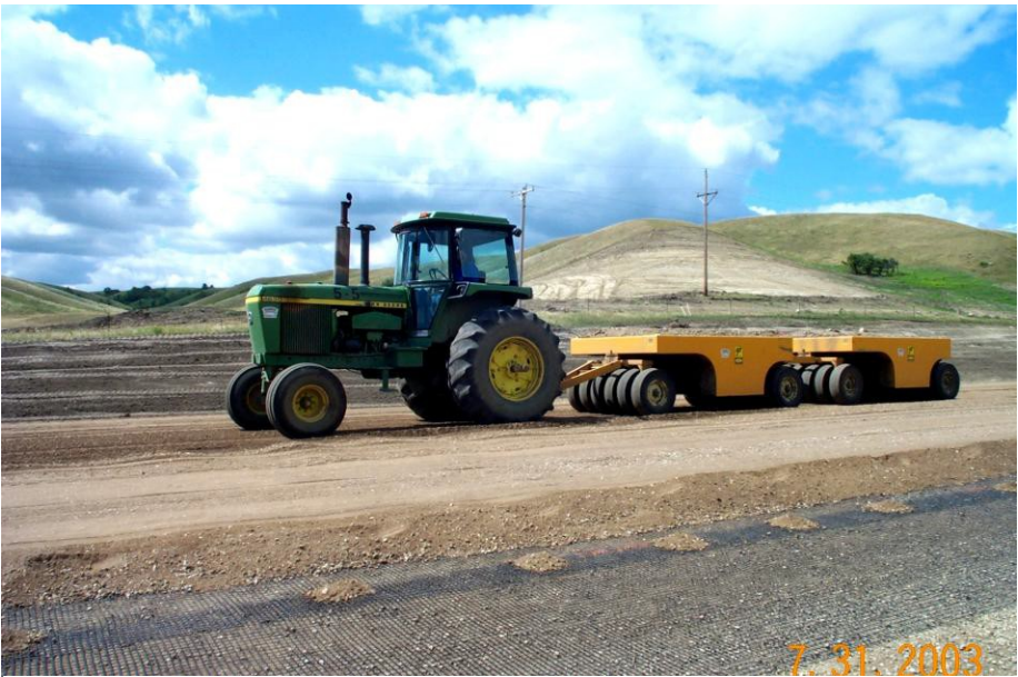
Photo 11 - Compacting the base material on top of the geogrid.
