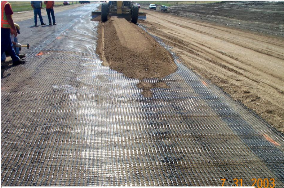
Photo 10 – Some waves in the geogrid – nailing overlap area.
