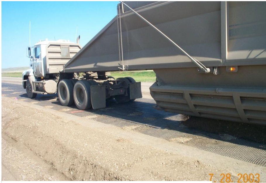
Photo 8 – Placing the base material on the geogrid.
