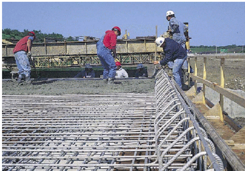
Photo 10. Bridge deck being poured
