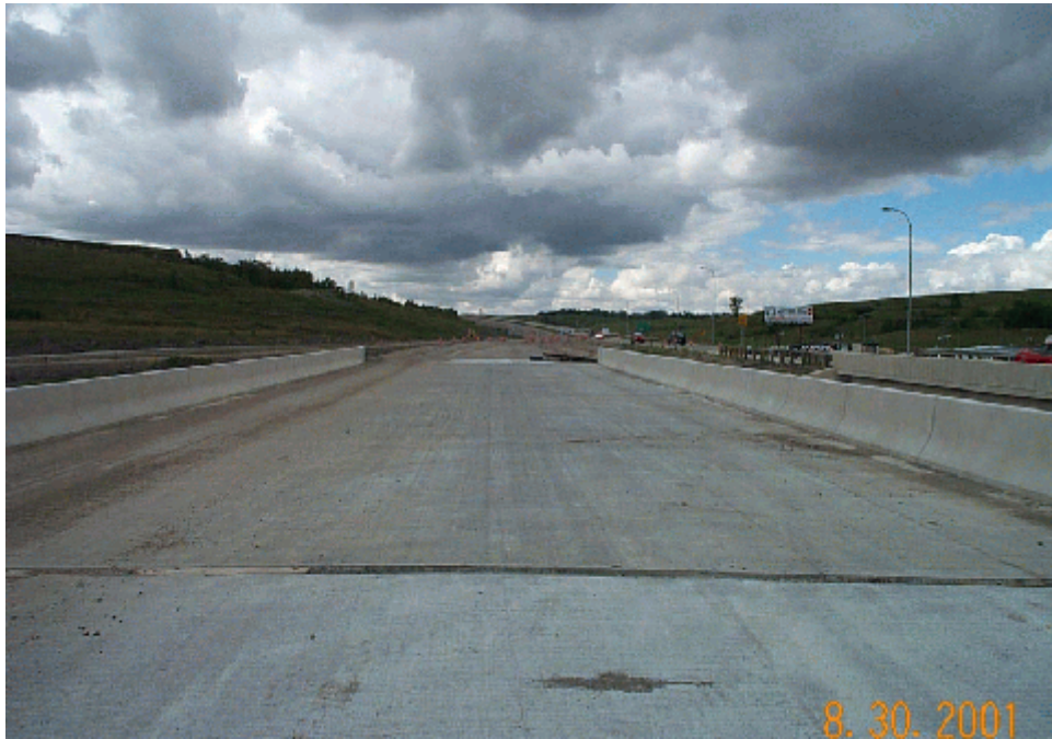
Photo 11. Finished bridge deck
