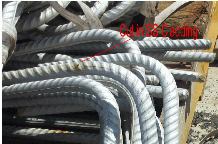
Photo 3. Cut in Stainless Steel Cladding
