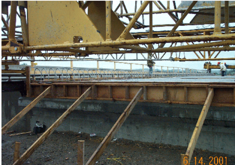
Photo 5. Bridge Deck Forms
