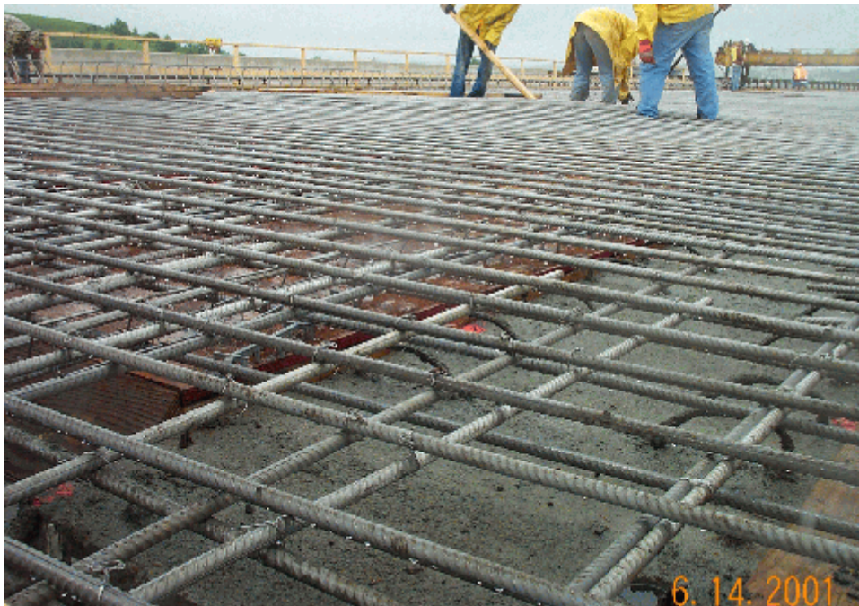
Photo 6. Placement of Stainless Steel Clad Rebar
