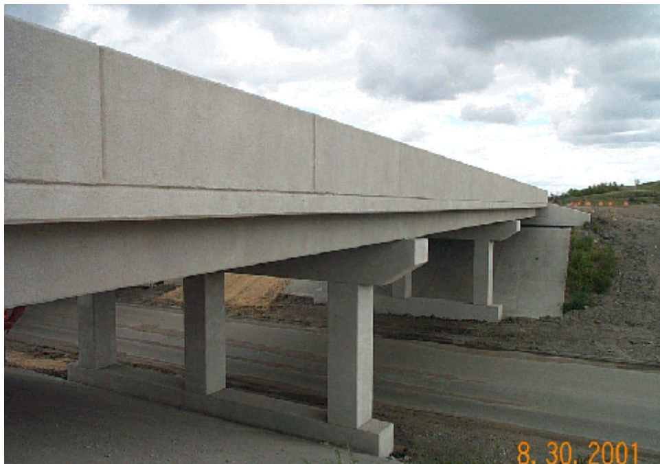
Photo 12. Side view of finished bridge deck
