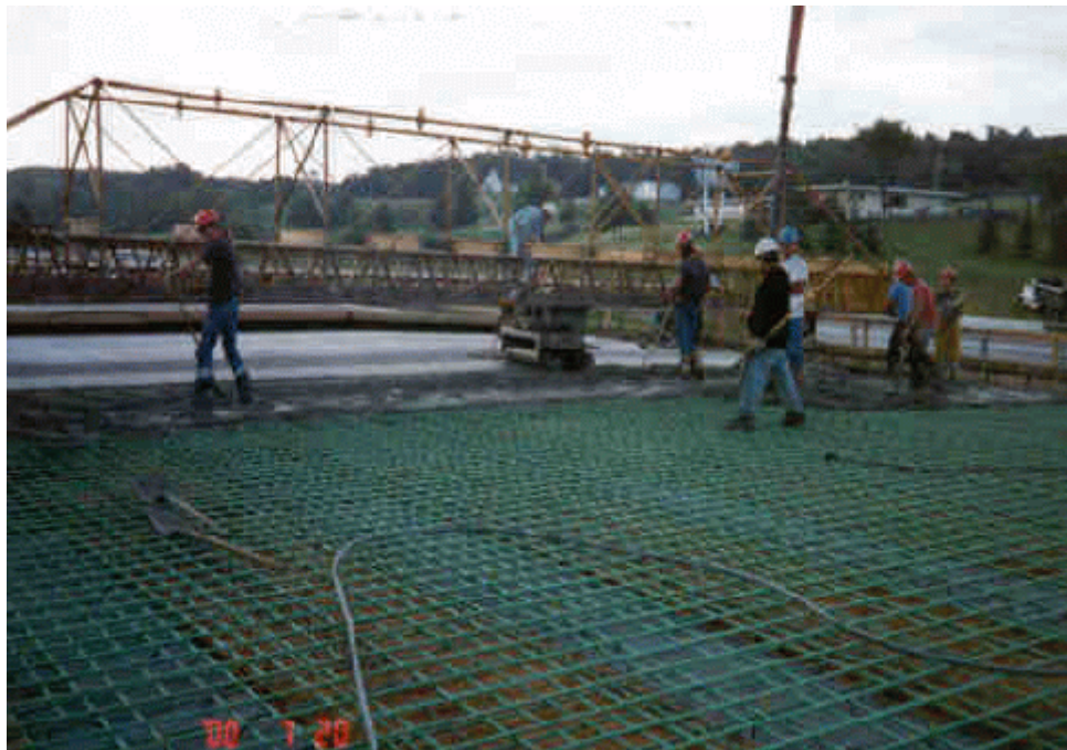
Photo 14. View of the control section bridge deck being poured
