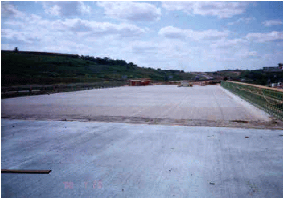
Photo 15. View of the control section bridge deck
