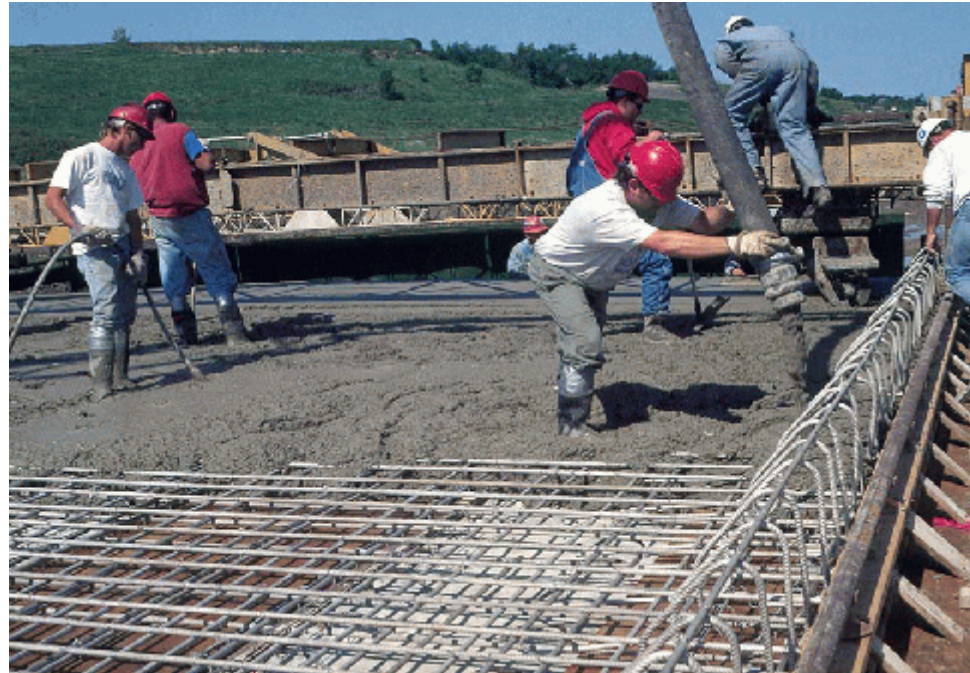
Photo 9. Bridge deck being poured
