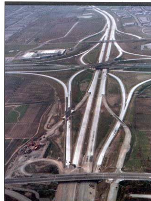
Delastic® Pavement Seals were successfully used on Route 407 near Toronto, Ontario.
