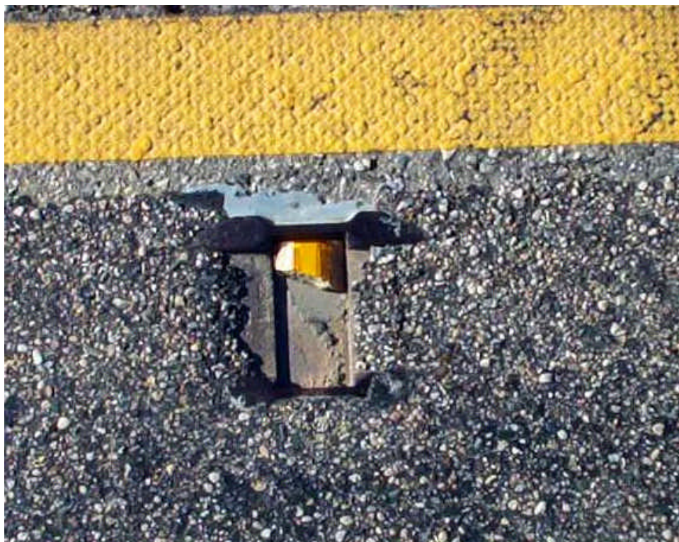
Photo 10 – A marker with a broken lens at US 52.
