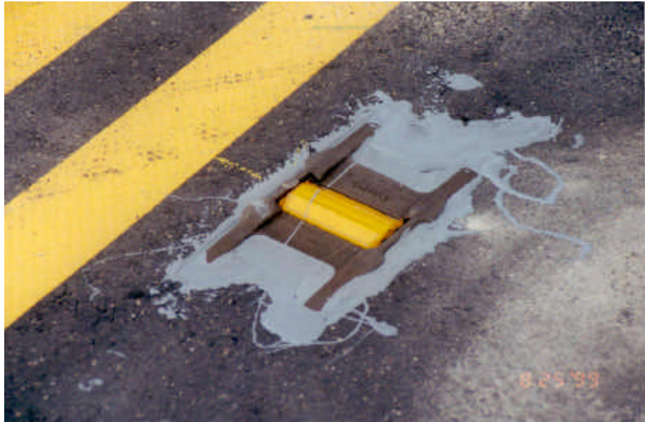
Photo 2 - A typical installation of a raised pavement marker.
