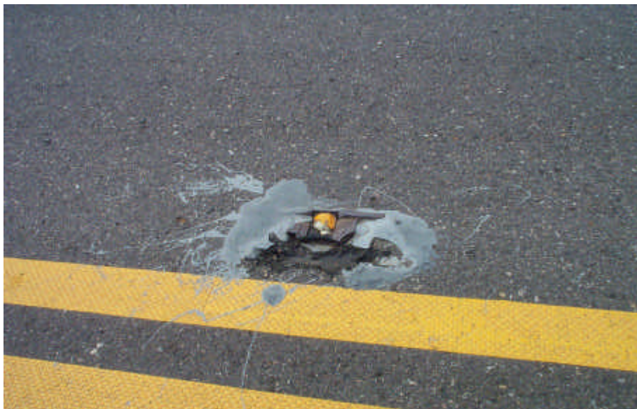
Photo 3 - A marker that had been partially removed by Section personnel.
