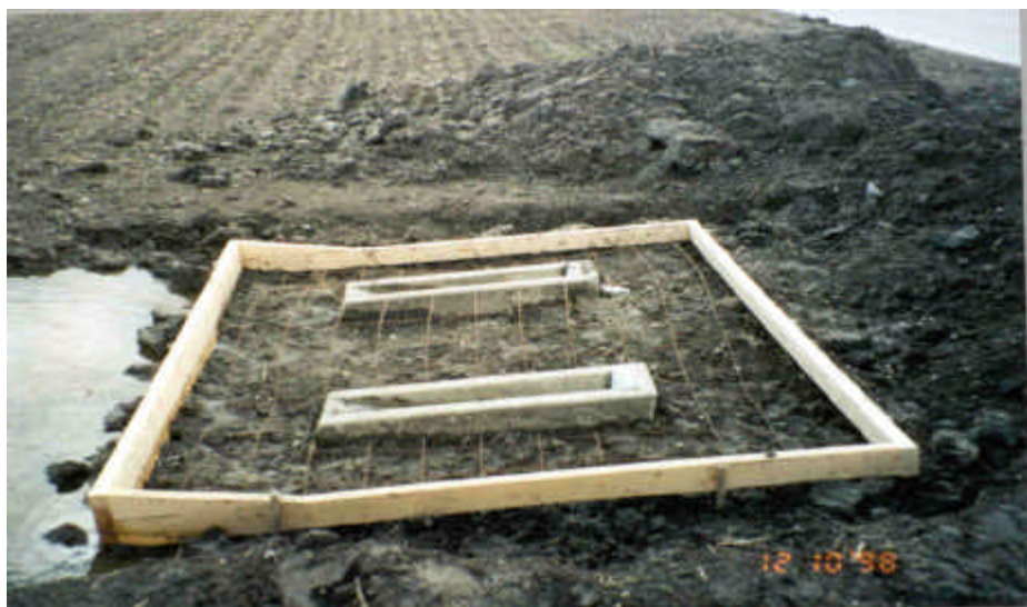
Photo 11 - Double concrete barrier.
