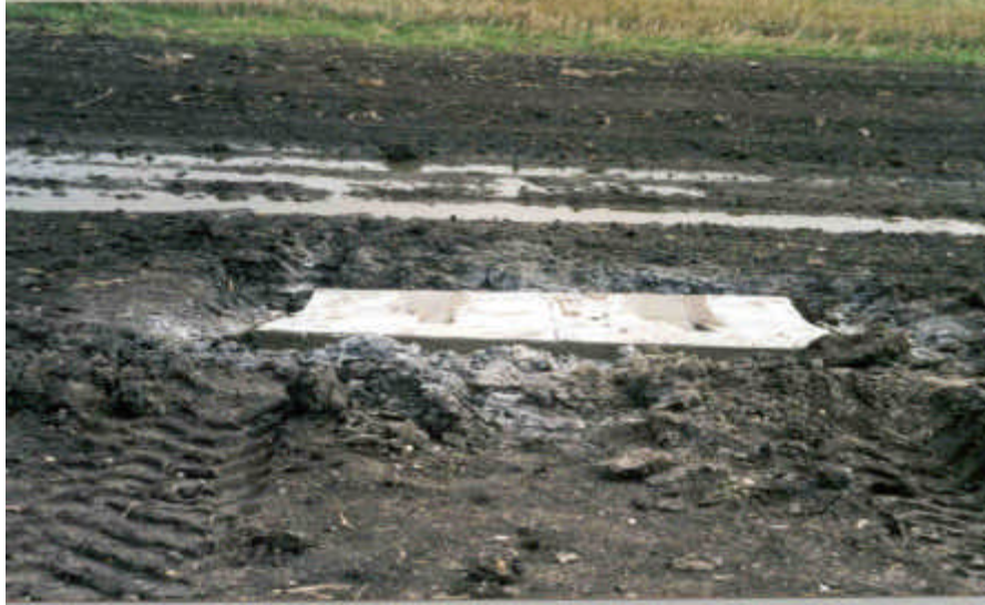
Photo 12 - Concrete barrier - top view.
