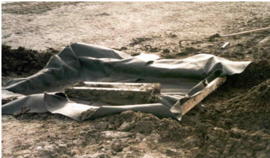
Photo 9 - Fabric in aggregate barrier.
