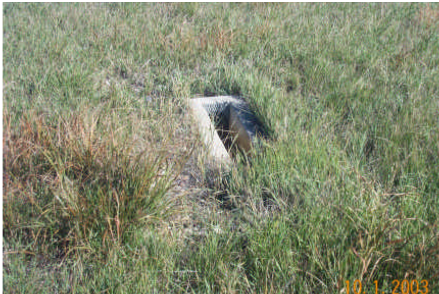
Photo 14 – Aggregate barrier – vegetation growth.
