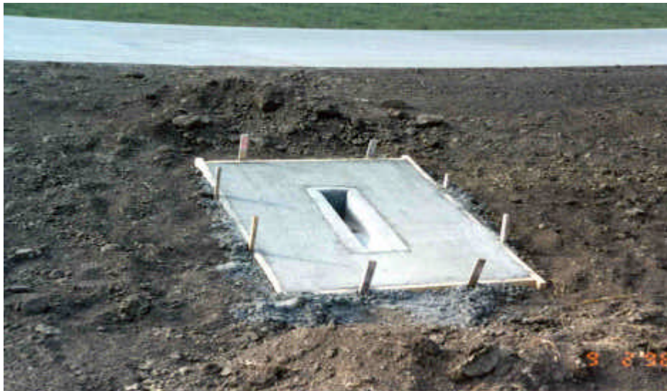
Photo 5 - Finished concrete barrier.
