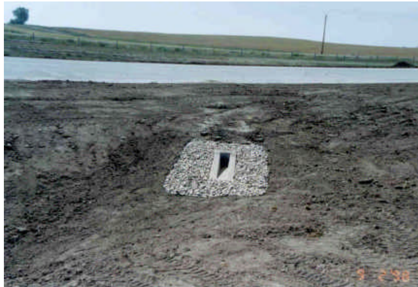
Photo 3 - Finished aggregate barrier.
