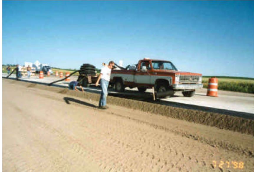
Photo 2 - Installing Drain.
