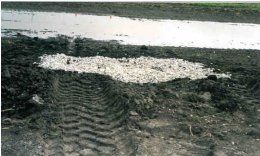
Photo 13 - Uneven surface - aggregate barrier.
