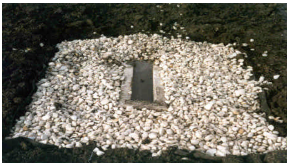
Photo 10 - Finished aggregate barrier.
