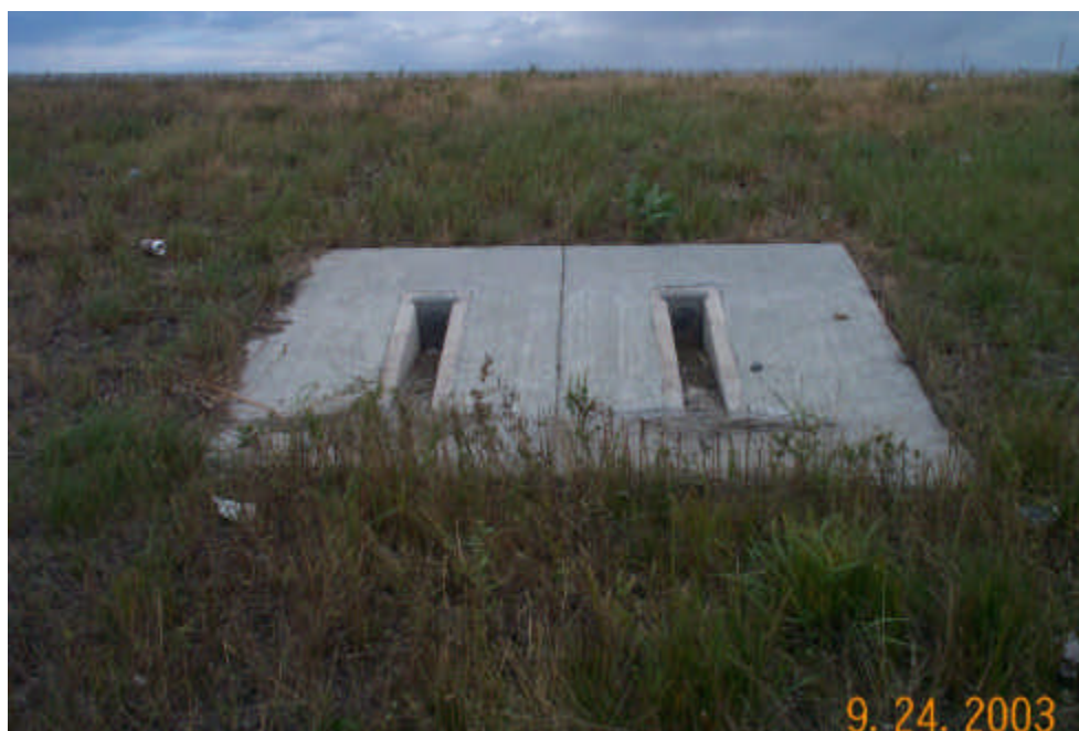
Photo 15 - Typical double concrete barrier.
