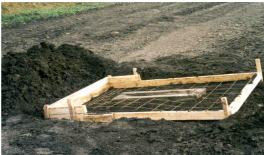
Photo 7 - Modified concrete barrier.
