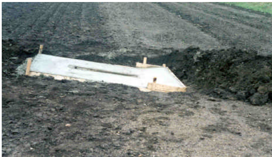
Photo 8 - Finished concrete barrier.
