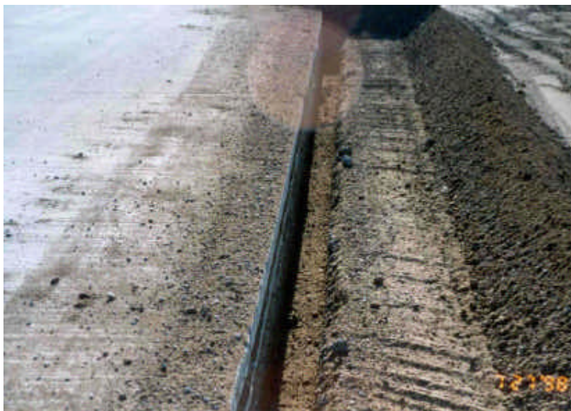
Photo 1 - Trench for edge drain.
