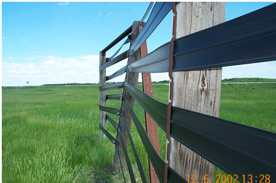
Photo 5 - A tilted fence post at Site 4.
