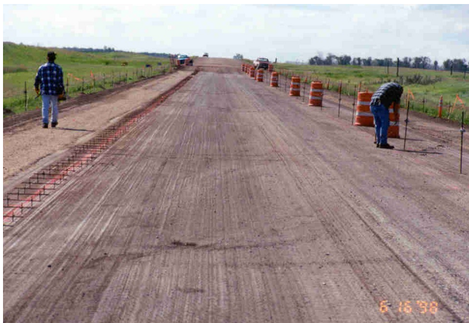
Photo 2 - HBP surface after milling was concluded.
