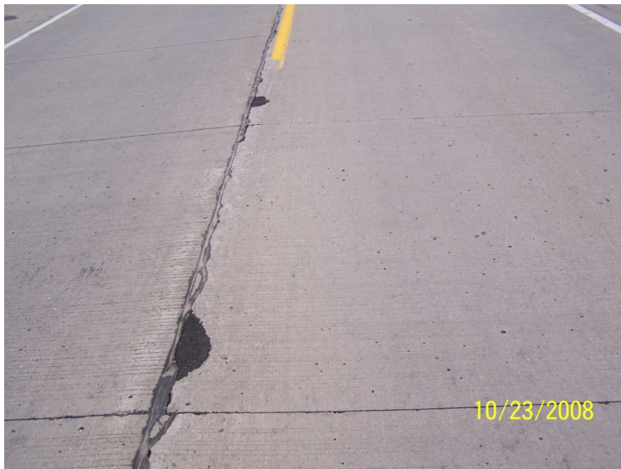
Photo 10 – Typical longitudinal and transverse joints.
