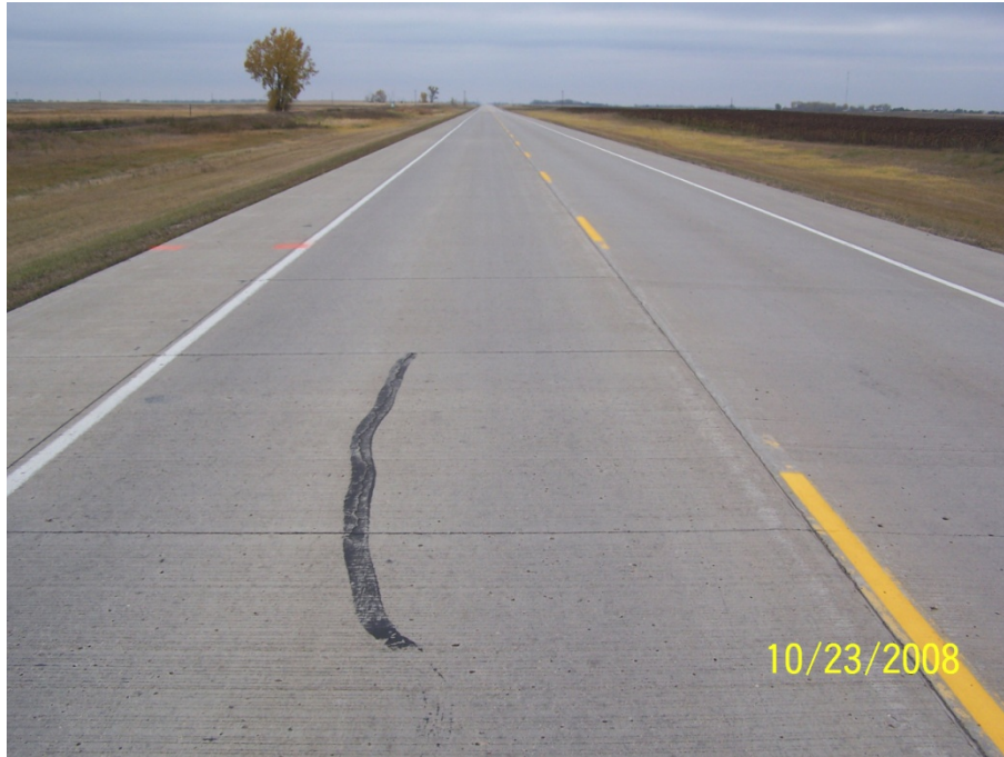
Photo 12 – Overview of Section 2, 6" PCC overlay
