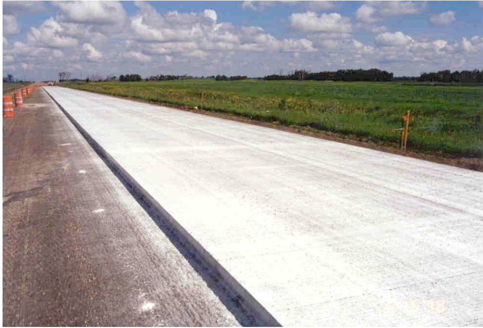
Photo 3 - Overview of finished slab in the northbound lane of section 1 (5" PCC).
