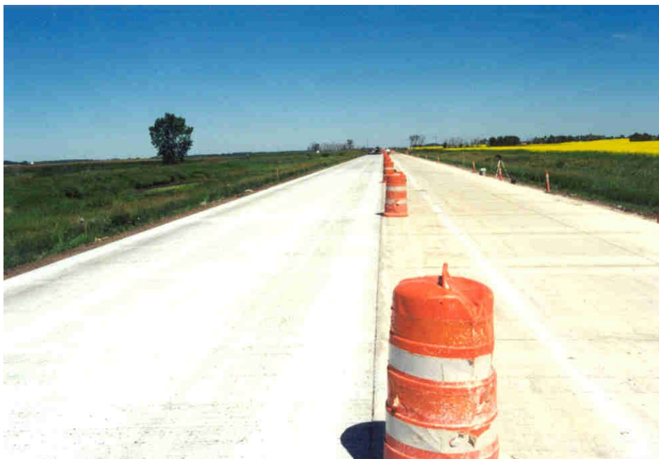
Photo 7 - Overall view of test section 1.
