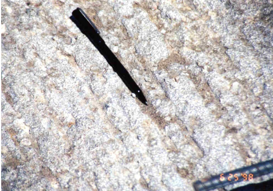
Photo 6 - Small particles found on the HBP prior to paving.
