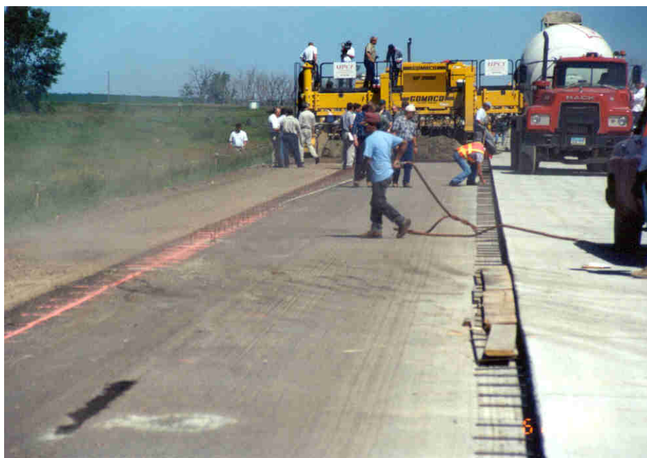
Photo 5 - Paving operation in southbound lane.
