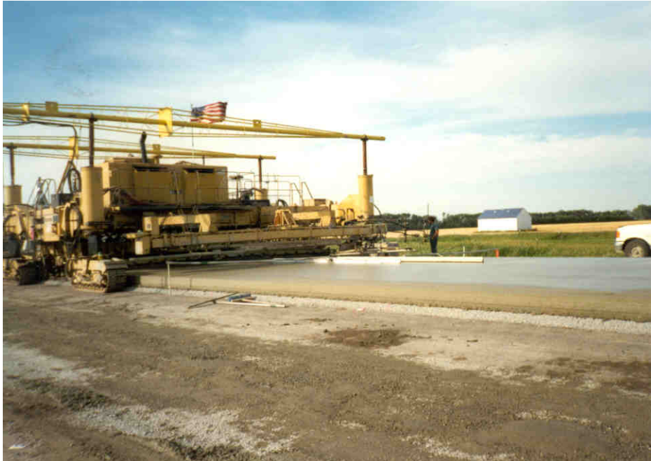
Photo 3 - Finished PCC pavement prior to carpet drag
