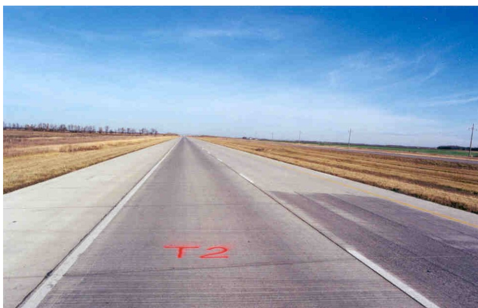
Photo 8 - Overall view of Test Section 2
