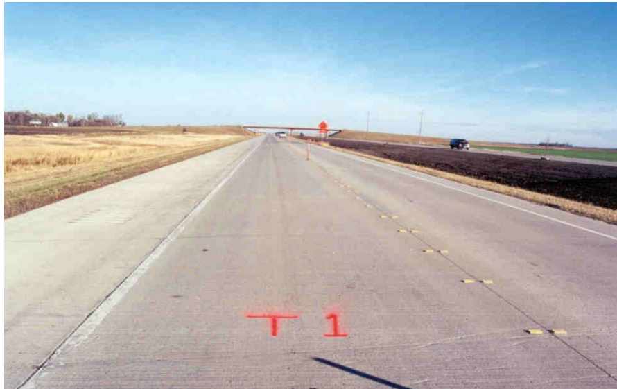
Photo 6 - Overall view of Test Section 1.
