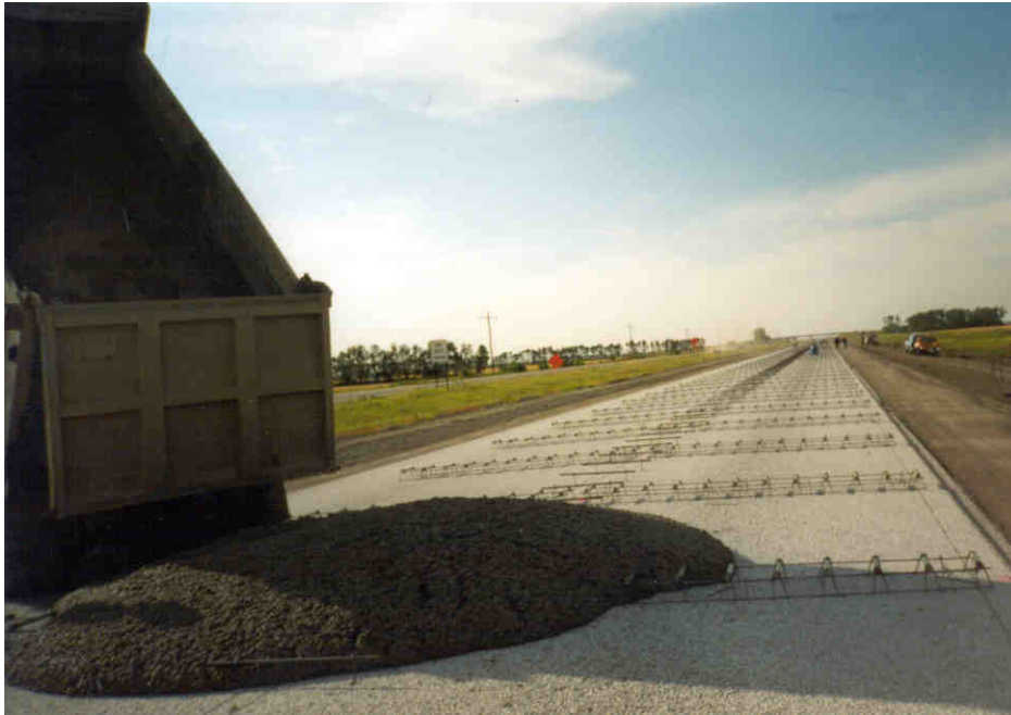
Photo 2 - Placing of the concrete
