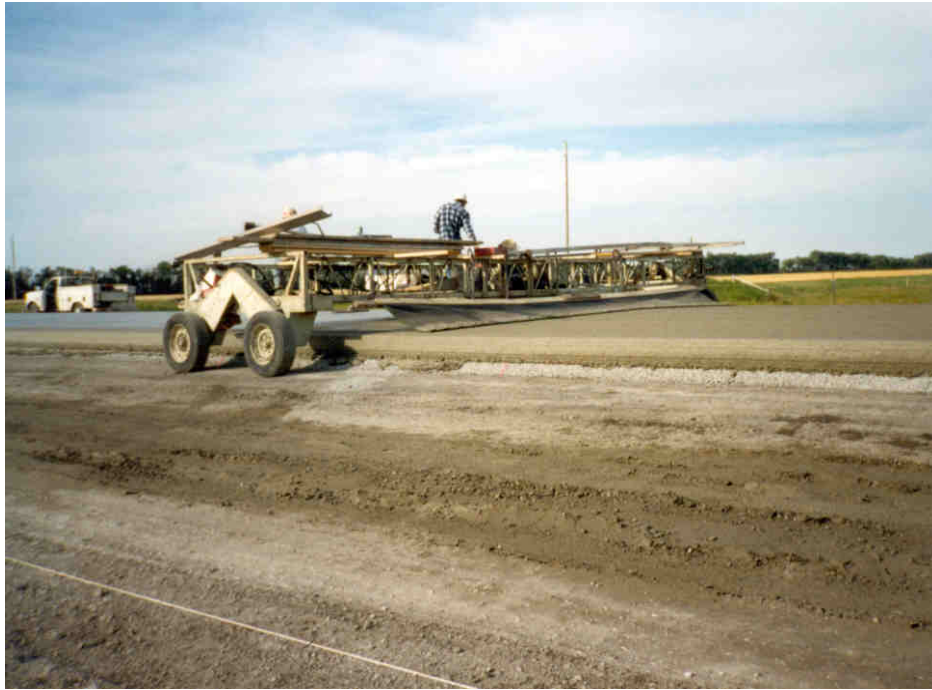
Photo 4 - Carpet dragging finished PCC pavement
