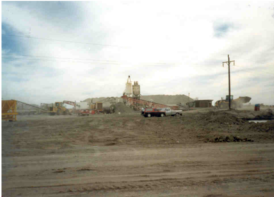
Photo 1 – Concrete plant site.
