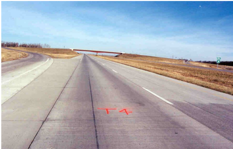
Photo 12 - Overall view of Test Section 4
