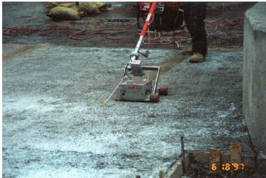
Photo 5. A view of the joints being sawed by the soft-cut procedure
