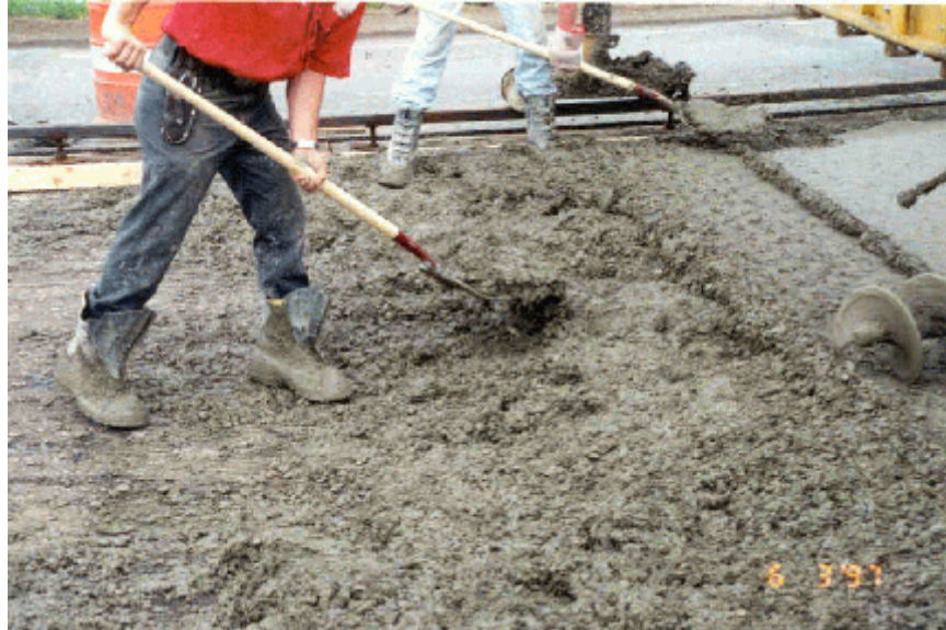
Photo 4. Shows the use of pitchforks to spread the fiber reinforced concrete.
