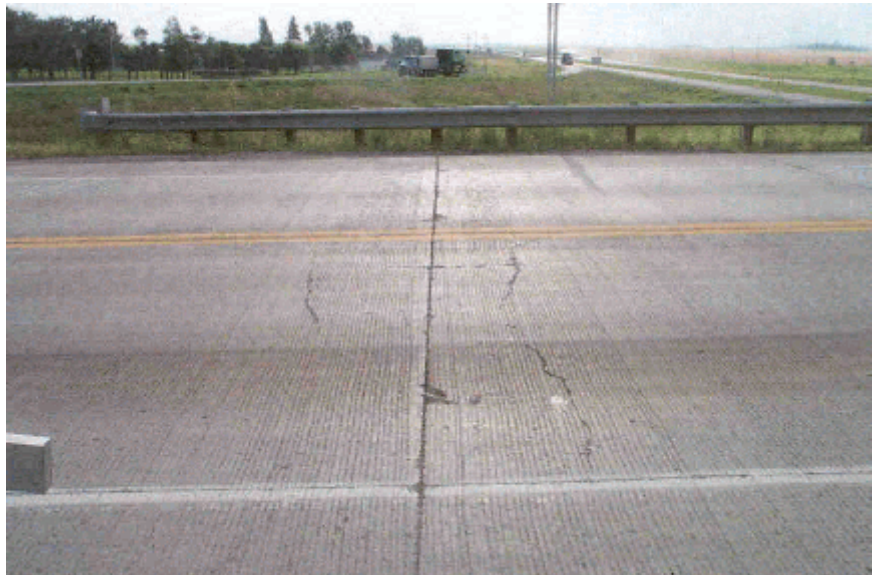
Photo 11. A view of the second joint in 2001.
