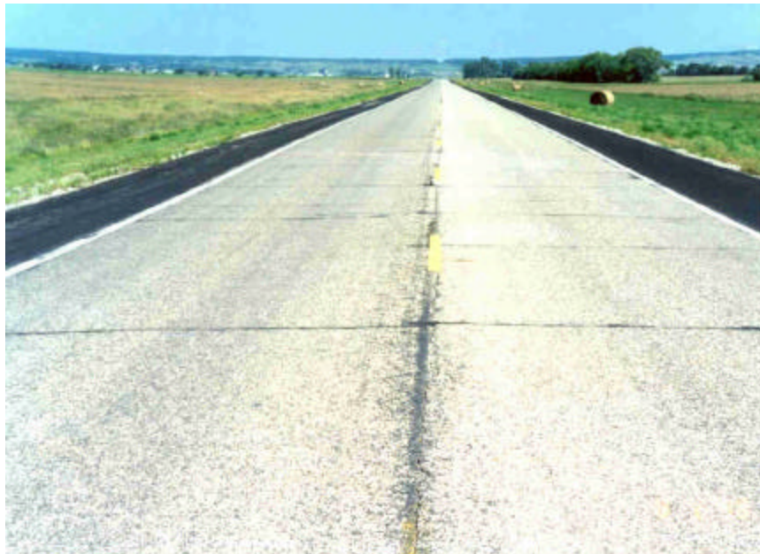
Photo 12 - Overview of section 5.
