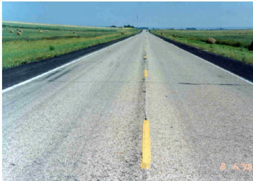
Photo 27 - Overview of section 10.
