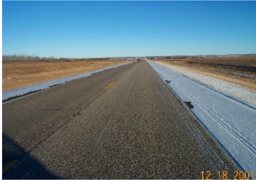
Photo 16 - Overview of section 6.
