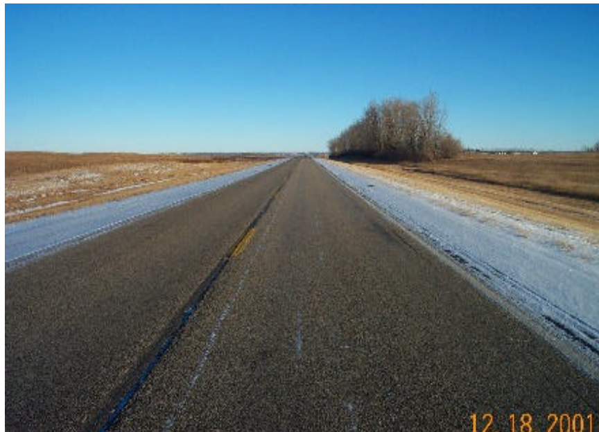
Photo 22 - Overview of section 7.
