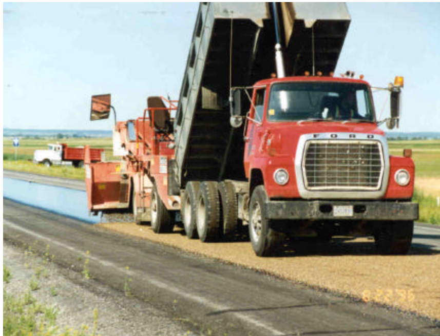
Photo 1 - Typical view of construction process.
