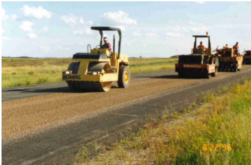
Photo 2 - Typical view of construction operation.
