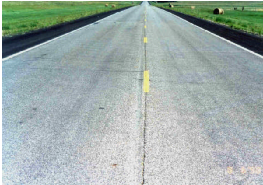
Photo 17 - Overview of section 7.
