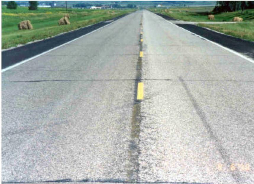
Photo 8 - Overview of section 3.
