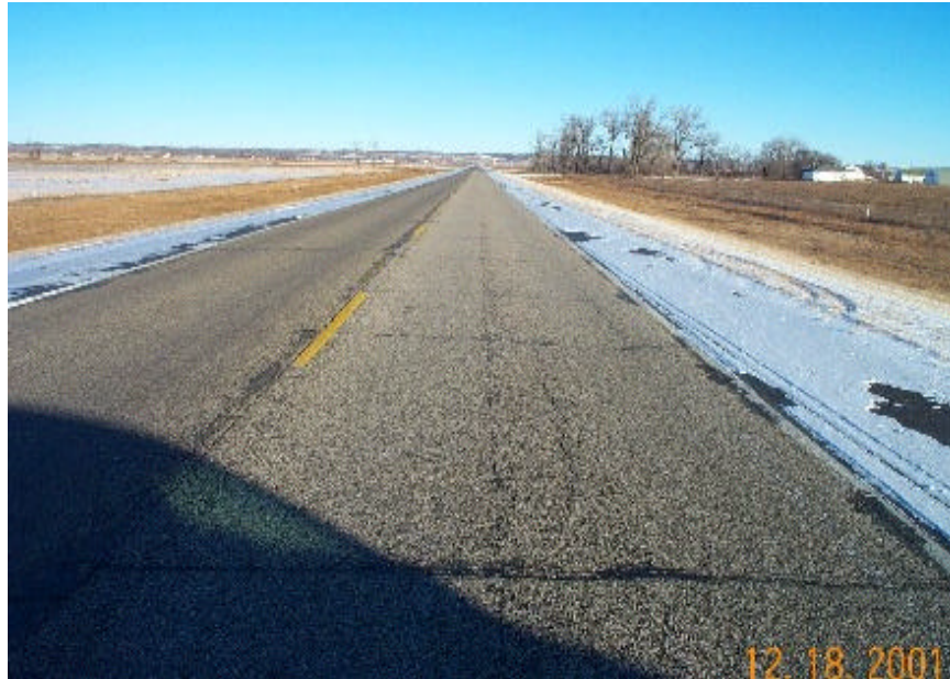
Photo 9 - Overview of section 3.
