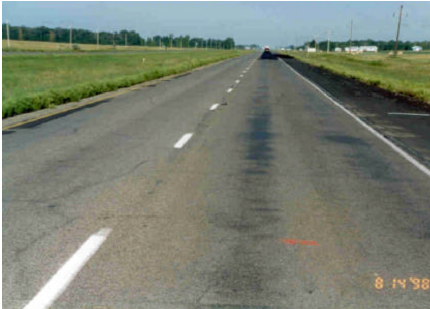
Photo 30 - Overview of Highway 2 where patching has been done.
