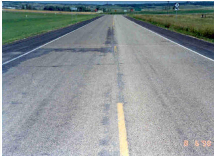
Photo 3 - Overview of section 1.
