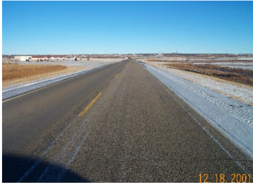
Photo 5 - Overview of section 1.
