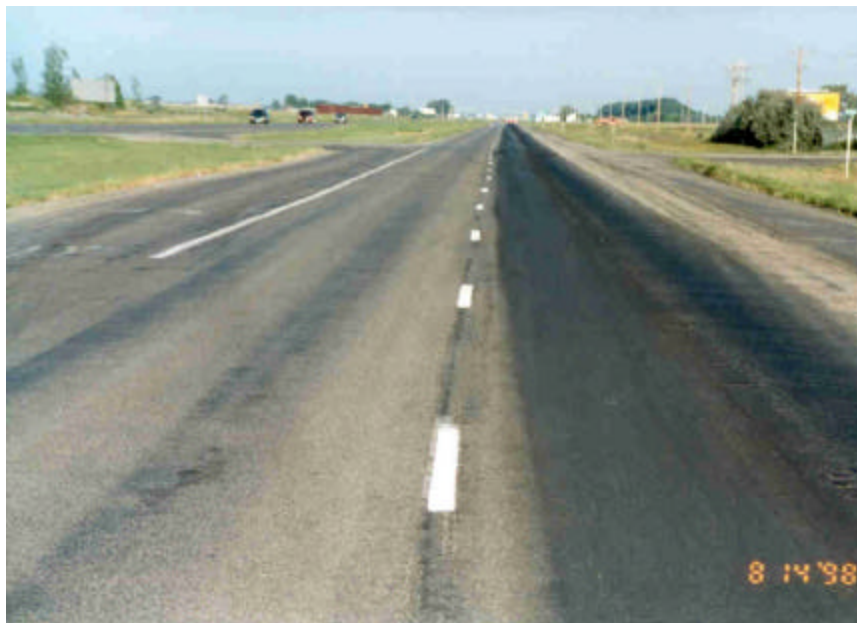
Photo 29 - Overview of Highway 2 test section.
