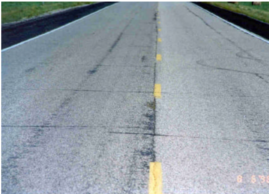
Photo 10 - Overview of section 4.
