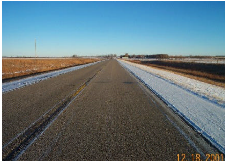
Photo 26 - Overview of section 9.
