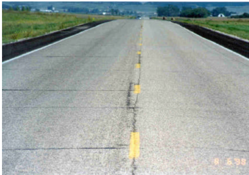
Photo 14 - Overview of section 6.
