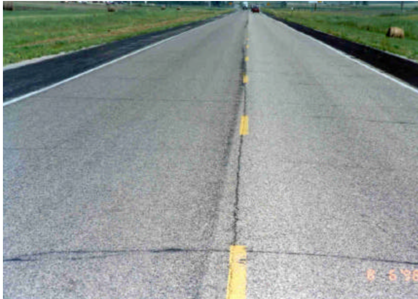
Photo 6 - Overview of section 2.
