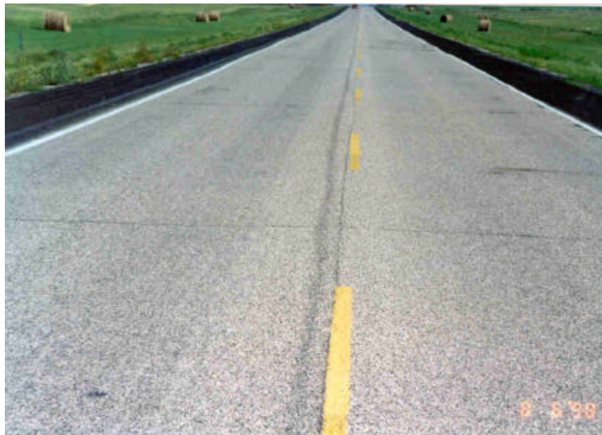
Photo 23 - Overview of section 8.
