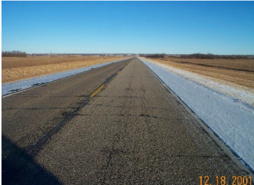
Photo 13 - Overview of Section 5.
