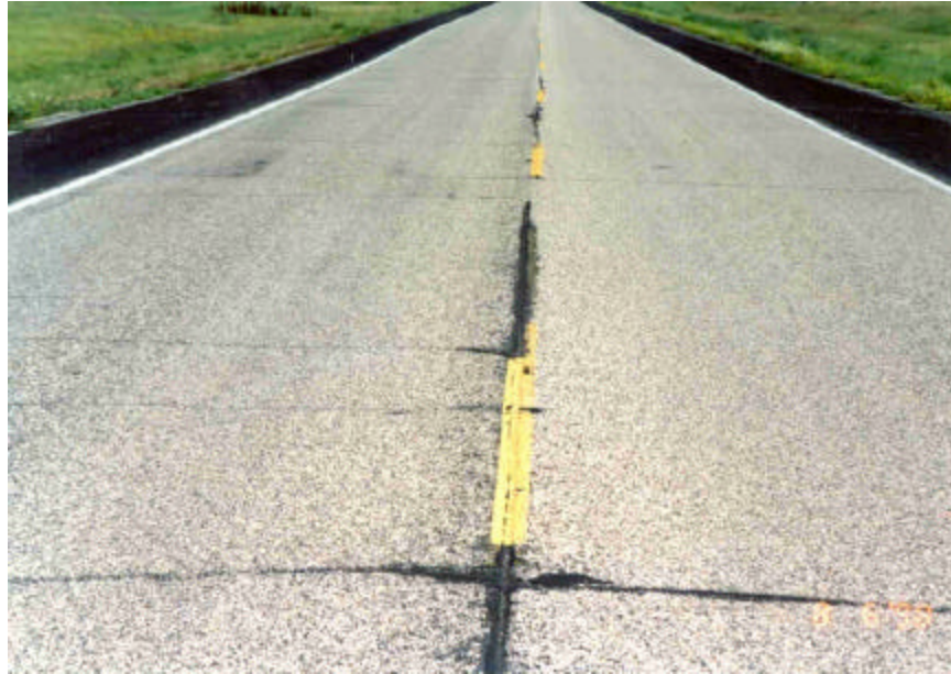
Photo 25 - Overview of section 9.
