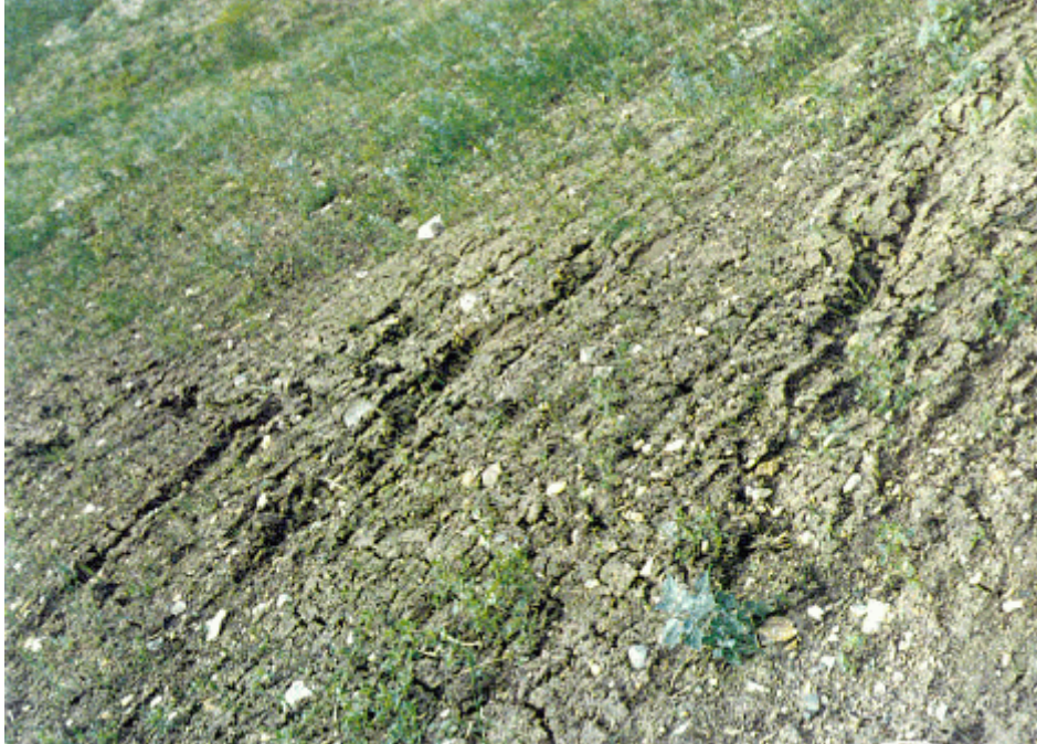
Photo - 15 Is a view of the slope where no slope protection was placed.
