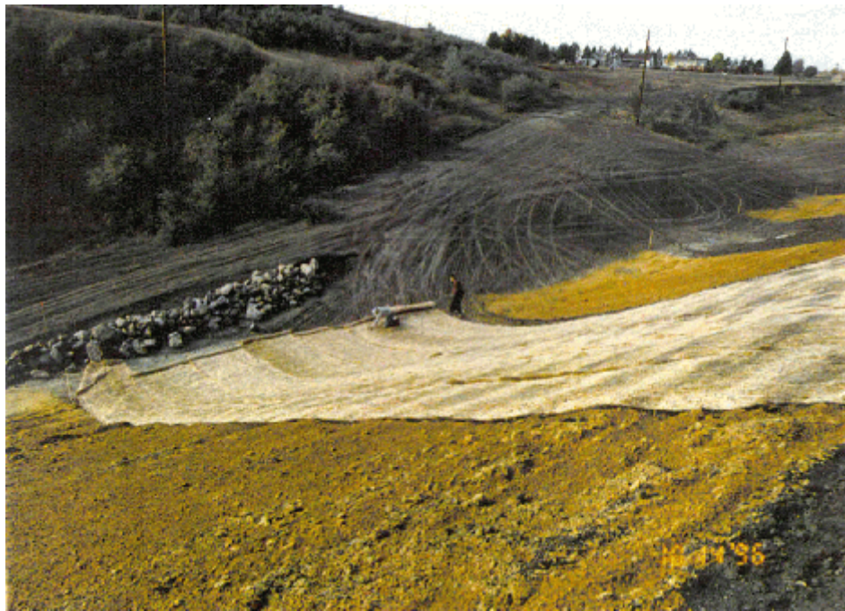
Photo - 8 Straw mat installation.
