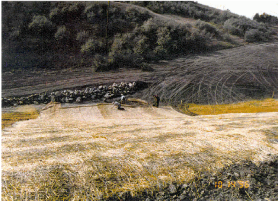
Photo 9 - View of nearly finished slope.
