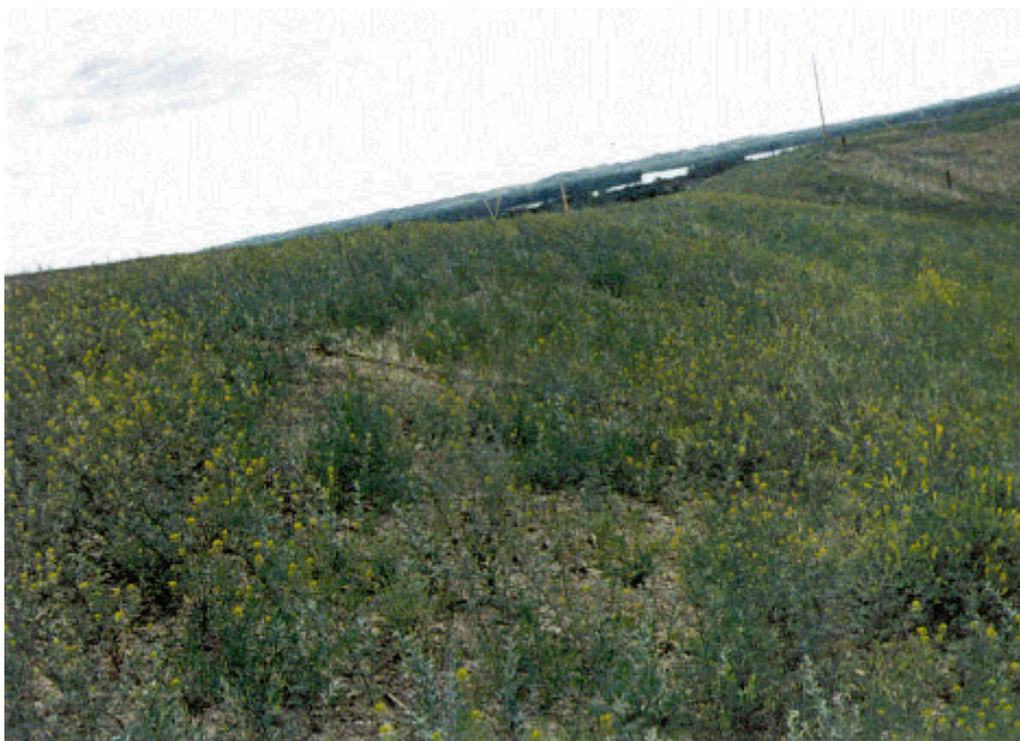
Photo - 20 A view from the side of the slope with the Soil Guard® on the left and the Double Netted Straw on the right or top of the picture.
