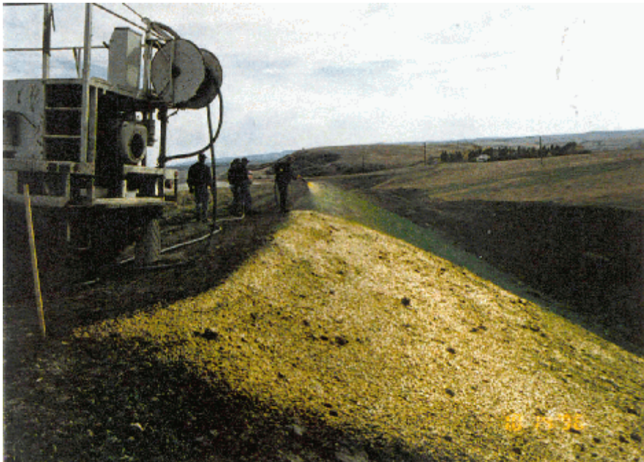
Photo 3 - Hydraulically applying the Soil Guard® Bonded Fiber Matrix.
