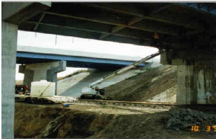
Photo 5: View of worker performing high pressure wash.
