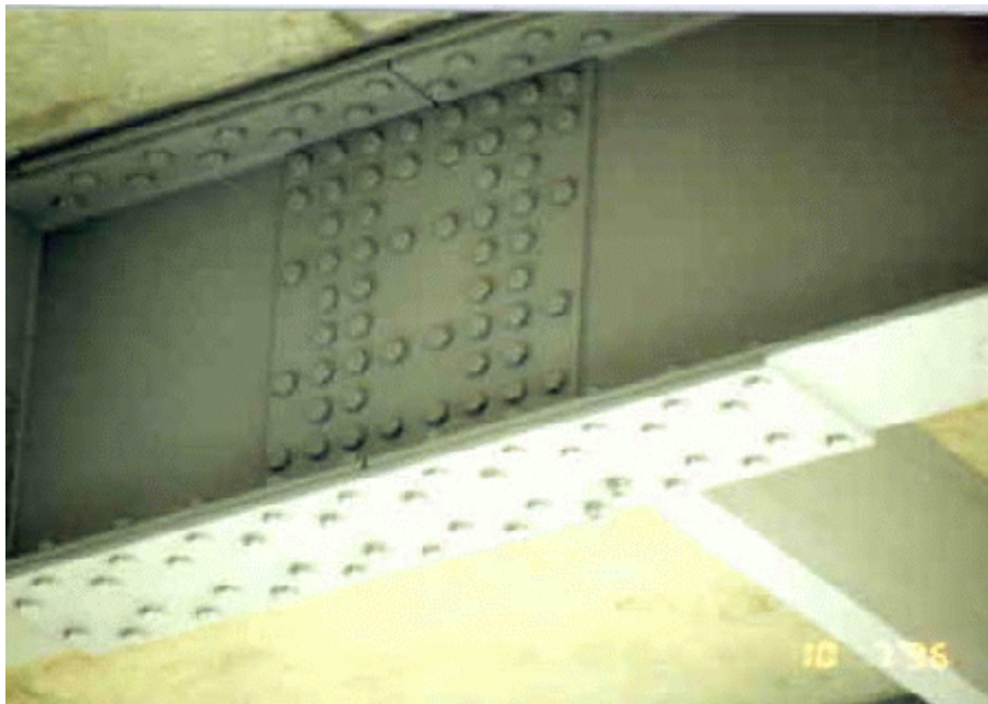
Photo 10: Close up view of beam splice with prime coat applied.
