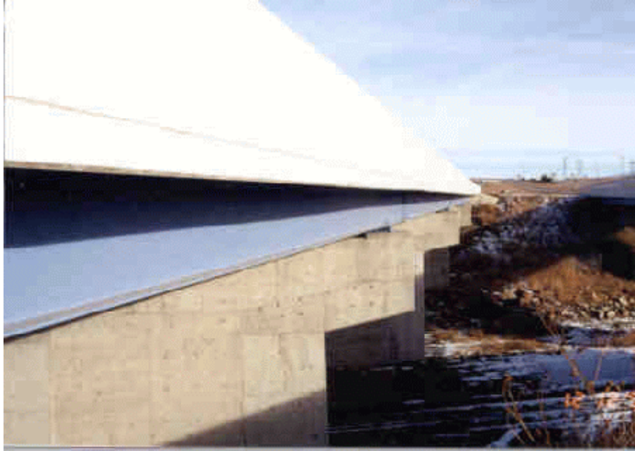
Photo 13: View of south side of westbound structure.
