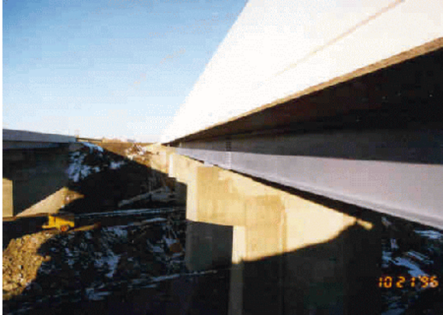
Photo 9: View of exterior beam with prime coat applied.
