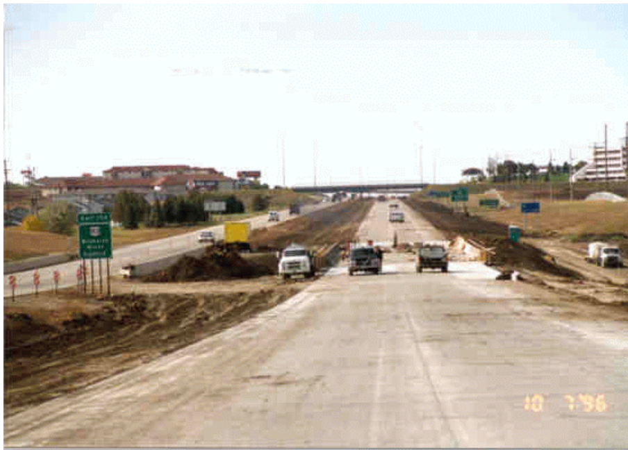
Photo 1: View of the site looking west.
