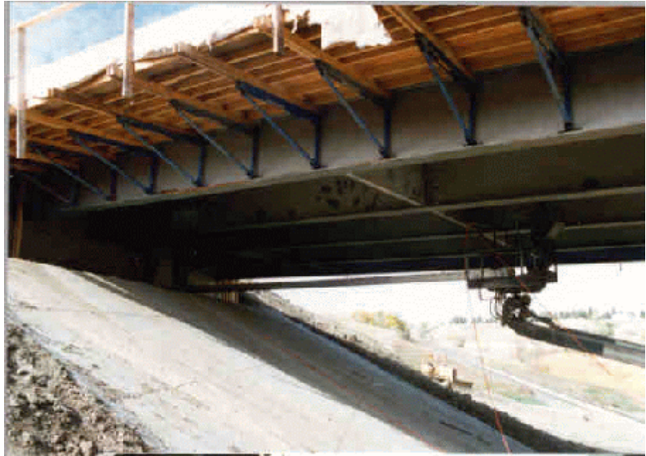
Photo 2: View of first span to be high pressure washed.
