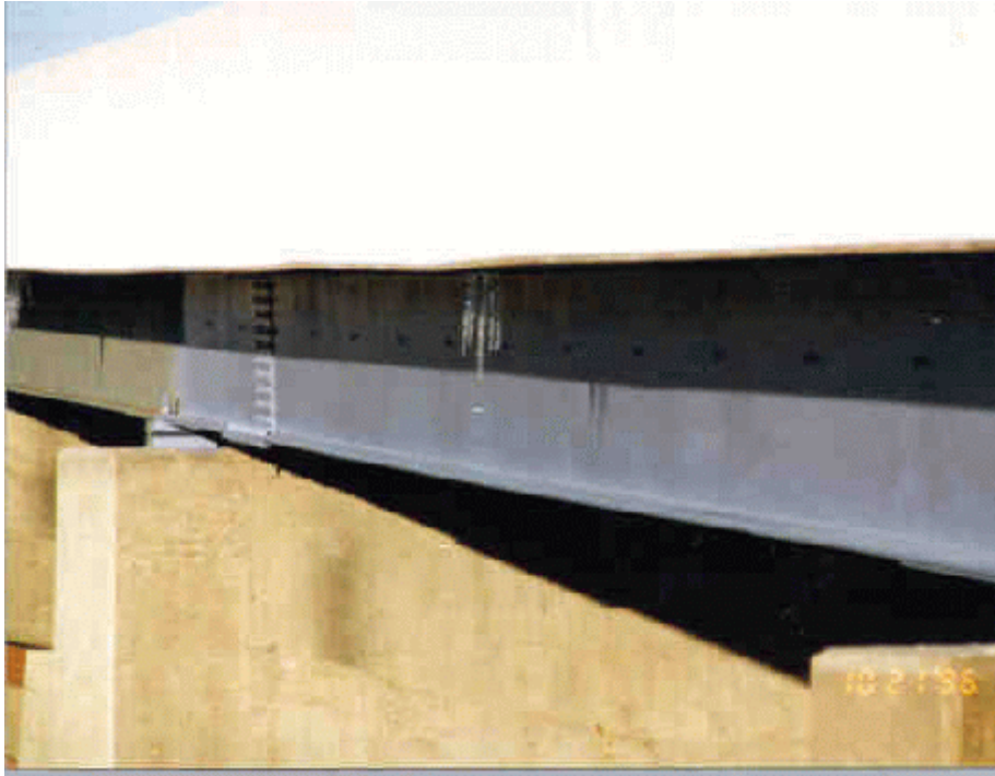
Photo 11: View of exterior beam with prime coat applied during cold weather.
