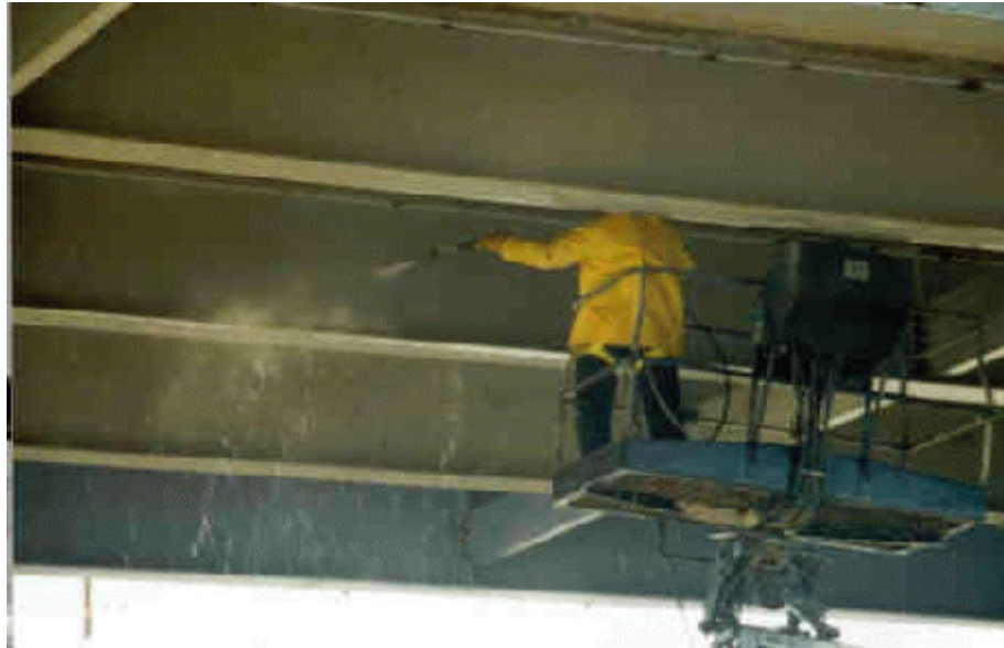
Photo 4: Worker performing high pressure washing.
