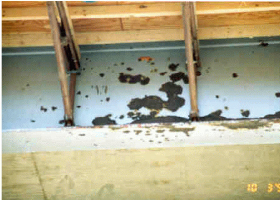
Photo 6: View of exterior beam after high pressure wash.
