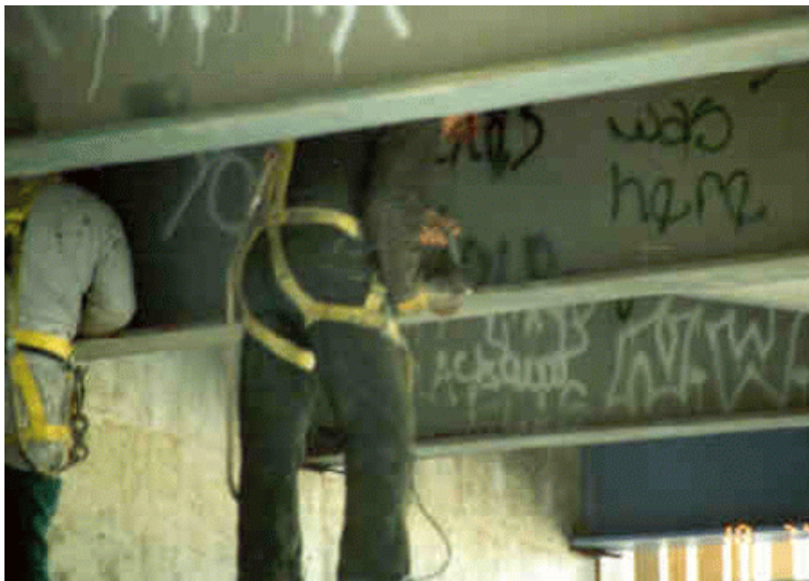
Photo 7: View of worker spot grinding.
