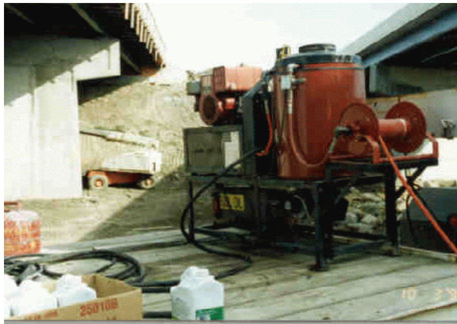
Photo 3: View of trailer mounted high pressure washer.
