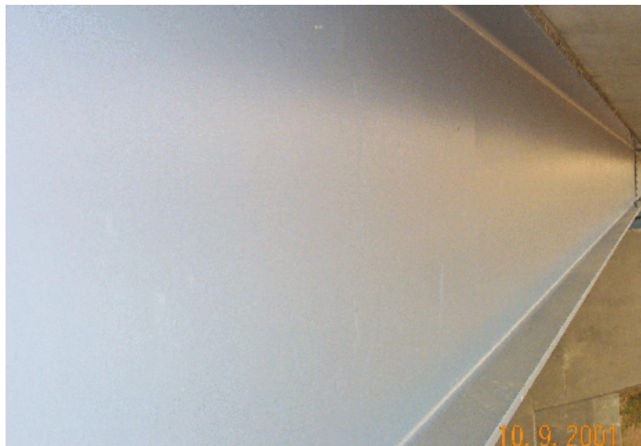
Photo 20: View of south beam on eastbound structure.
