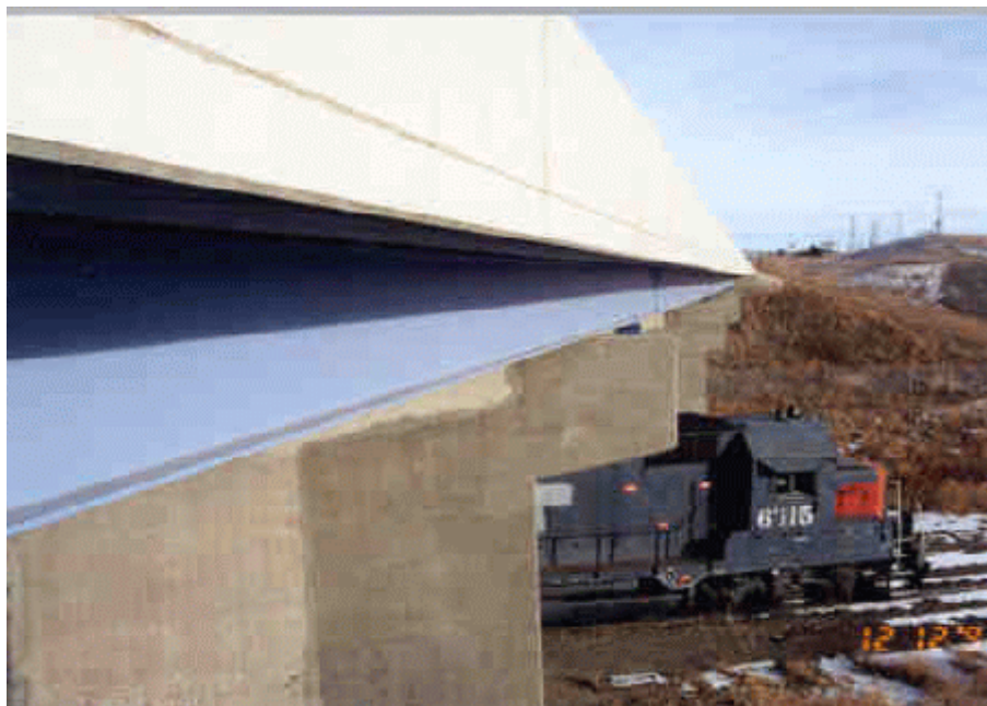
Photo 14: View of south side of eastbound structure.
