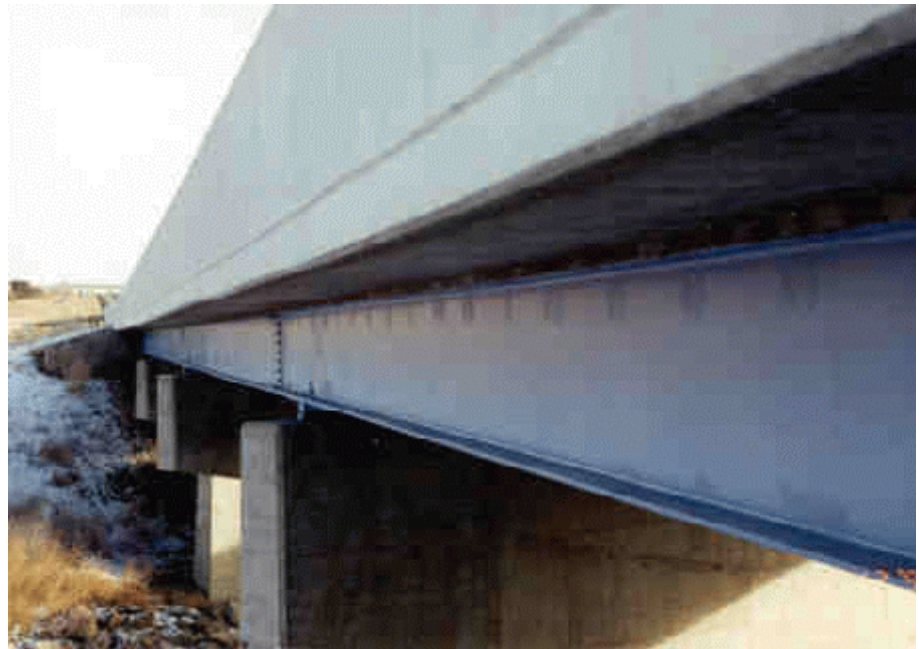
Photo 15: View of north beam on westbound structure.
