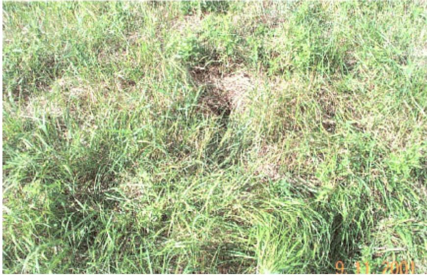
Photo 3. Grass covering headwall (Sta. 2073+00L).
