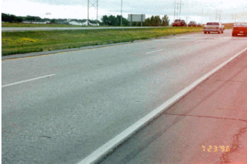
Photo 6. View of the northbound test section between 12th Avenue North and 19th Avenue North.
