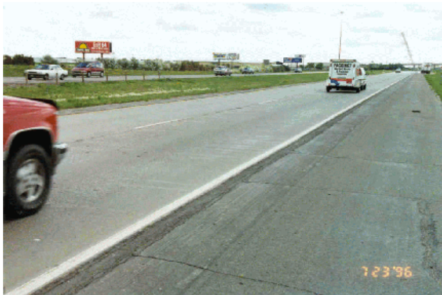
Photo 11. A typical section in the southbound lane of I-94.
