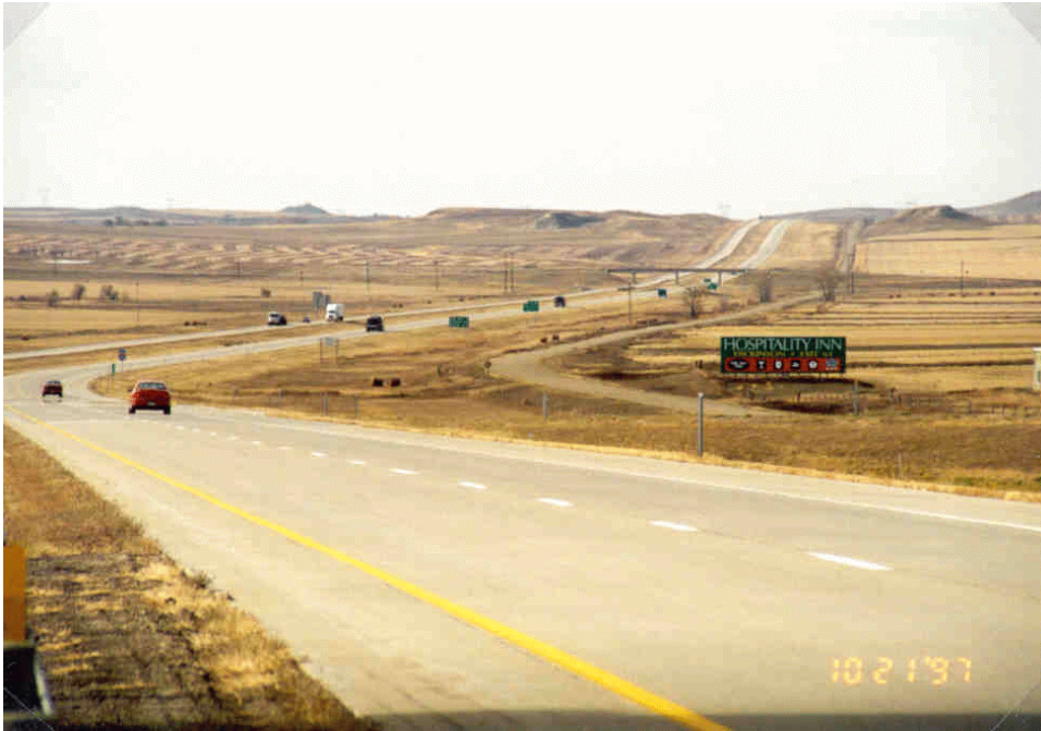
Photo 1. Overview of the tining project
