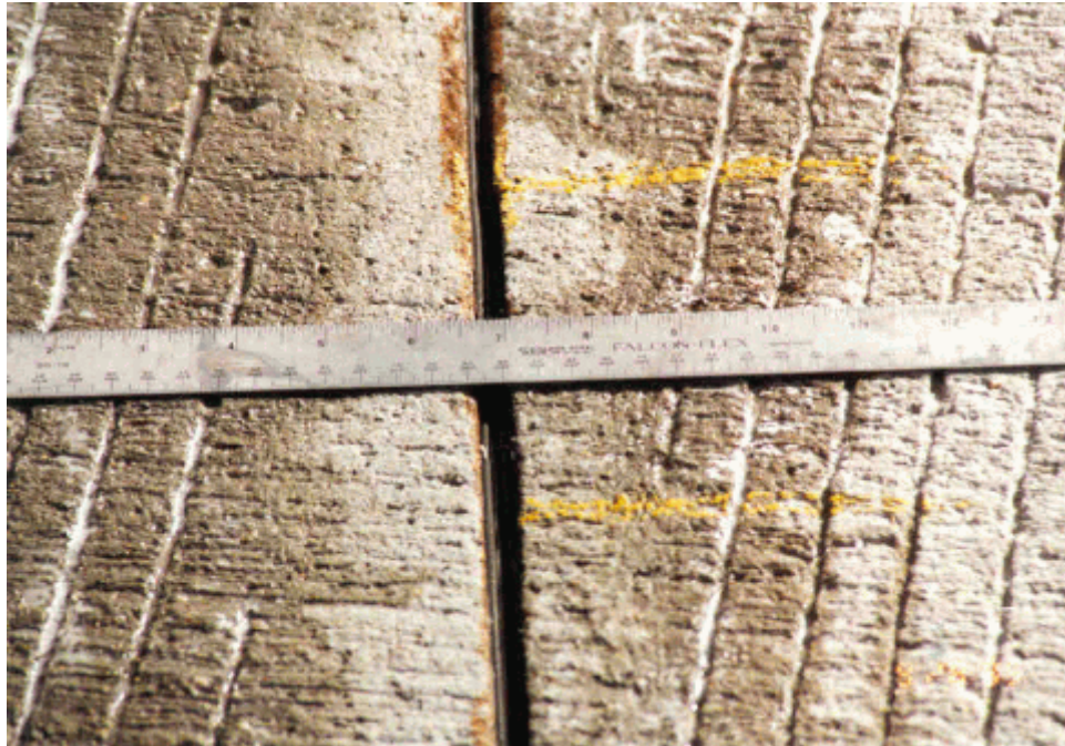
Photo 11. View of sealant in an irregular sawed joint
