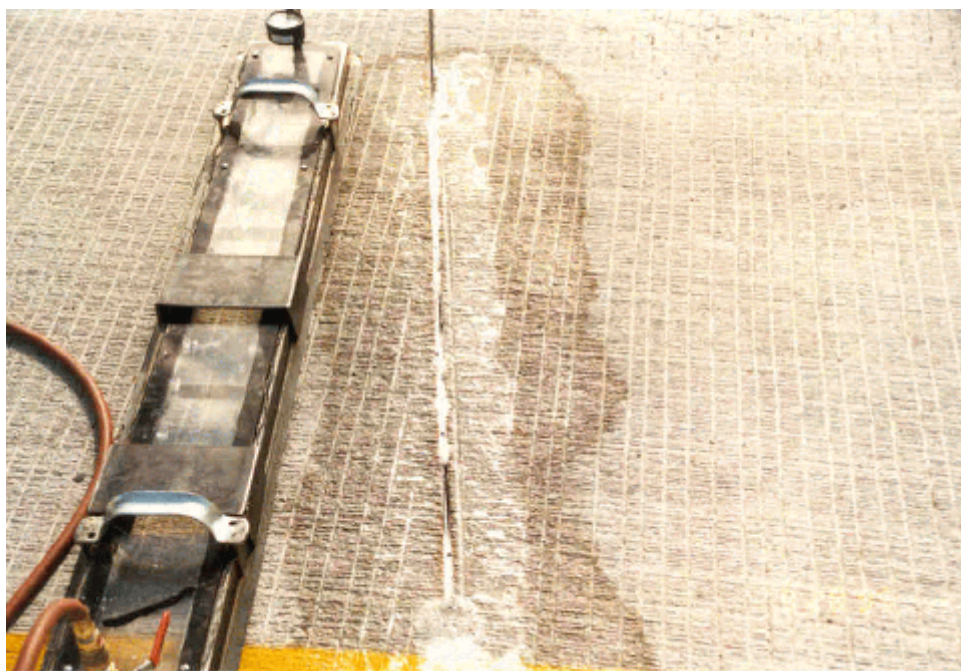
Photo 10. Close-up of Station 1094+95
