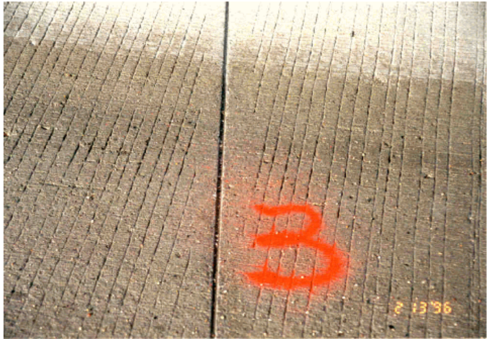
Photo 17. Typical joint where silicone sealant is applied
