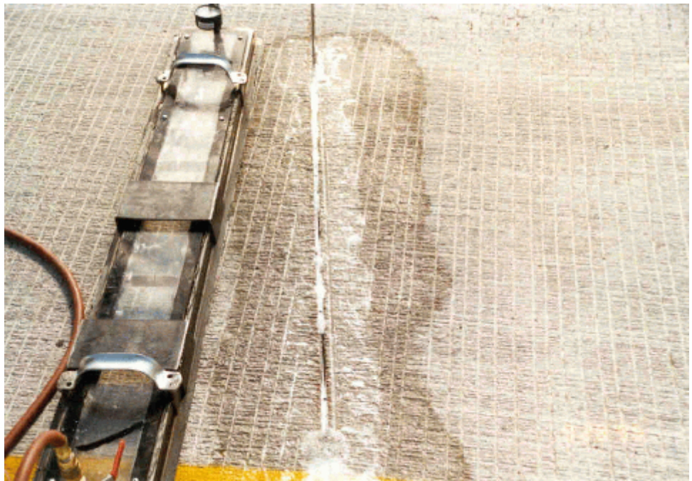
Photo 2. Joint sprayed with soapy solution
