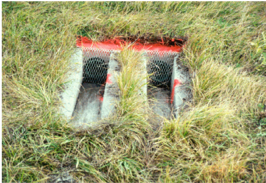
Photo 2: Typical Headwall-Painted for Ease of Location and Identification of Damage
